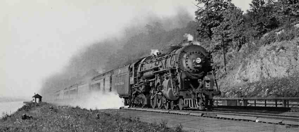
New York Central J-1 Hudson 5328 leads the North Shore Limited through Tivoli, New York, in September 1949. The locomotive is taking water from a track pan located between the rails. New York Central was one of a few lines that used track pans to speed up operations. On most lines, steam locomotives had to stop at regular intervals to fill the tender. William D. Middleton
