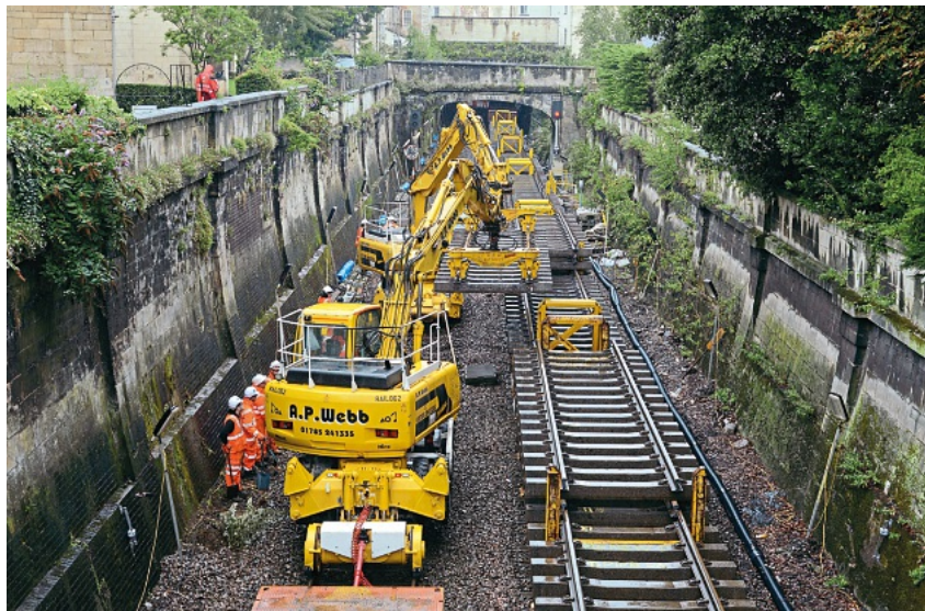
Sydney Gardens in Bath is a mass of yellow on August 24 as work to lower the track by 200mm enters its final stages through this famous World Heritage Site. NETWORK RAIL
