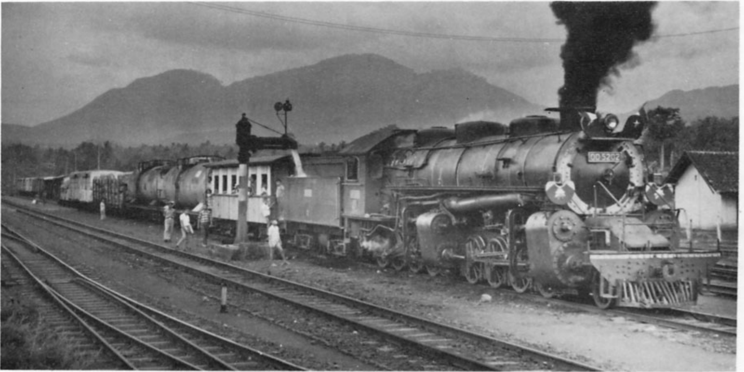
PNKA's massive 2-8-8-0 No DD5202, one of the world's last few eight-coupled Mallets, seen at Tjitjalengka, Java, in October 1970, heading a mixed in stormy weather
