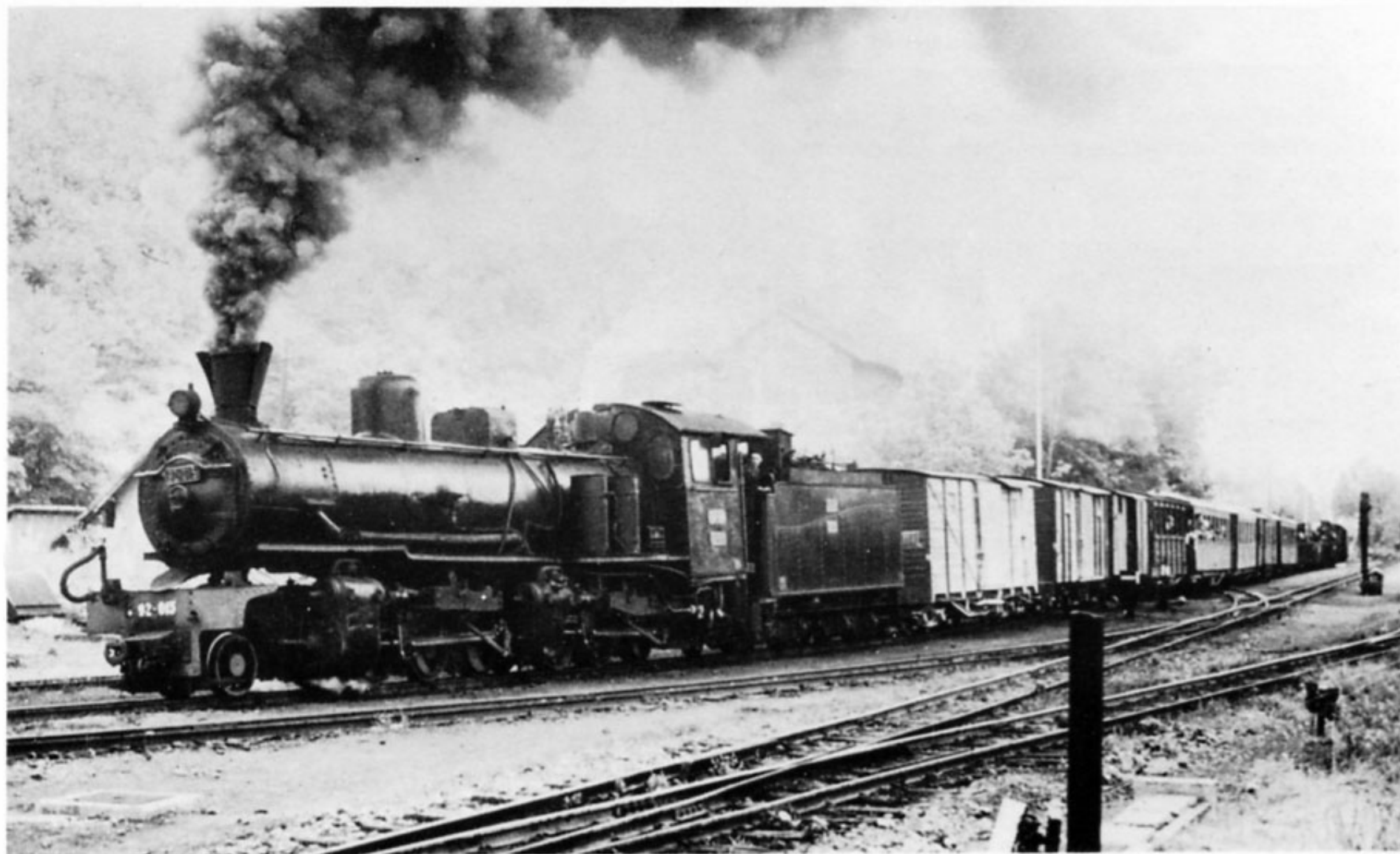
Two Yugoslavian 760mm gauge 2-6-6-0s, one fore and one aft, lift a mixed train out of Metovnica, in Eastern Serbia
