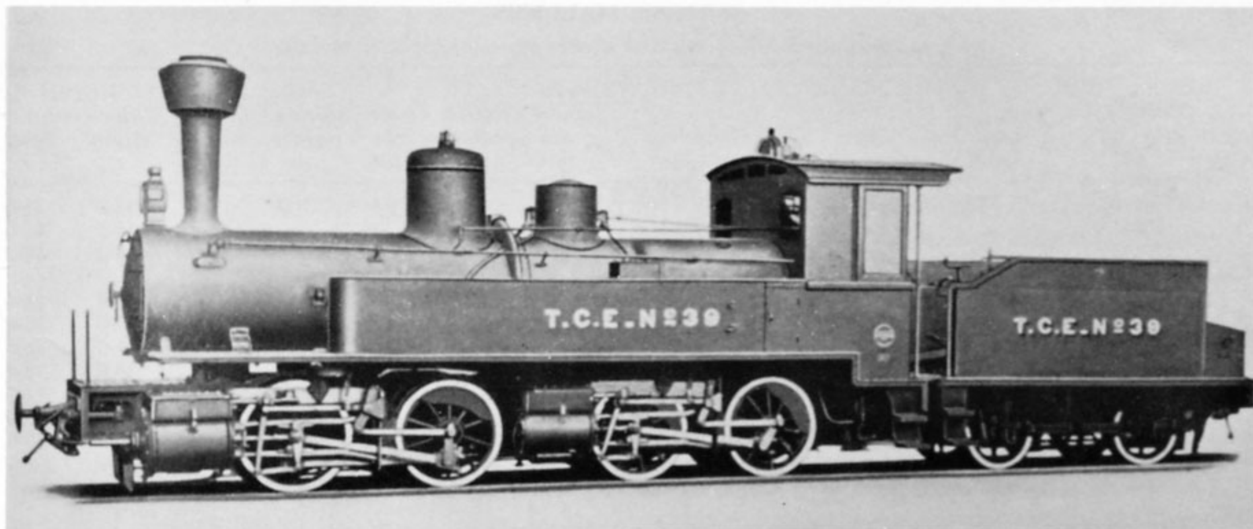
Madagascar's unique island evolution in Mallet types was the 0-4-4-0 tank + tender compound. One of Baldwin's batch is shown here
