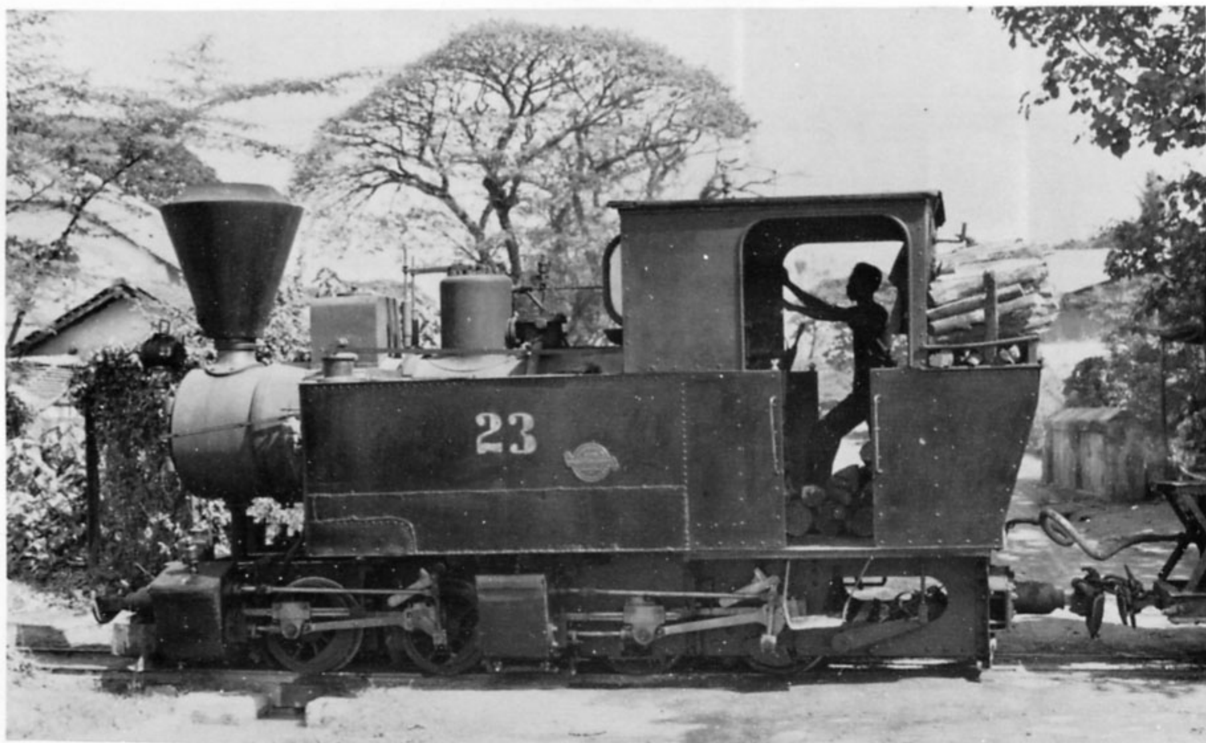
Not the first Mallet, but differing little in size or detail, a narrow-gauge 0-4-4-0T compound at Redjo Agung Sugar Mill in Java, Indonesia
