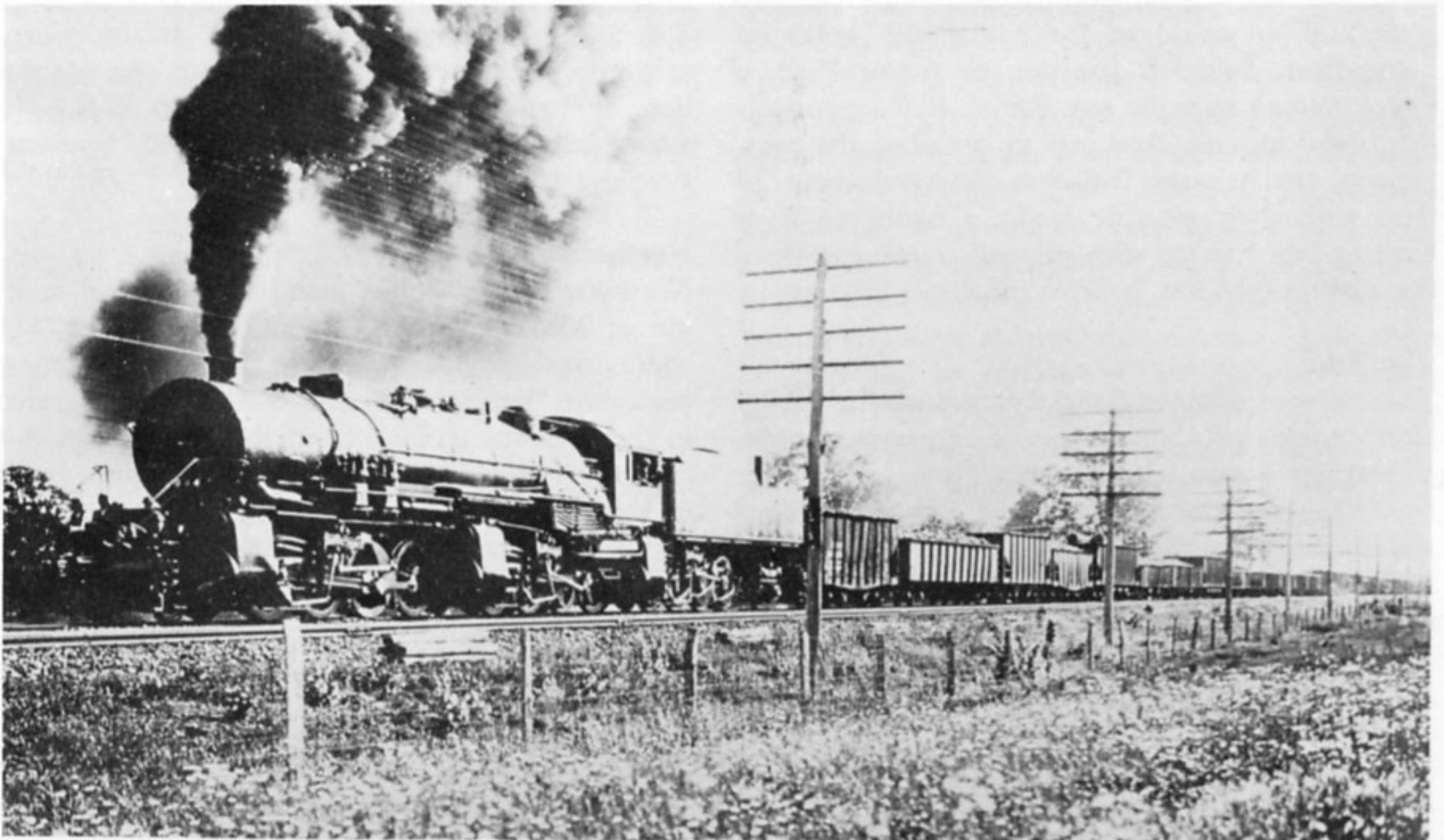
A rare old print of an Erie Triplex in action, probably No 5014 on its trial run with 250 cars of coal
