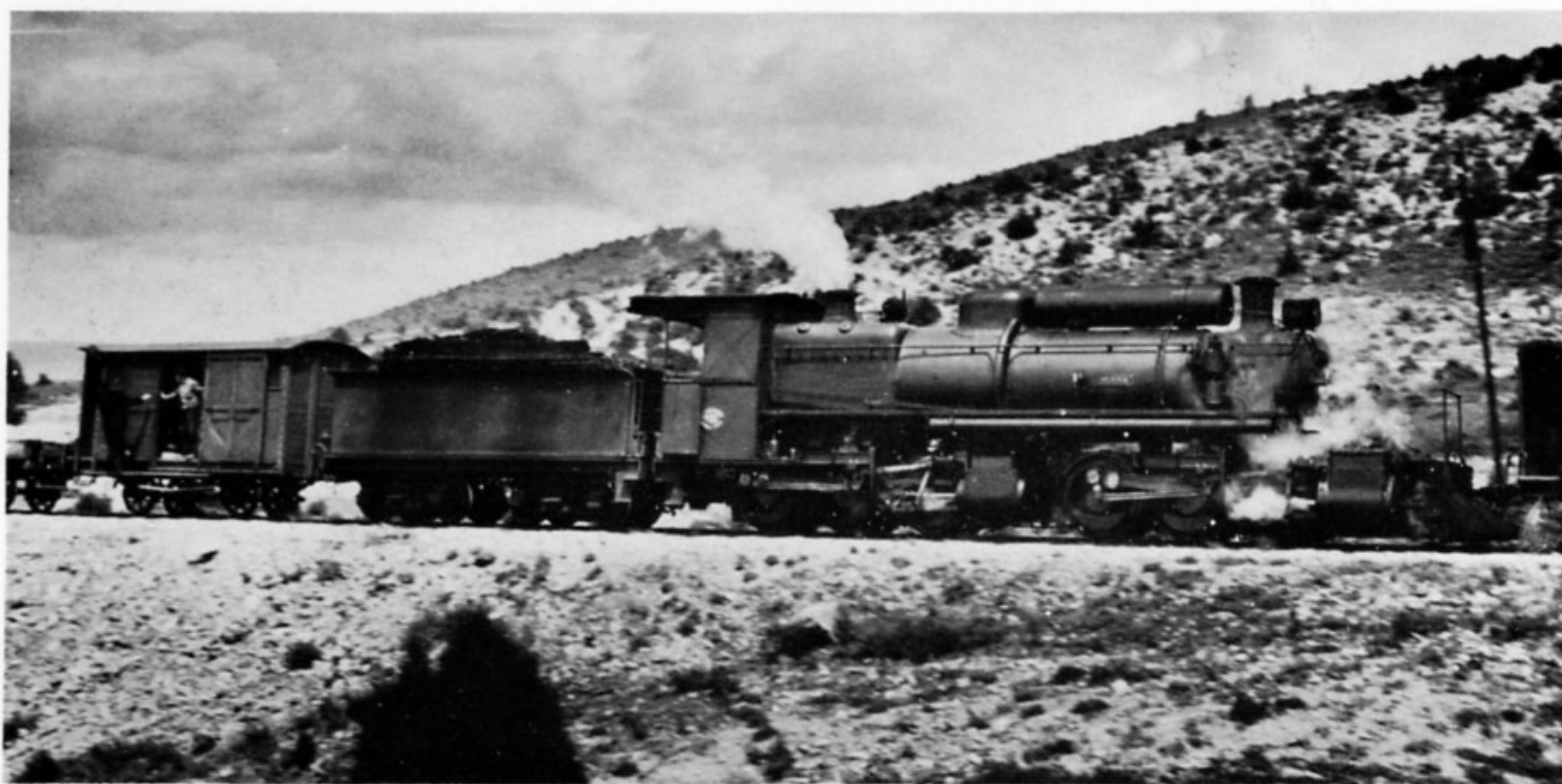
Sierra Menera's North British 0-6-6-0 No 401 climbs up from Teruel to Puerto de Escandon in 1962, assisting a Garratt-hauled ore train
