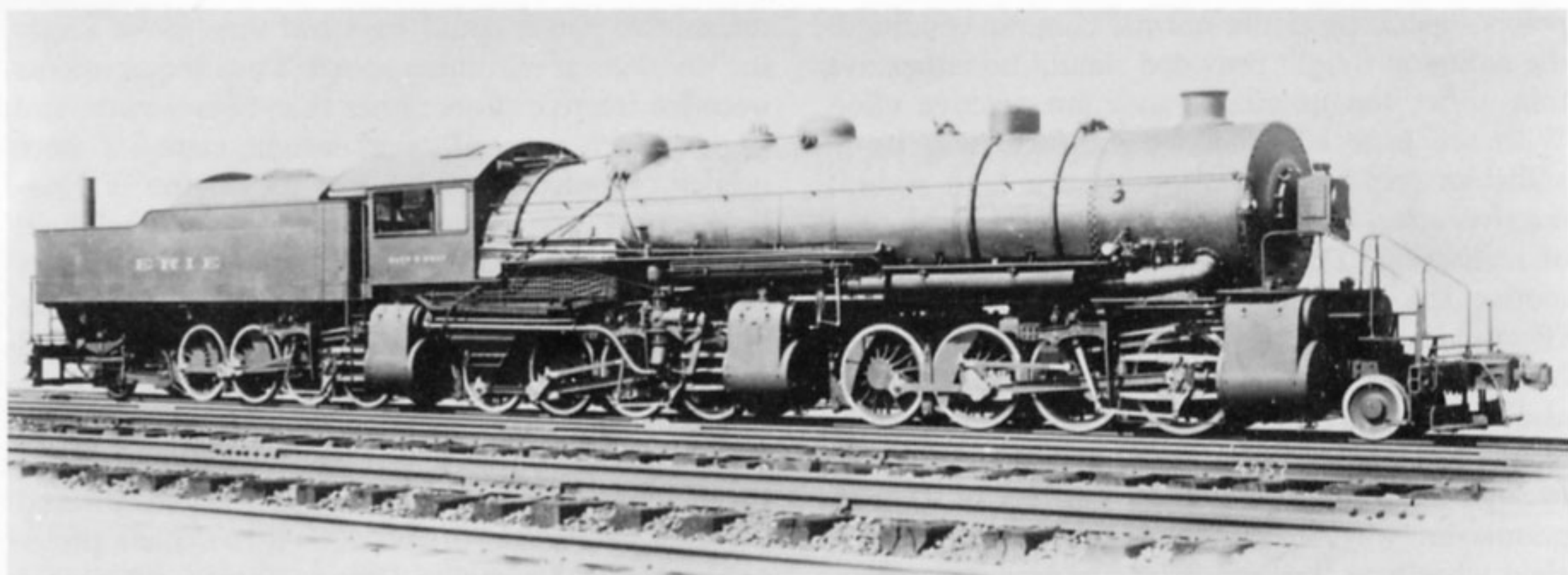
Henderson's original Triplex, a 2-8-8-8-2 built for the Erie Railroad in 1916, was an unsuccessful attempt to use the Mallet's tender weight to increase adhesion and tractive effort
