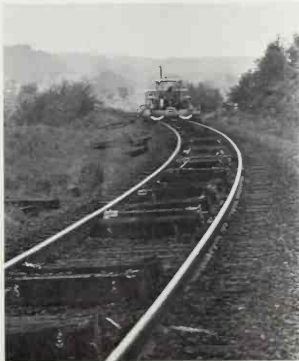
Sawing old ties for removal
