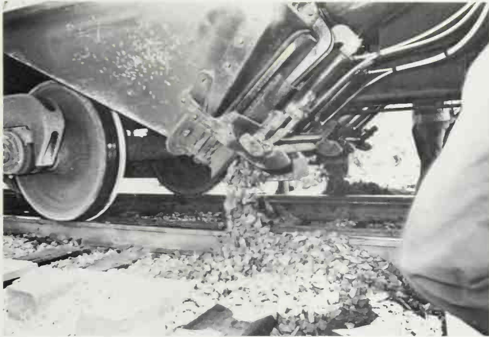
The rocks between the railroad ties are dropped from a hopper.
