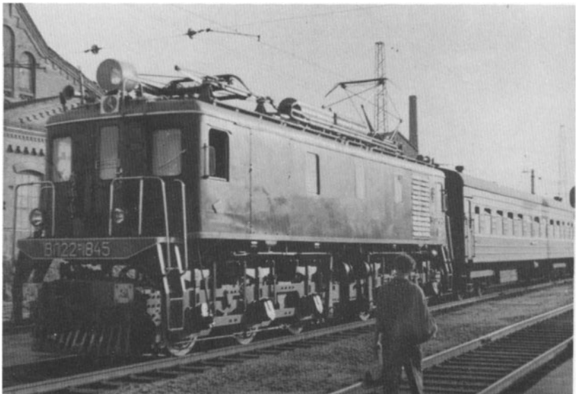
26. The VL22m type electric locomotive, a further development of the General Electric design.
