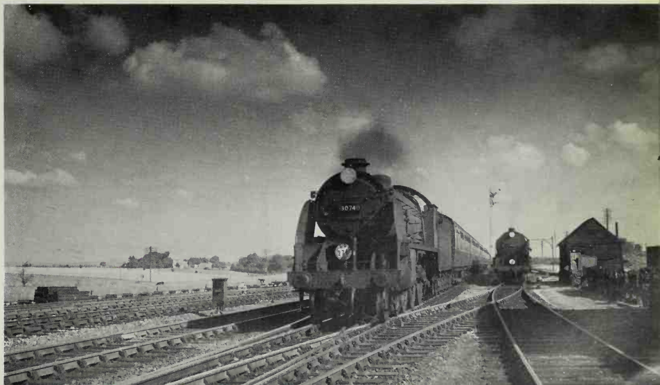
Urie 'N15' 4-6-0 No. 30740 Merlin tops the summit of the climb up from Andover Junction as it roars through Grateley on 29 September 1951. At the time the engine was allocated to Bournemouth (71B) shed and was a stranger on the line to Salisbury. The electric headlamps serve as a reminder that this engine was one of those modified in the abortive post-war oil-fired conversion programme on the SR. [Brian A. Butt]
