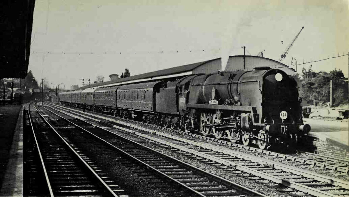
Urie 'N15' 4-6-0 No. 30740 Merlin tops the summit of the climb up from Andover Junction as it roars through Grateley on 29 September 1951. At the time the engine was allocated to Bournemouth (71B) shed and was a stranger on the line to Salisbury. The electric headlamps serve as a reminder that this engine was one of those modified in the abortive post-war oil-fired conversion programme on the SR. [Brian A. Butt]
