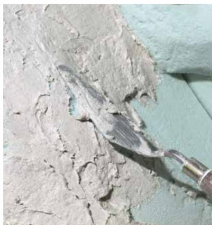
The blend of paper paste and plaster is applied with a spatula.
