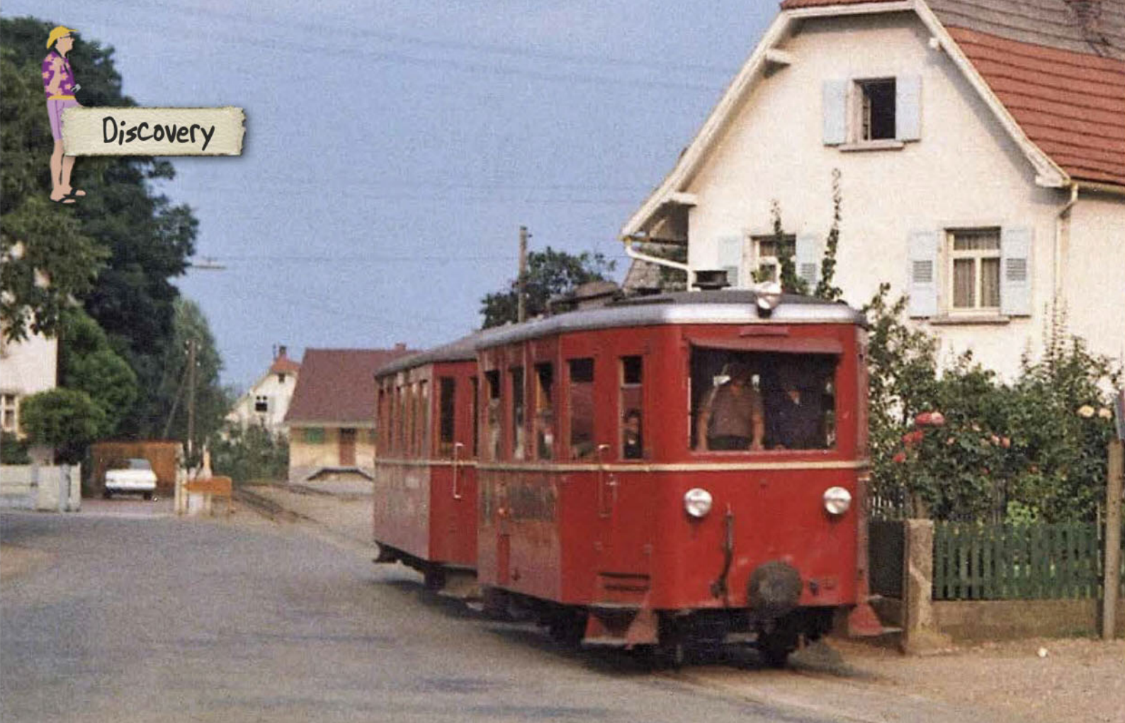
A Kehl-bound train arriving in Leutesheim (km 8.5). Four-wheeler railcar and trailer N° 8, ex-bogie railcar N° T 11 demotorized, built by Orenstein & Koppel 1936. (14 August 1965, J.-L. Rochaix)
