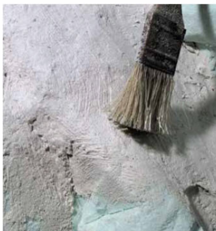
The ground is textured by stippling it with a dry paintbrush.
