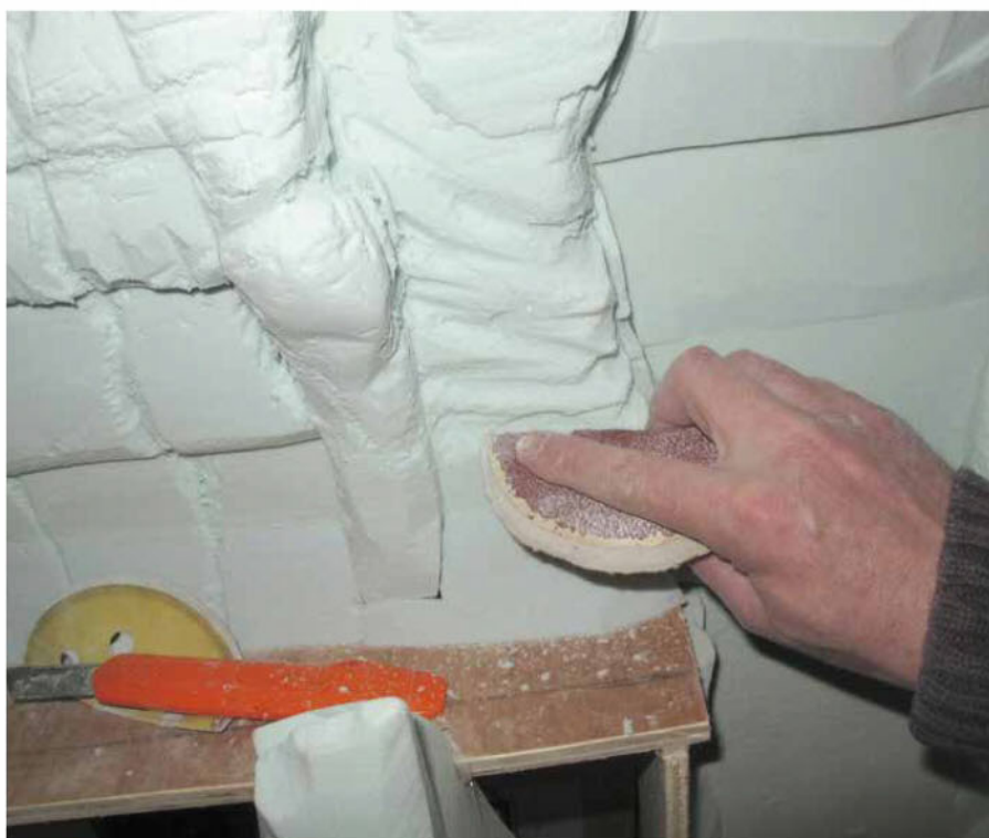
The cracks are opened up with sandpaper, I use the same tool to shape the curved parts.
