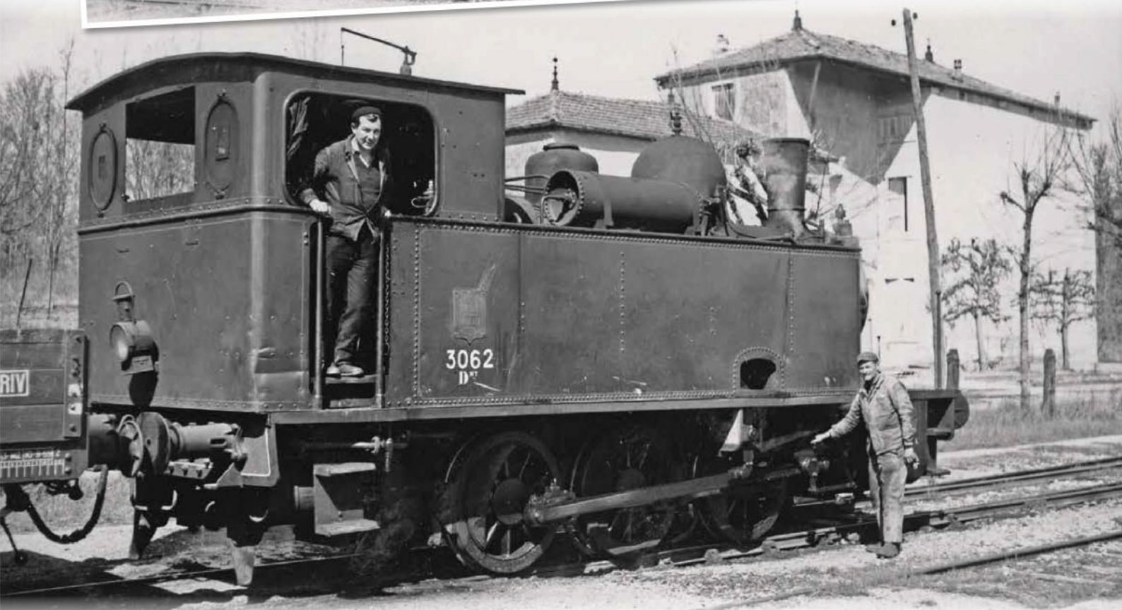
Even more so than meter gauge railways, standard gauge secondary lines often called upon stock built by industrial locomotive manufacturers, notably Belgian ones such as La Meuse or Couillet, the latter having built this 0-6-0 T used on the Guë - Ménaucourt line. (Photo Renault/Coll. R. Thévenin).
