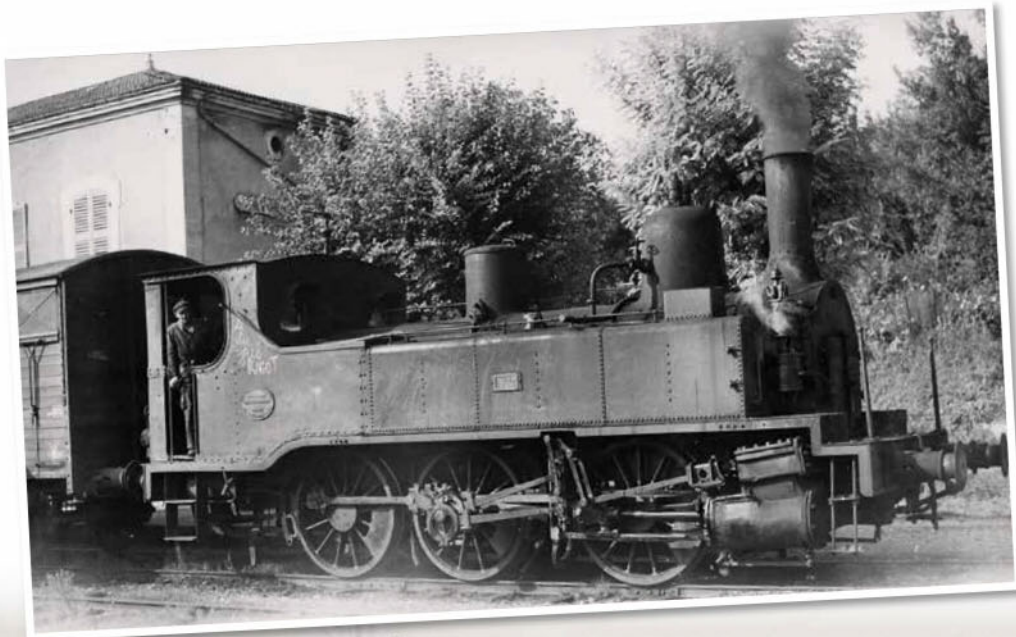
Faced with the same constraints as their meter gauge counterparts, standard gauge secondary railways also made use of 0-6-0 T locomotives. This engine, built by SACM for the Guë - Ménaucourt railway, is broadly contemporary of the first meter gauge 0-60 T engines. (Photo Renaud/Coll. R. Thévenin).
