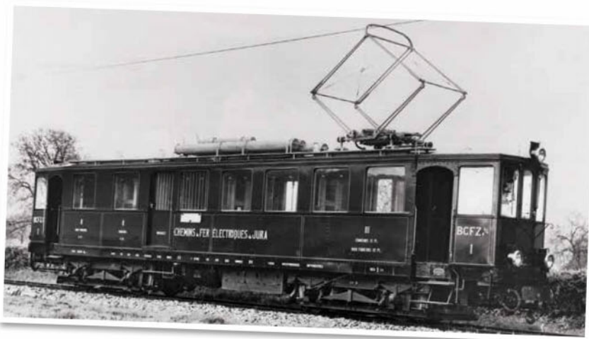
French motor-unit BCFZe4/4 1, built by Dyle et Bacalan for the mechanical part and BBC (Brown Boveri Cie) for the electrical part, seen leaving the factory in 1924. Power 4 x 70 kW. Photo BBC.
