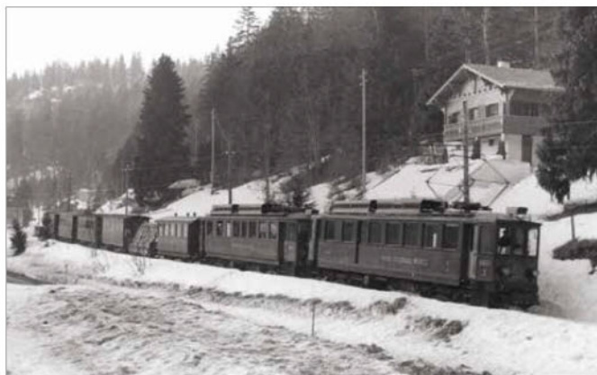
A double-headed winter sports train, with its ski wagon, seen at Crêt du Rosset, below La Givrine. Even though the train is going downhill, the pantographs have been raised to provide heating for the carriages. 12 February 1967. Photo S. Jacobi.
