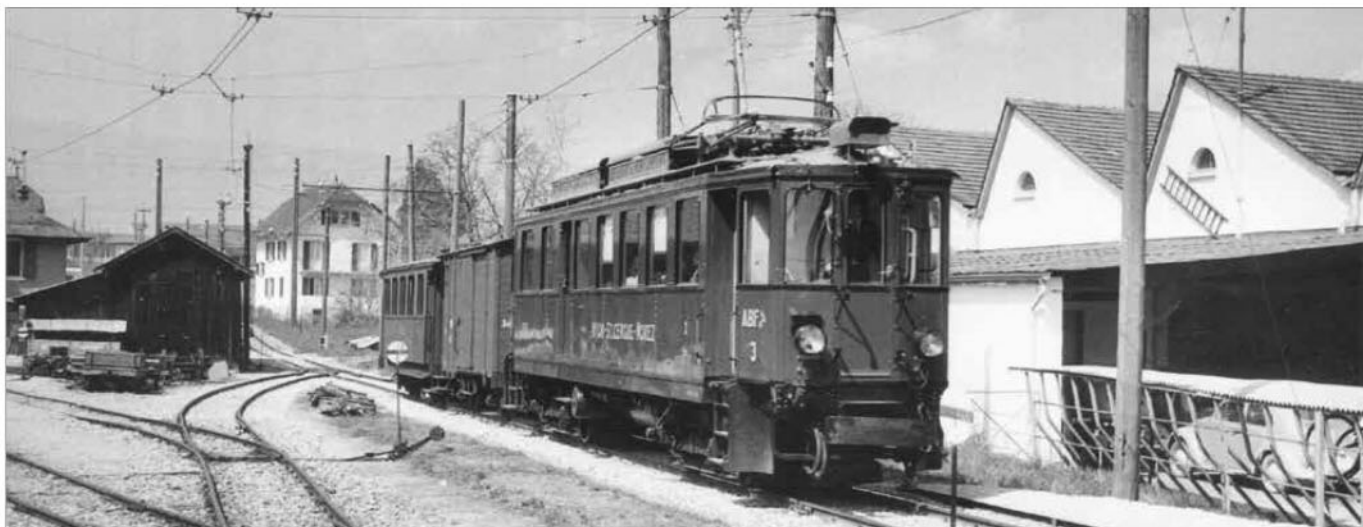
A Nyon-bound train running down from Les Plantaz, with the pantograph down. The motor-unit, ABFe4/4 3, is the former French BCFe4/4 1, renumbered. 2 May 1964. Photo M. Grandguillaume.
