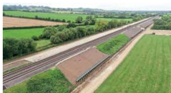
The completed embankment at Bridge Farm on Chiltern's Marylebone to Aylesbury line. NETWORK RAIL
