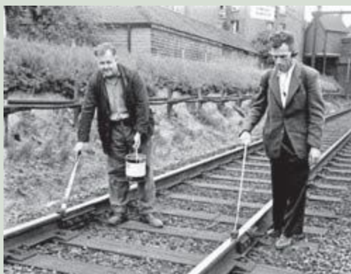
Track workers use Audigauge equipment to test rail for cracks in 1962. SCIENCE & SOCIETY LIBRARY
