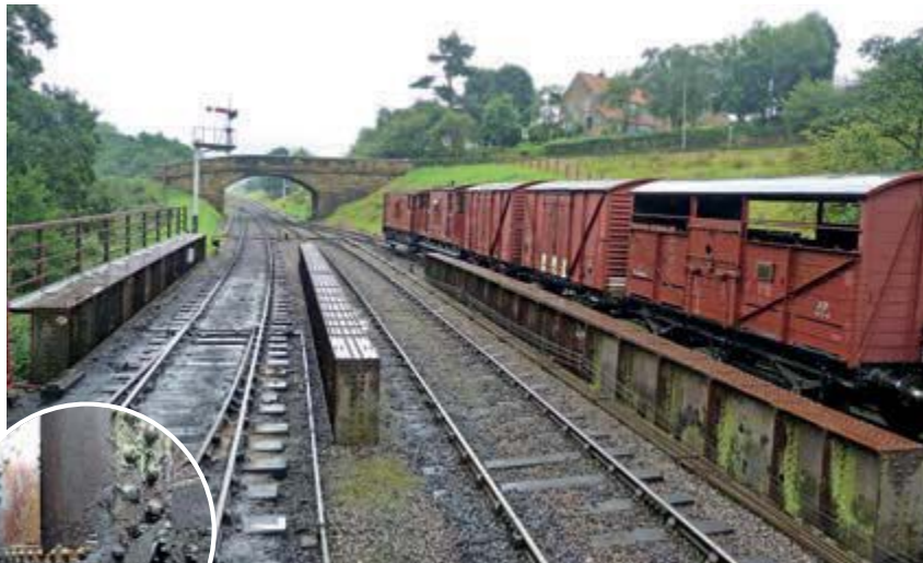
A driver's eye view of Bridge 27 at Goathland, which is to be replaced as part of the YMJ project. Inset: The extent of corrosion beneath Bridge 27 is evident here, the structure now being beyond economic repair and requiring full replacement by 2021. BOTH: GARY BOYD-HOPE
