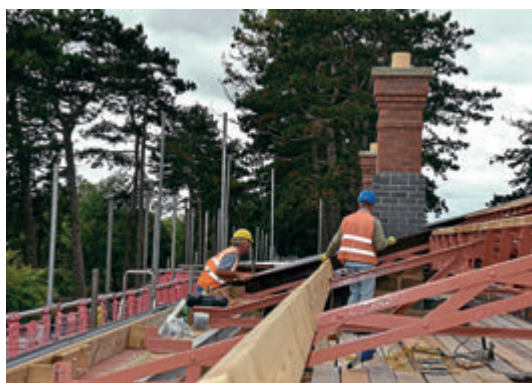
Corrugated steel being installed on Broadway station's riveted roof and the canopy frame, manufactured by the steam locomotive department. This work is now completed and the scaffolding has come down. IAN CROWDER
