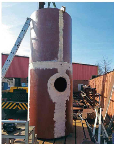
The two halves of the boiler barrel for new LMS Patriot 4-6-0 No. 45551 The Unknown Warrior lined up at LNWR Crewe in late March 2016 after one half was lifted in top of the other to be dropped into position to allow drilling and riveting to take place, with the dome hole cut out. GAVIN SHELL/LMS PATRIOT PROJECT
