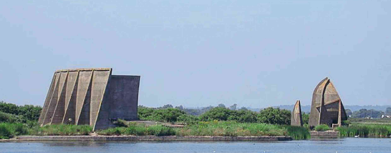
The acoustic mirrors at Denge: left to right, the 200ft, 20ft and 30ft mirrors. A short branch of the Romney, Hythe & Dymchurch Railway carried the raw materials to build them. JK SOLOMON*
