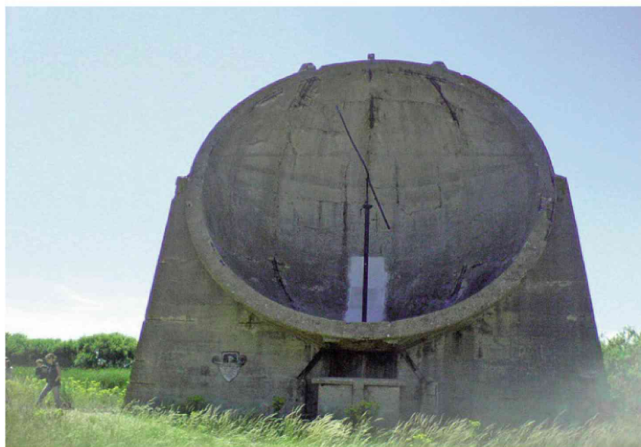
The microphone housing in one of the Denge acoustic mirrors survives. RHDR
