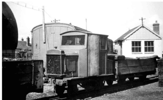
By 1950, the War Department locomotive had a makeshift cab. A major rebuild followed in the early Sixties and it was again rebuilt in 1974-75. The arrival of two diesels on the line made 'The Scooter' as it is now known redundant, but it is kept in working order and makes very occasional journeys, although the sole-surviving original part is said to be the gear differential. RHDR
