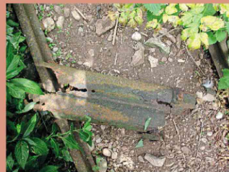
The salty air of the Severn estuary is not good for metal sleepers. ROBIN JONES
