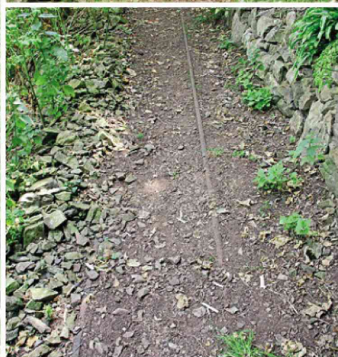
ABOVE: The Second World War railway track still in place on the zigzag incline path. The sleepers have been covered with soil to make it easier for the island's Honda Power Carrier to take supplies to the summit. ROBIN JONES
