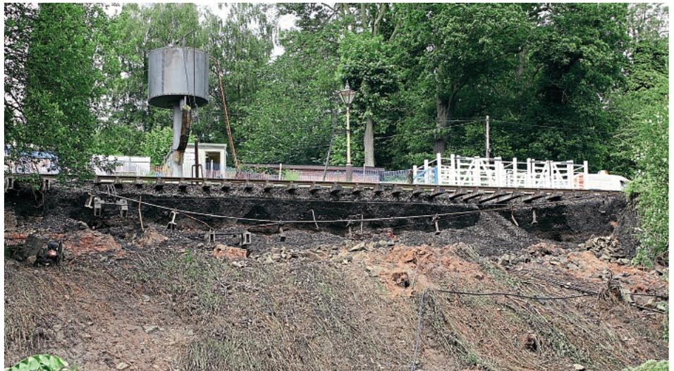
**ABOVE:** The washout beneath the track at Highley station left daylight showing between the sleepers and rails. BOB SWEET
