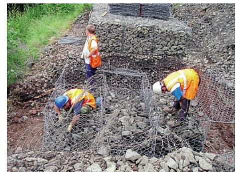
**ABOVE:** Gabions, or rock-filled cages, being placed in position at Folly Point. SVR
