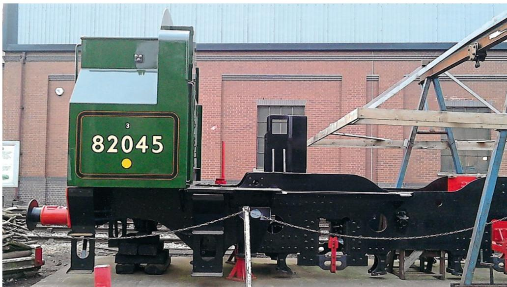
**ABOVE:** The bunker of new-build BR Standard 2MT 2-6-2T No. 82045 is fitted to the frames. PAUL APPLETON
