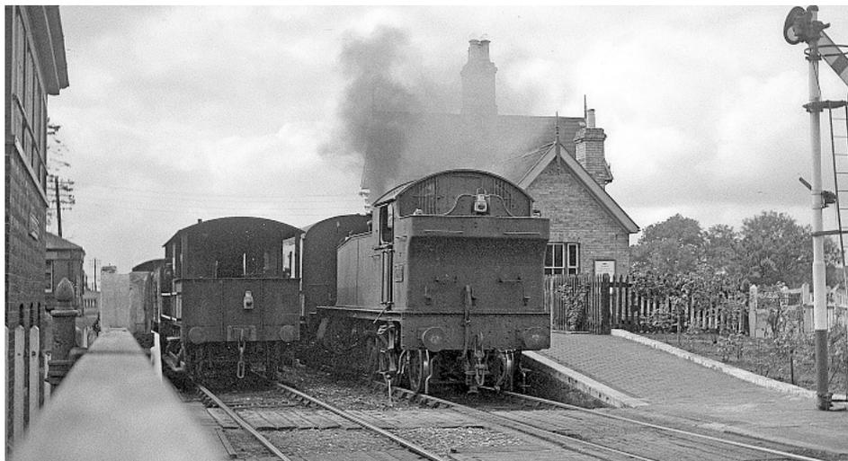
**ABOVE:** A view from track level at Cressage station on July 24, 1954. Standing in the platform bunker first with the 3.50pm Shrewsbury to Kidderminster local is GWR 2-6-2T No. 5518. On the left is a Down goods headed by GWR 2-6-0 No. 6334. On the right is a lower quadrant stop signal pulled off for the train. J WOOD/KIDDERMINSTER RAILWAY MUSEUM
