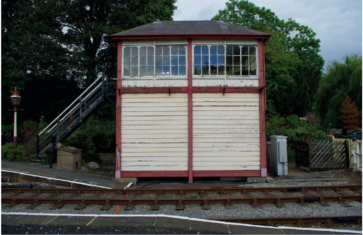
The classic British signal box is a fairly standard shape in terms of a control cabin atop a locking room. Yet within this, there is a huge variety of designs in terms of construction material, roof style, length, windows, verandas and so on. This example is an all-wooden affair at Darley Dale on the Peak Rail preserved railway.
