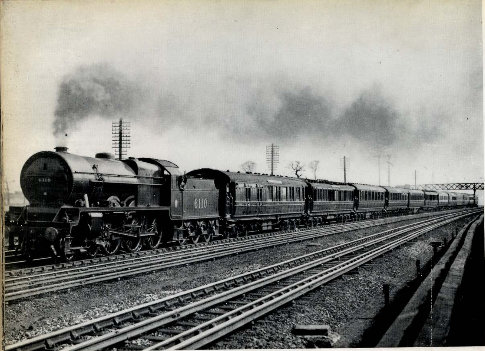
This photograph shows the forerunner of the "Mid-Day Scot" at Kenton in 1928. Heading the 1.30 p.m. Euston-Edinburgh-Glasgow express is one of the first batch of "Royal Scots", No 6110 Grenadier Guardsman of Crewe shed, built only in September of the previous year and not yet fitted with smoke shields. The first four coaches are part of the famous stock built in 1908 specially for the 2 p.m. from Euston to Scotland, a train then called "The Corridor" by the staff. Fitted with 6-wheeled bogies, they were some of the finest coaches ever built by the London and North-Western Railway.
