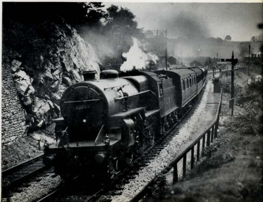
Another "Crab" 2-6-0, No 13160 (original numbering) passes Matlock in 1932 with a down fast passenger train. The Midland-pattern signal is located on the opposite side of the track to which it relates due to the curvature of the line.
