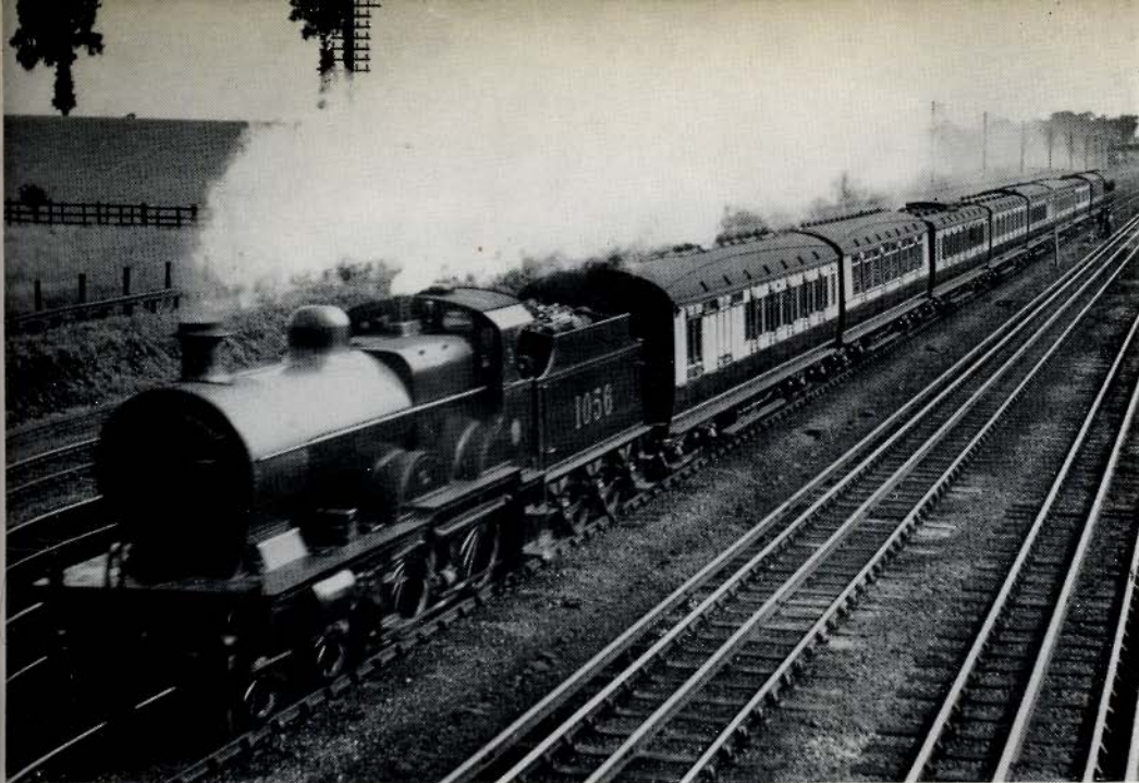
A standard L.M.S. Compound 4-4-0 No 1056 takes the 2.50 p.m. Manchester express past Kenton in 1924. With the exception of the last coach, the train is still in L. & N.W. livery.
