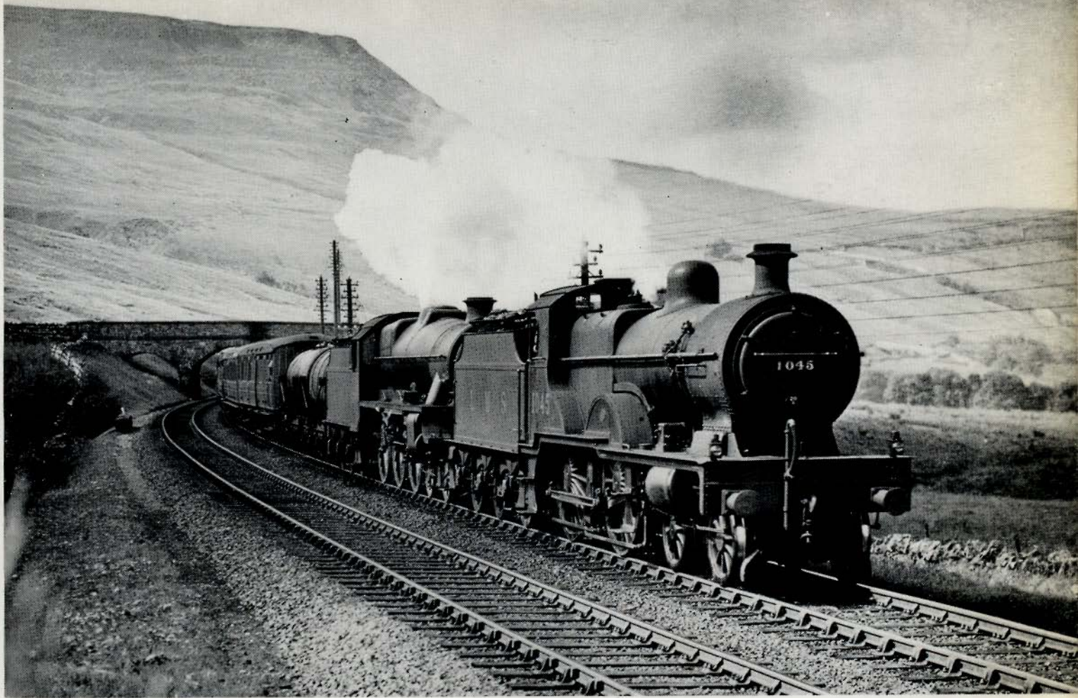
In true Midland style, a double-header! Pilot engine 4-4-0 Compound No 1045 of Leeds shed and train engine "Jubilee" 4-6-0 No 5562 Alberta steam up the last stage of the southbound climb at Ais Gill, with the 2.45 p.m. from Carlisle in 1939.
