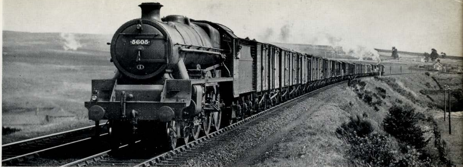
A Class "C" or "D" freight makes a steady climb on Shap in 1937. The train engine, No 5605 Cyprus of Rugby shed, is a 4-6-0 "Jubilee" in original condition, and is helped by L.M.S. "Jinty" 0-6-0T No 7338 as banker. The angle of the photograph shows the wide open spaces of the Fell country around Shap.
