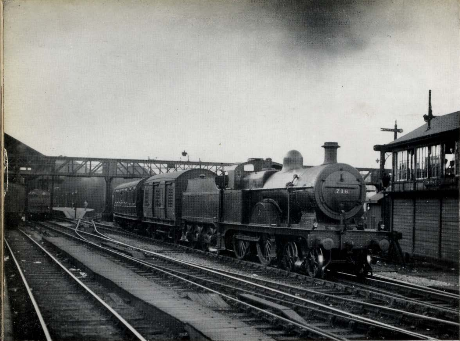
This photo shows Derby station as it appeared in 1932, complete with an over-all roof. Class 3 4-4-0 No 716 leaves with a Birmingham fast. Notice the typical Midland-pattern distant signal just showing on top of the signal box.
