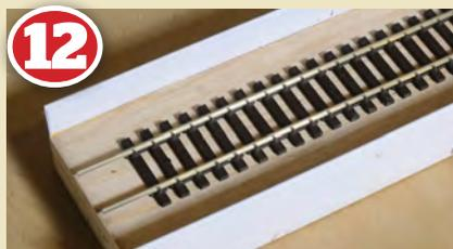
**12** Having built the cassettes they now need a means of receiving trains. Other designs have featured aluminium angle set at the same gauge as the track, but for ease of construction and operation, we elected to lay Peco code 75 track on our cassettes. The first two sleepers are removed at each end of the cassette and the track is then pinned to the 18mm plywood.
