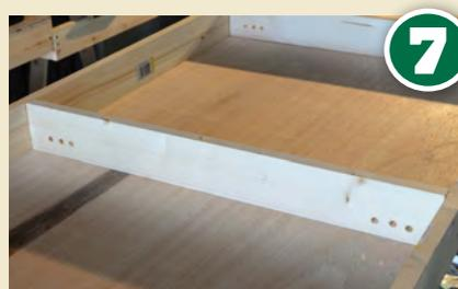
Before fitting the cross braces three 8mm diameter holes were drilled at each end of each brace for wires to be fed through. Doing this now saves a headache later. 3.5 x 35mm screws were used to fix the cross braces to the baseboard frame sides.
