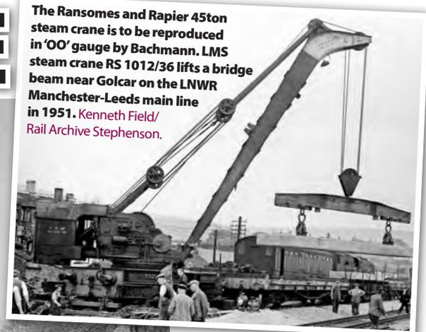
The Ransomes and Rapier 45ton steam crane is to be reproduced in 'OO' gauge by Bachmann. LMS steam crane RS 1012/36 lifts a bridge beam near Golcar on the LNWR Manchester-Leeds main line in 1951. Kenneth Field/Rail Archive Stephenson.
