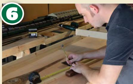
Having measured the braces for the centre of the baseboard they were marked up using a tri-square, tape measure and pencil before being cut to length.
