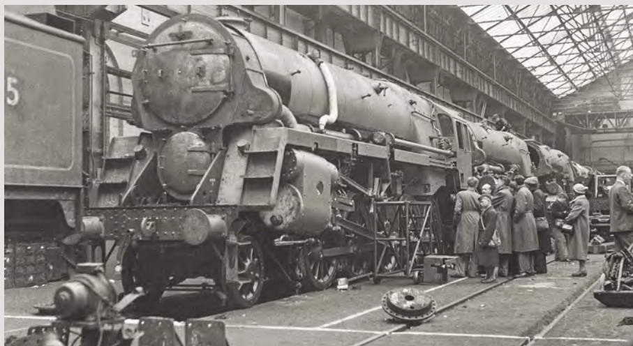
A group of visitors inspect a line of Crosti boilered '9Fs' under construction at Crewe Works in March 1955 with 92022 at the front. www.railphotoprints.co.uk
