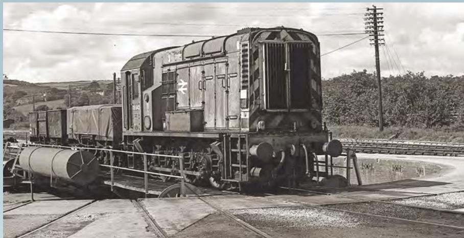
**The short length of the Class 08 played well in many situations including at depots where they could shunt with wagons onto turntables. 08643 ticks over on the St Blazey turntable on June 25 1979.**
