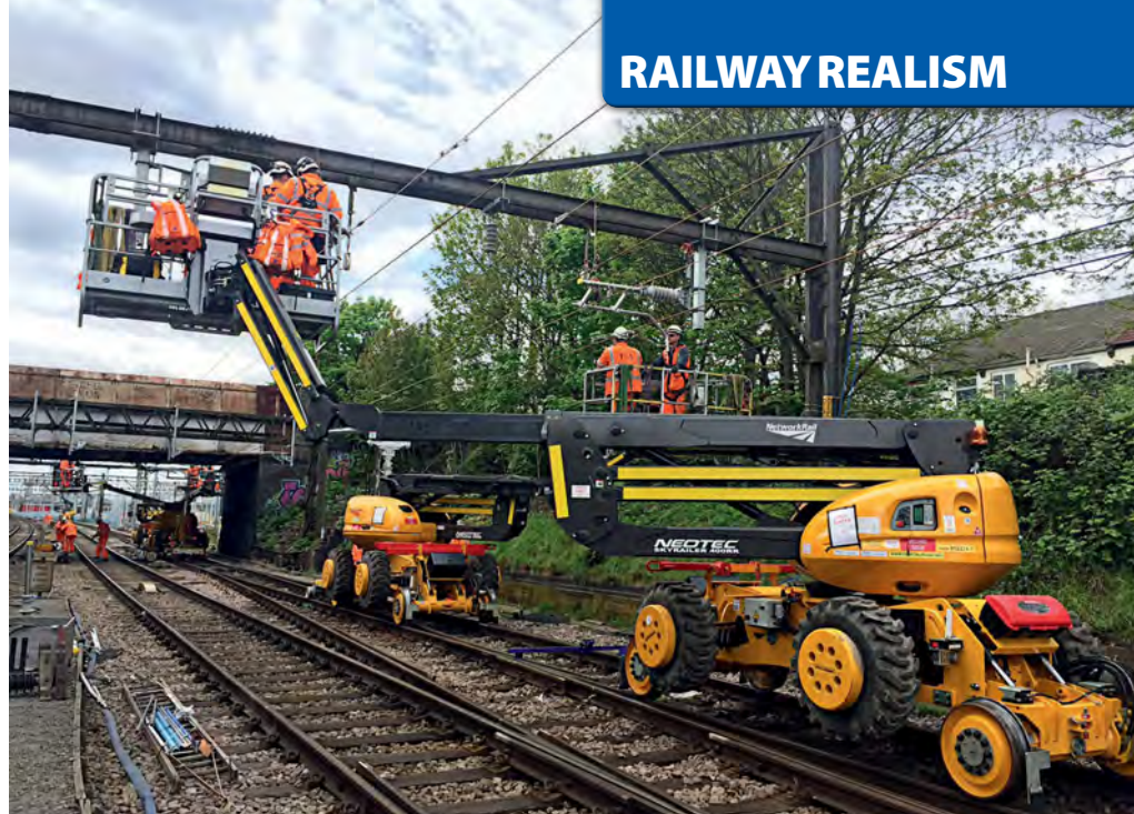
Modern day on track plant has taken on a completely different design. Here a collection of lightweight road rail platforms work on wiring at Seven Kings. Network Rail.
