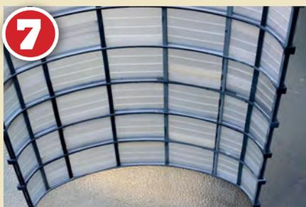
**7** Carry on adding trusses and glazing sections until each roof unit is finished. Slotting components over a framework of rods is very much on the same principles as a child's construction toy – my generation will register the similarities with Bayko!
