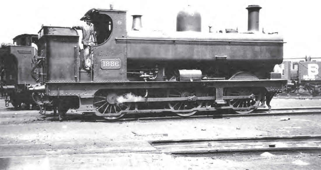
The 1854 Class was widely used in South Wales for shunting and tripping until 1950. Introduced as saddle tanks from January 1890, they were converted to pannier tanks during the 1910s and '20s. 1886 received panniers in September 1914 and was superheated in October 1921, but the elements were later removed. She is seen at the shed on 6 May 1935, being withdrawn in June 1945. (F.K. Davies)
