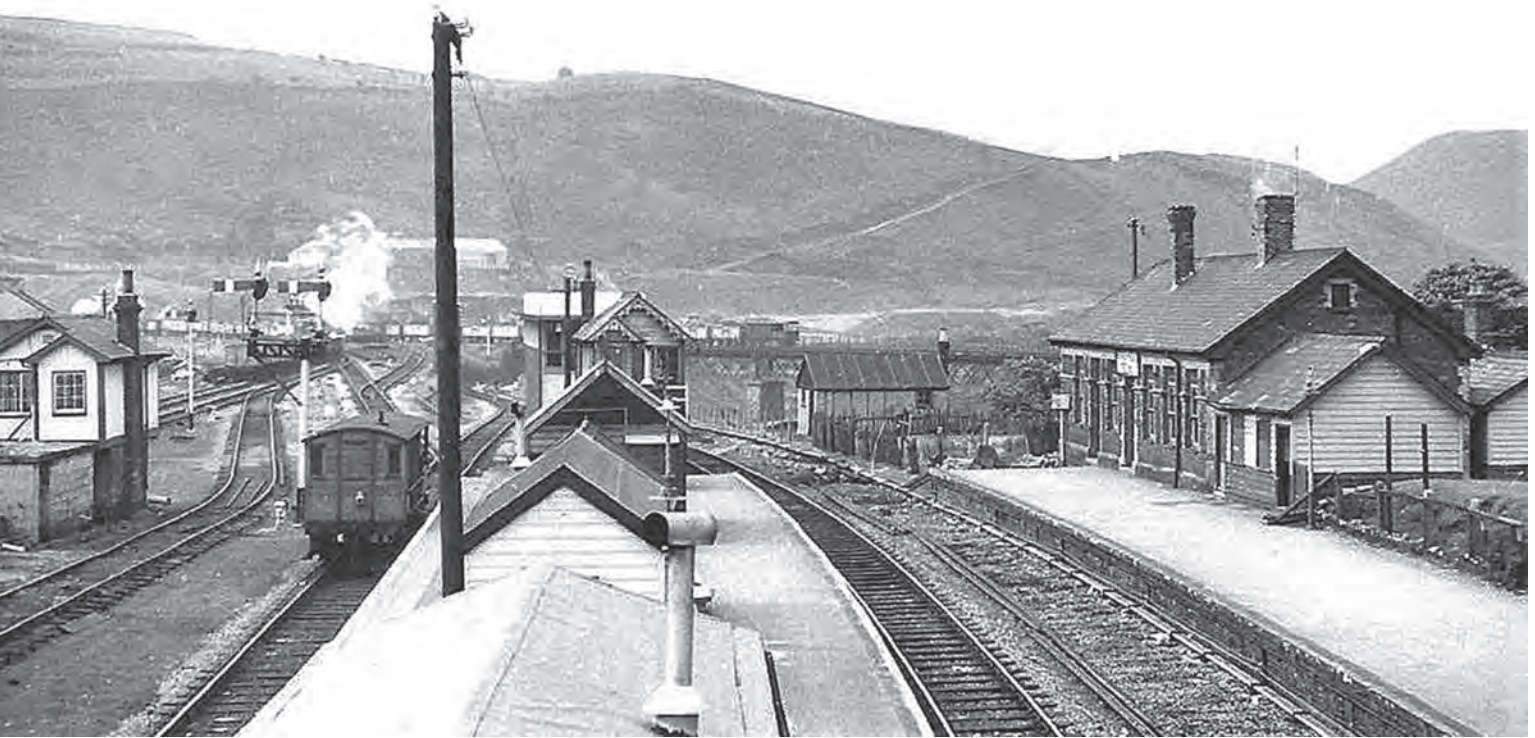
A view of the platforms at Cymmer following the remodelling on 13 June 1960, as seen on 27 September 1960. The track serving the previous northbound R&SB platform has been lifted and the Refreshment rooms marooned there. The former Down Platform had been widened and made into an Island with the track layout enabling R&SB Swansea/ Treherbert trains to use either face but the Llynvi Valley service had access only to the South face. The single platform at the adjacent Cymmer General became part of the new Cymmer Afan but was converted into a Bay Platform. Here a Brake van stands at the south end of the branch while its train engine works in the sidings below, and the new connection can be seen above the van. In this view there appear to be three Signal Boxes, on the left Cymmer General (GW) alongside Cymmer Afan (R&SBR) 'both decommissioned' and behind the latter the New Cymmer Afan. Even further behind can be seen a train of minerals coming off the viaduct from the Glyncorwg Branch. (H.C. Casserley)
