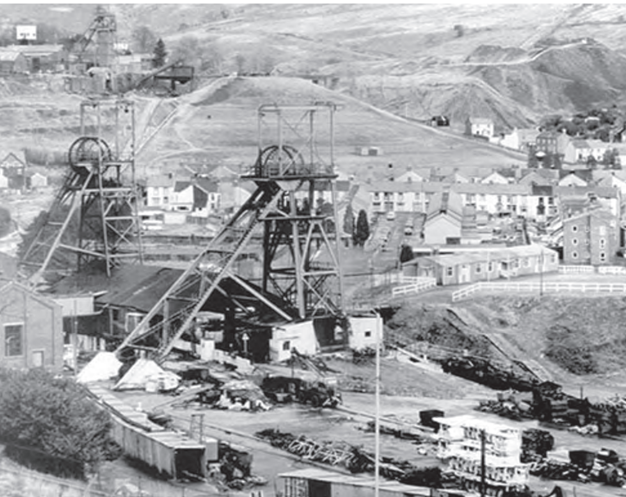
A panoramic view of the Wyndham Western Colliery with three quintessential Winding Gear towers, each at the head of a lift shaft giving access to the coalface.
