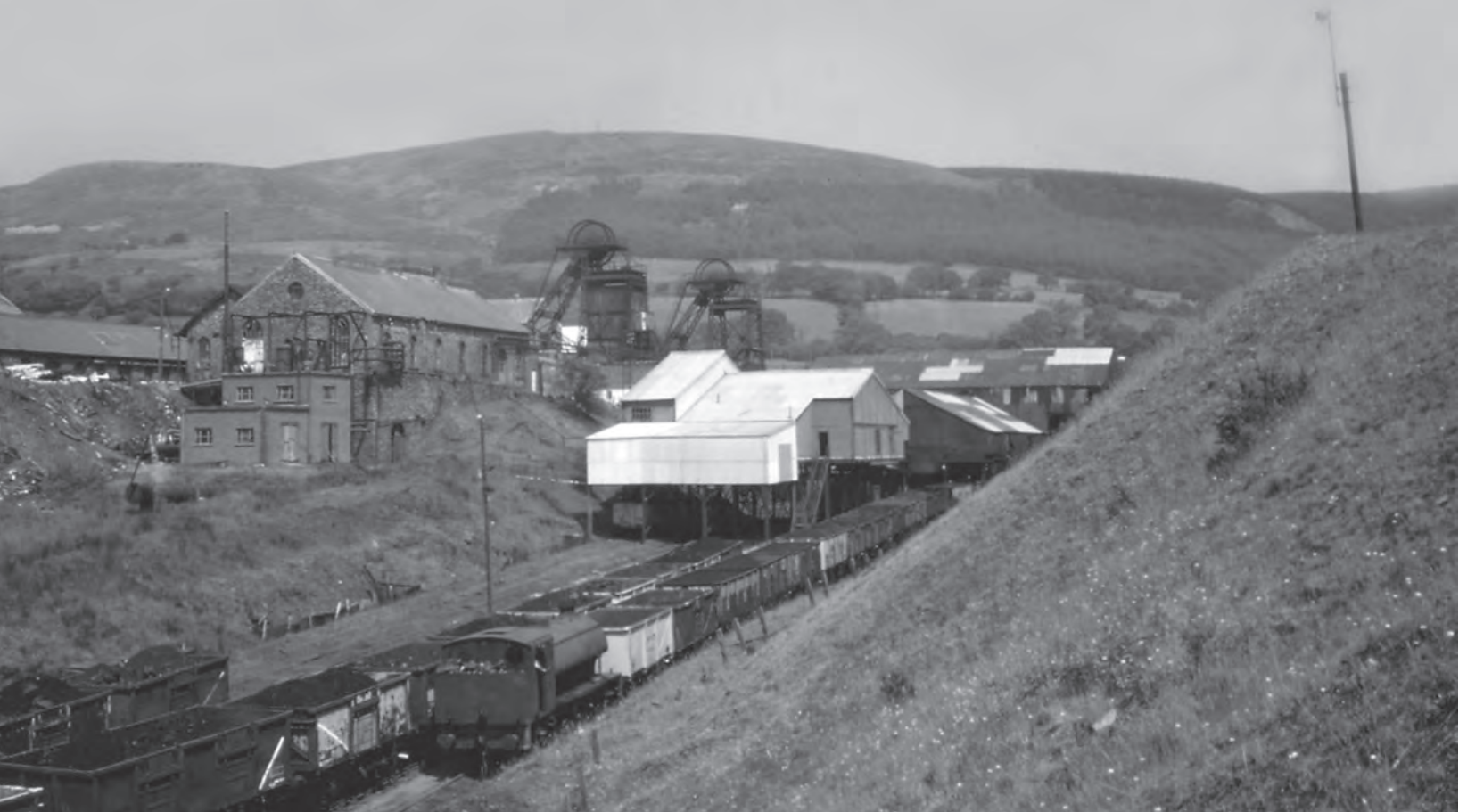
A view of the NCB loading screens and network at St. John's Colliery, Cwmdu, with Pamela shunting.
