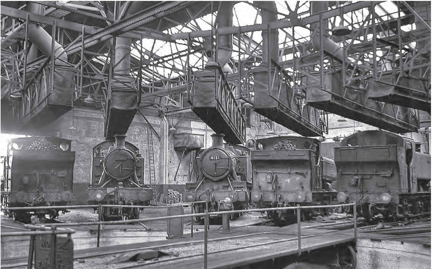
A 1960 view from the turntable and the surrounding roads with five locos from four classes but only 4121 & 5560 discernible. As with other glass-roofed roundhouses, the shed was quite light enabling photographs of the interior to be taken with ease. This view shows the smoke vents and overhead rigging to good advantage. (John Wiltshire)
