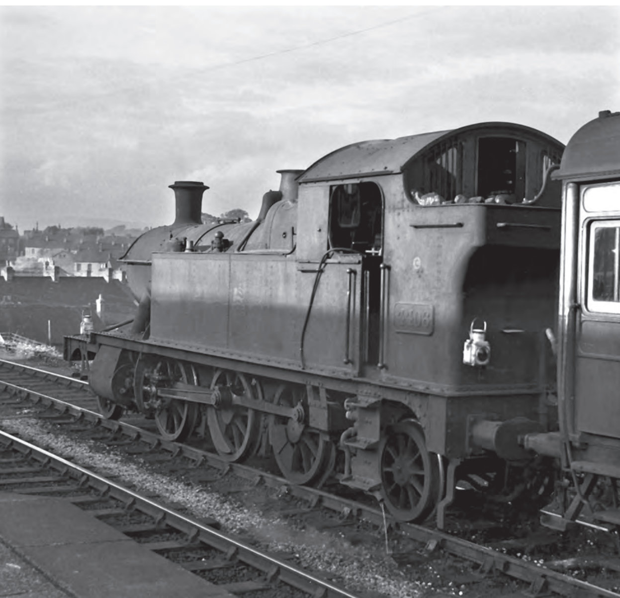
Bridgend with 4406 standing at the head of empty coaching stock consisting of a pair of ex-Taff Vale Railway Auto-Coaches on 18 September 1954. 4406 was not auto fitted and this photo was taken just after the arrival of some of her larger 4575 class sisters that were modified in 1953 for widespread Auto working at Tondur which saw the demise of 4406. (B. Moone/Kidderminster Railway Museum)
