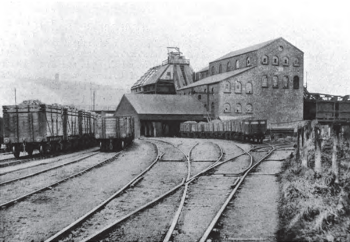
Central Washery at Tondy next to Tondy South Sidings with coke wagons on the left and wagons receiving washed coal on the right. The Washery was replaced by new ones at Maesteg and Caedu just to the south of Ogmore Vale.
