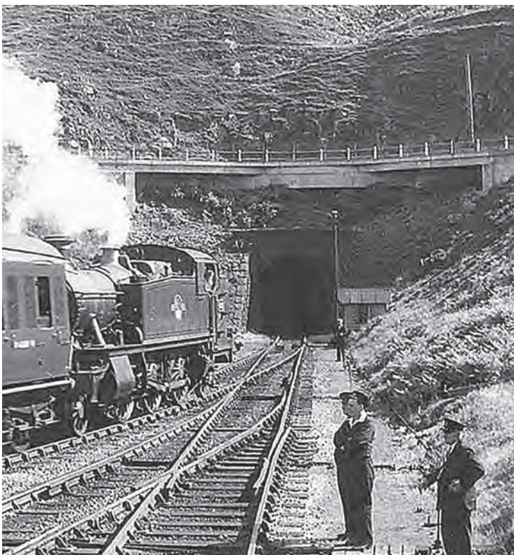
The entrance to Cymmer Tunnel as seen on 13 July 1959. The three tracks are the single running line (left), the lead into the four sidings (centre) and the track crossing the Glyncorrwg Viaduct (right). The ground frame to operate the last two is on the right of the tunnel mouth. (H.C. Casserley)
