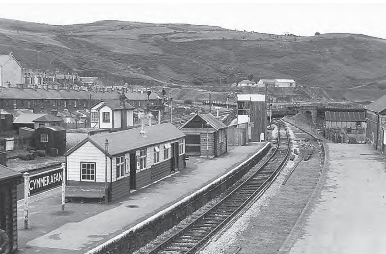
A view of the platforms at Cymmer following the remodelling on 13 June 1960, as seen on 27 September 1960. The track serving the previous northbound R&SB platform has been lifted and the Refreshment rooms marooned there. The former Down Platform had been widened and made into an Island with the track layout enabling R&SB Swansea/ Treherbert trains to use either face but the Llynvi Valley service had access only to the South face. The single platform at the adjacent Cymmer General became part of the new Cymmer Afan but was converted into a Bay Platform. Here a Brake van stands at the south end of the branch while its train engine works in the sidings below, and the new connection can be seen above the van. In this view there appear to be three Signal Boxes, on the left Cymmer General (GW) alongside Cymmer Afan (R&SBR) 'both decommissioned' and behind the latter the New Cymmer Afan. Even further behind can be seen a train of minerals coming off the viaduct from the Glyncorwg Branch. (H.C. Casserley)
