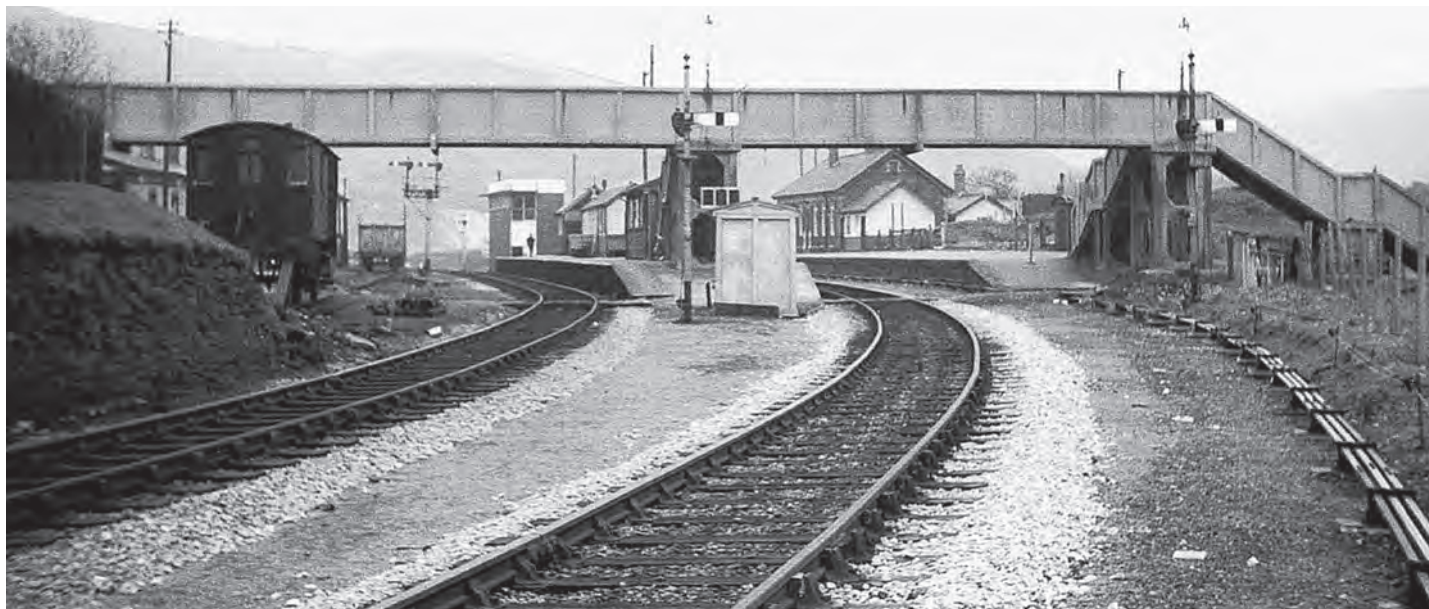
A view on 28 March 1964 from north of the station showing the former north-bound R & S B platform on the right, the island platform centre and the station siding on the left. The signal box is at the south end of the island platform. (Jeff Stone)
