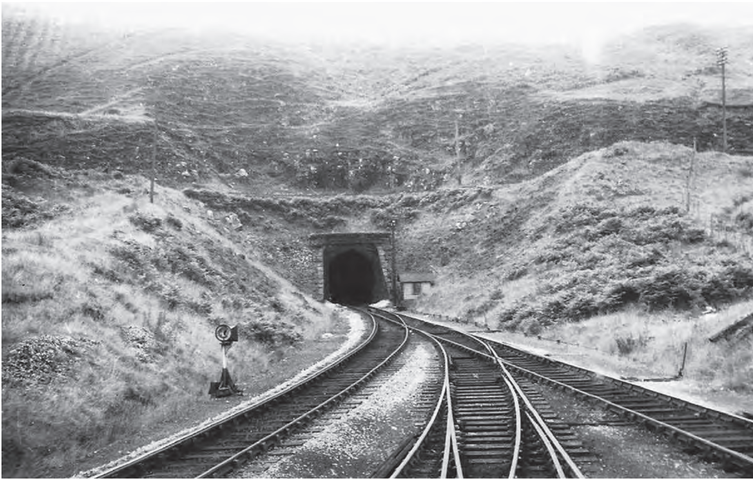
The entrance to Cymmer Tunnel as seen on 13 July 1959. The three tracks are the single running line (left), the lead into the four sidings (centre) and the track crossing the Glyncorrwg Viaduct (right). The ground frame to operate the last two is on the right of the tunnel mouth. (H.C. Casserley)
