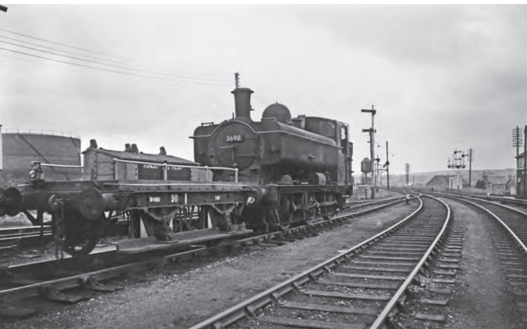
Ogmore Yard with 3690 and Shunters' Truck 41812. Built and allocated to Tondur in 1895, the Chariot, Gig or Runner depending on locality, conveyed a Tool Box equipped with spare head, tail and side lamps, shunting poles, brake sticks, spare coupling links but most importantly two re-railing ramps.
