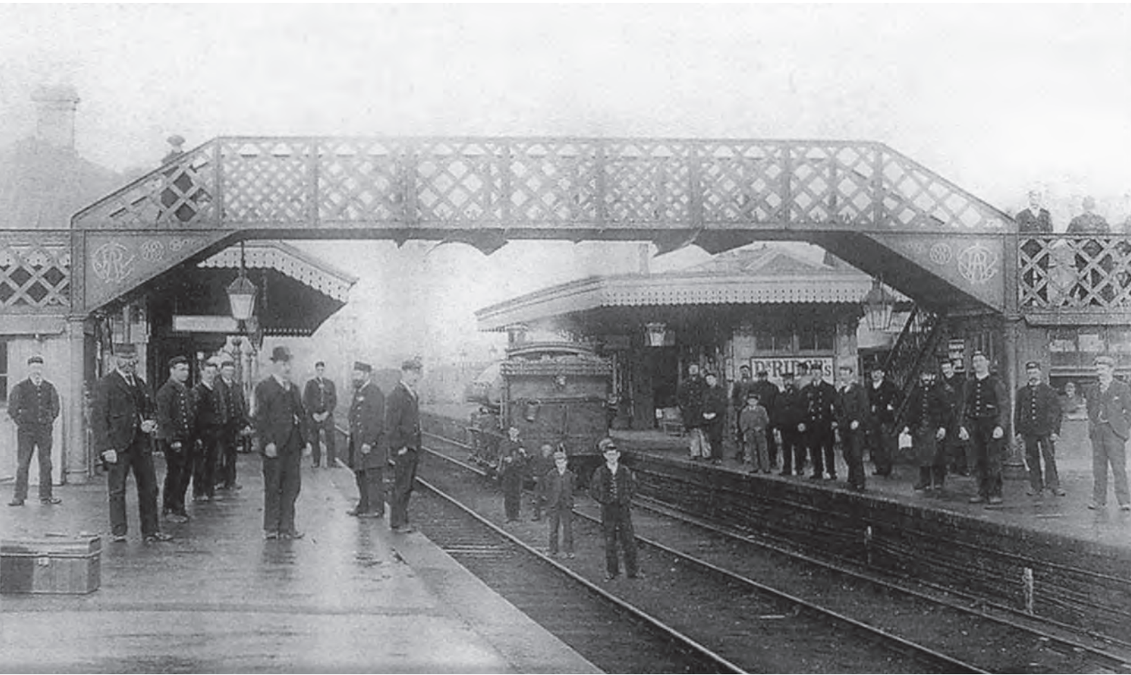
Bridgend c1900 with the station staff posing for an unrecorded event. Meanwhile, a Buffalo Class 0-6-0T is in the process of running round one of the Tondy Valleys services in the adjacent platform 4 by means of the Up Main Platform 3. Bridgend opened on 18 June 1850 but the footbridge dates from 1884 and is seen here before the fitting of its protective canopy and sides. (Courtesy of Colin Prosser)
