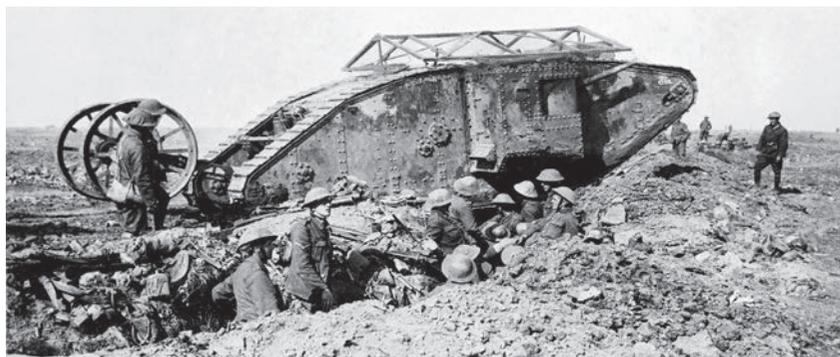
An early model British Mark I 'male' tank, named C-15, near Thiepval, 25 September 1916. Note that the tank is fitted with the wire 'grenade shield' and steering tail, both features which were discarded in the next models.
