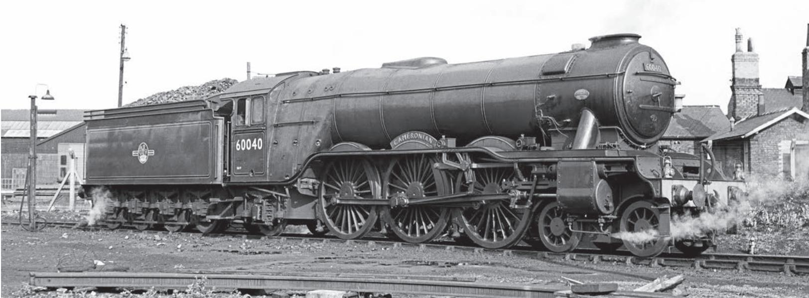
Gresley 'A3' Pacific BR No 60040 CAMERONIAN with lipped double chimney is seen in the shed yard at Darlington depot in May 1960. The locomotive is coupled to a ex GNR tender with coal rails, which has the later BR so called 'ferret and dartboard' logo. Note the Doncaster Works maker's plate mounted on the smoke box and the 'RA9' route availability indication shown on the bottom left cabside panel. The locomotive had BR Brunswick Green, orange and black lined livery. *Norman Preedy Collection*
