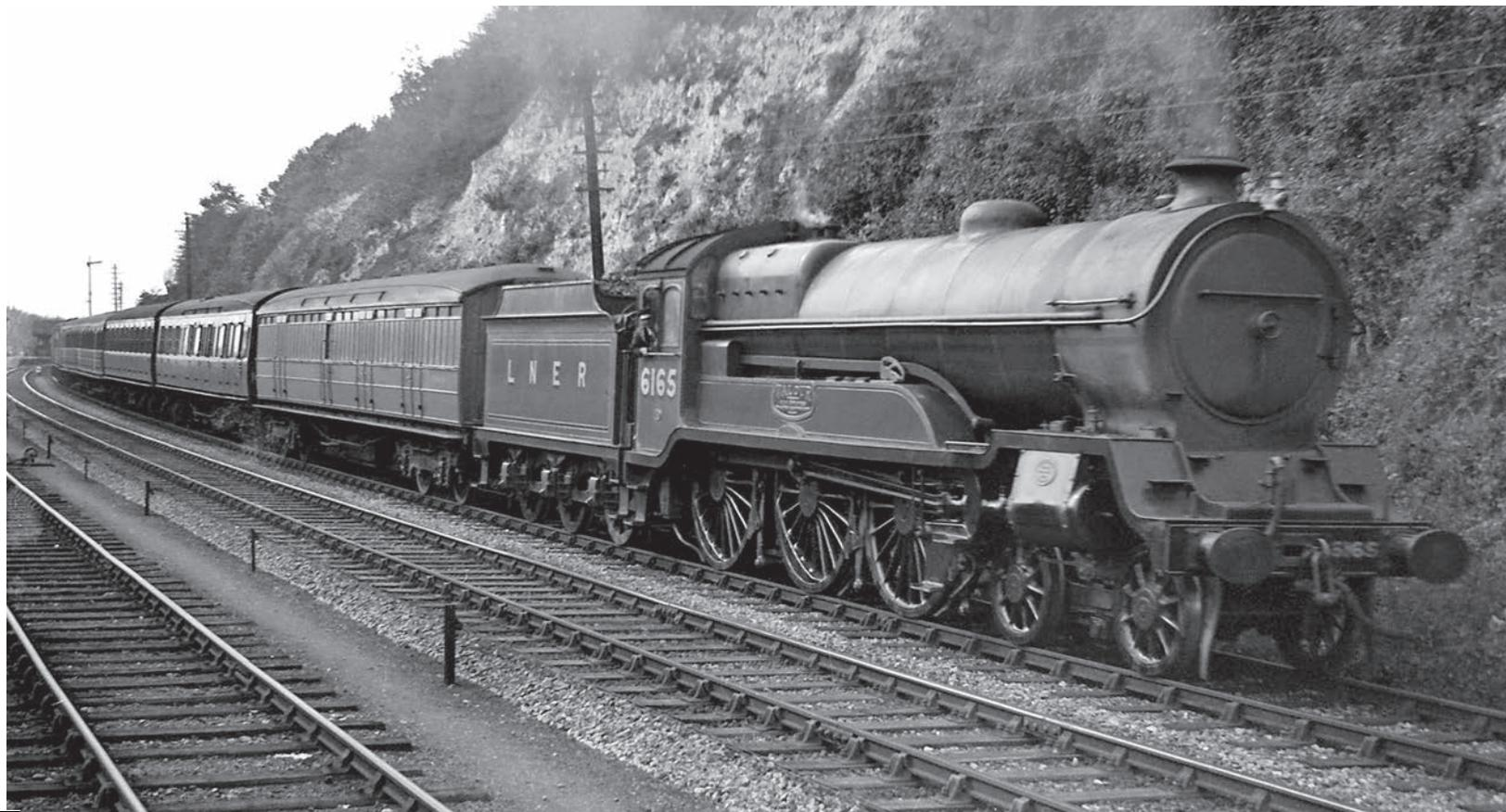
**GCR No 1166 EARL HAIG**, (LNER 6166 and 1497) built at Gorton Works, Manchester, the locomotive entered traffic August 1920 and became an LNER engine at 'Grouping'. Rebuilt in December 1929 as a B3/2 and rebuilt again in October 1943 as a B3/3. Allocated BR No 61497 in 1948, withdrawn and cut up by BR in April 1949.
