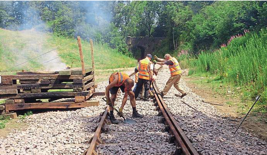
Fitting a check rail on one of the tight radius curves. MALCOLM LAW
