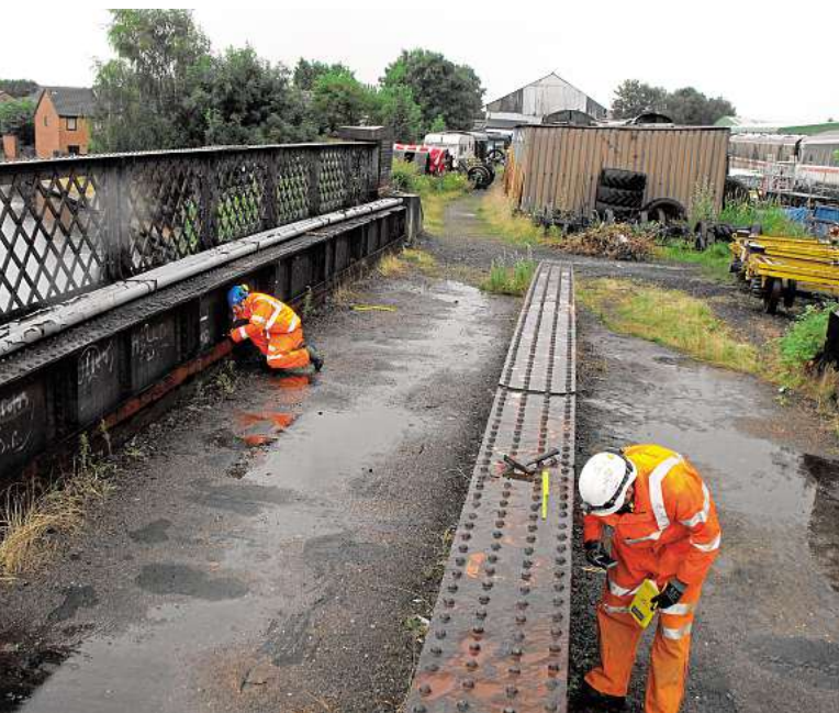
Surveyors examine the parapets and decking of the Grand Union Canal bridge. GCR
