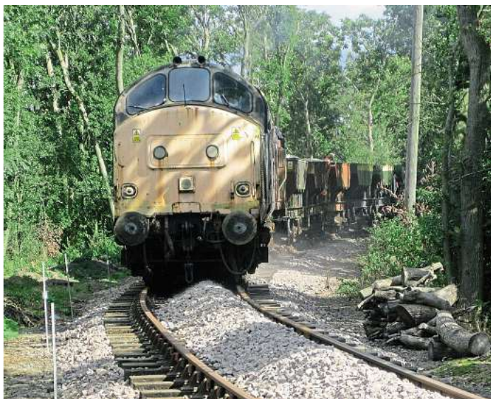
A Class 37 would never have visited the branch in its operational days! Ballast laying is seen in progress in 2012. MALCOLM LAW
