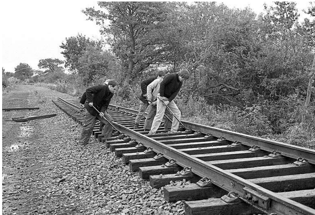
Early tracklaying being carried out on the extension to Leicester North. DENNIS WILCOCK/GCR
