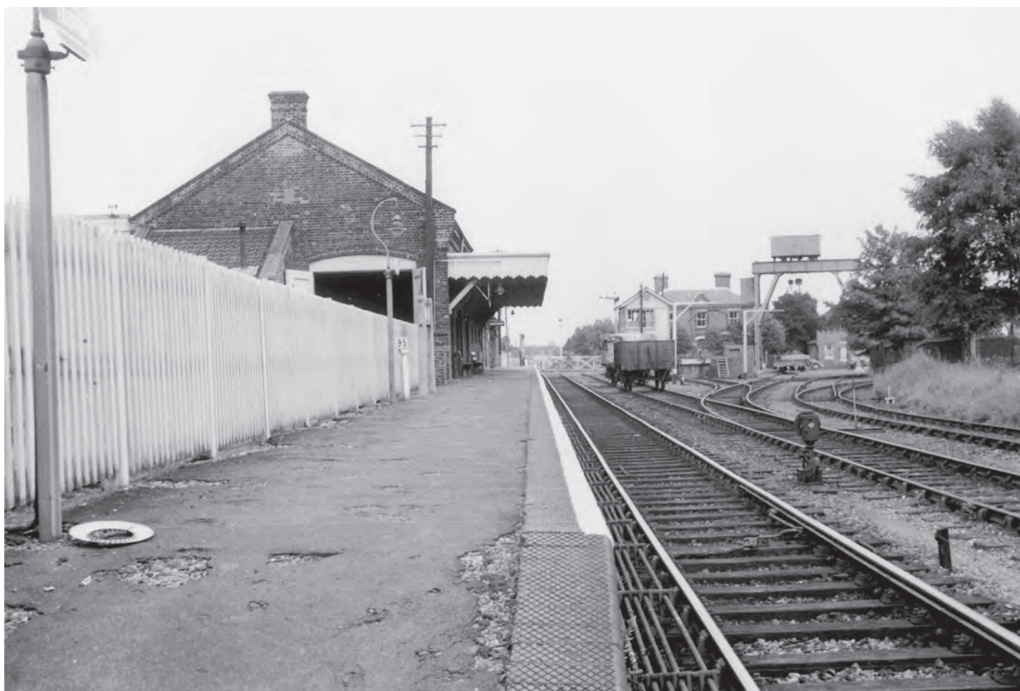
Here is Leiston station looking towards Aldeburgh, with the lines to Garrett's works curving off to the right. Note the lower quadrant signal beyond the signal box. 8 September 1960.
