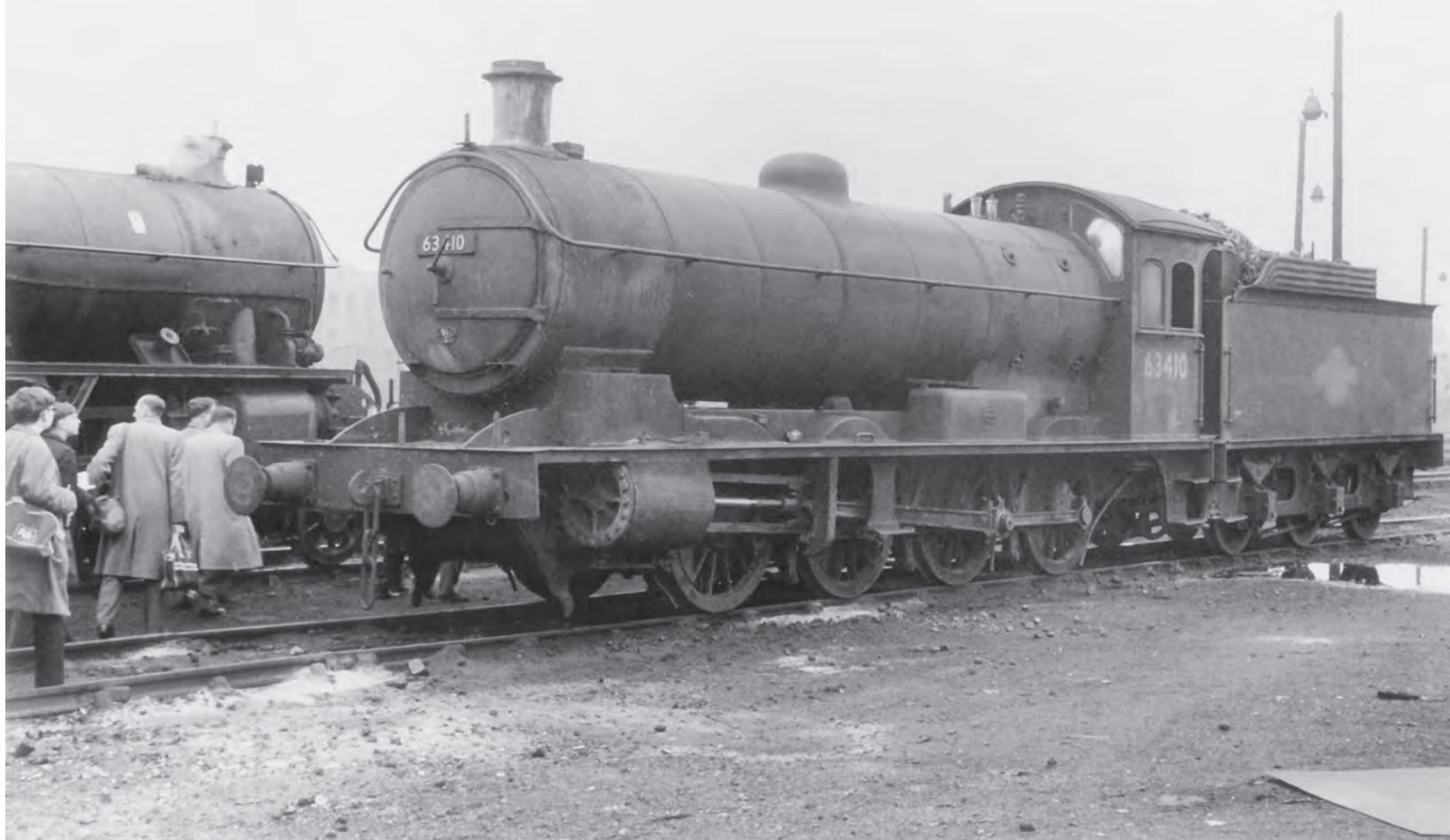
West Hartlepool's 'Q6' 0-8-0 63410 is resting at Darlington after exertions that have burned its smokebox door, and priming could be the cause of decoration to the chimney.
