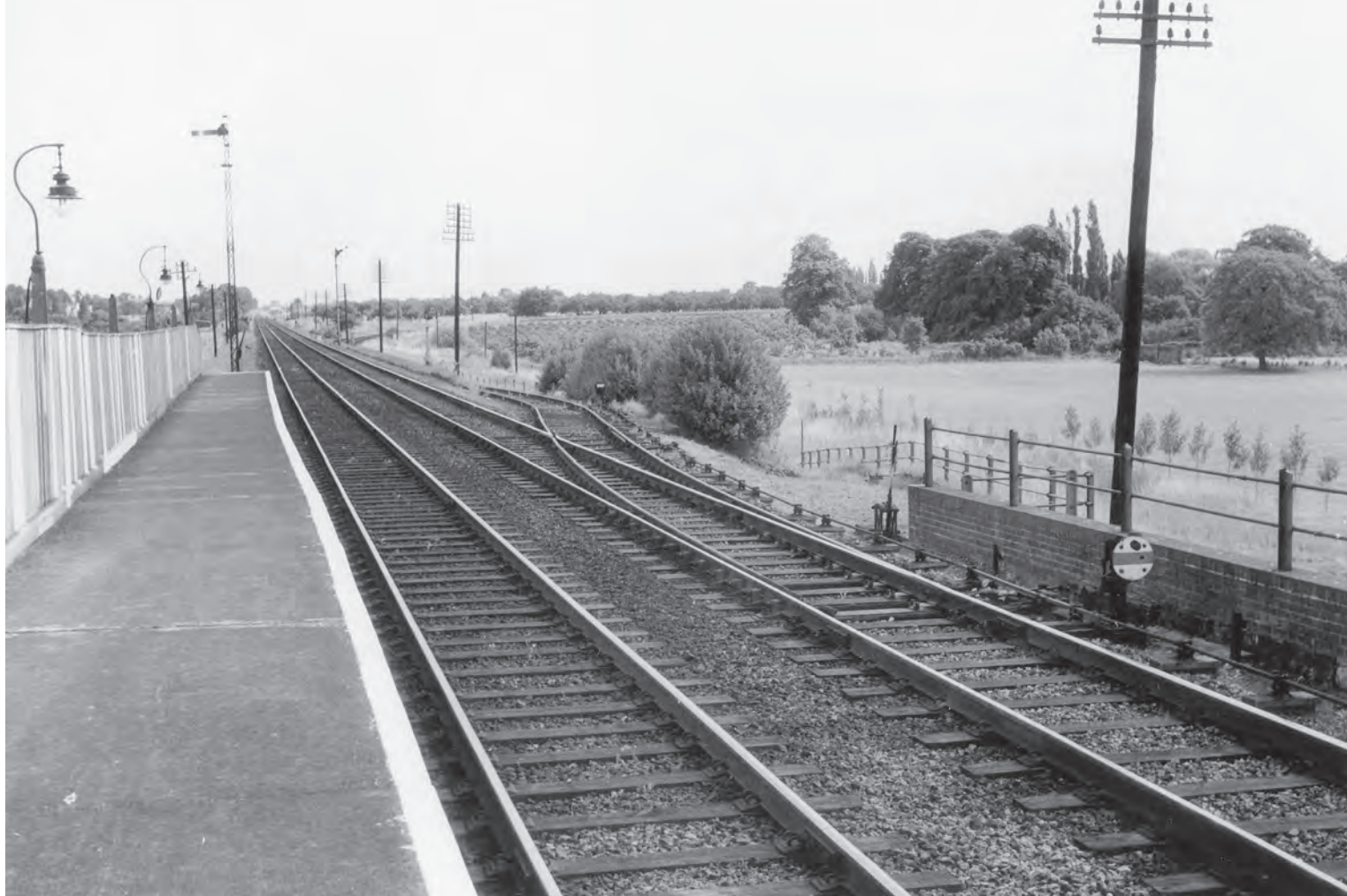
Kelvedon's up home signal is expectant, whilst the view portrays the junction with the Tollesbury branch, dropping away from the main line and then curving to the south. The branch was open for freight traffic to Tiptree for the jam factory. This view is looking towards Feering Halt.
