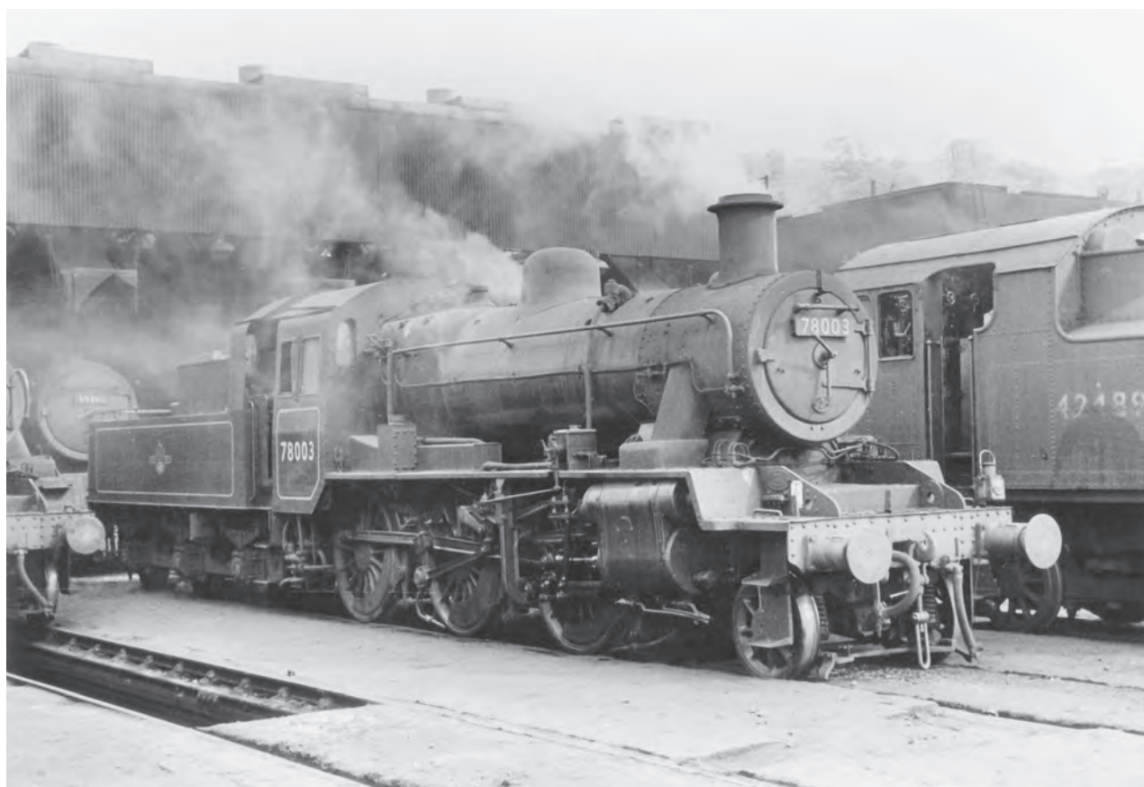
Bangor shed was very close to the station, so it seemed appropriate to make a visit. Resident Stanier '4MT' 2-6-4T 42489 is on shed. Note Bangor West End signal box in the distance behind 42489. 7 June 1964.
