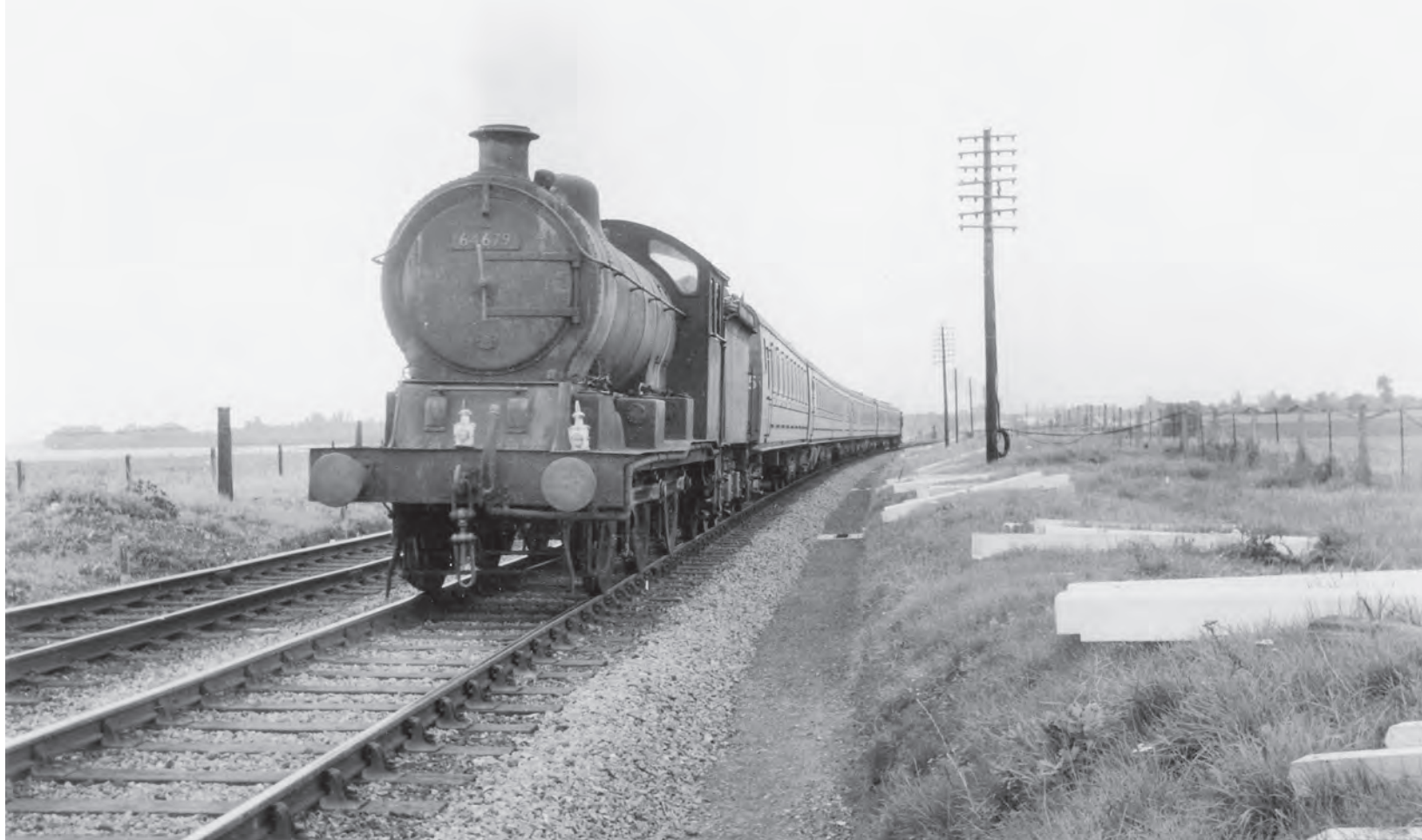
Another electric unit is being returned to Ilford, headed by A.J. Hill designed 'J20' 0-6-0 64679. These locomotives were rebuilt with 'B12/1' boilers with round topped fireboxes.
