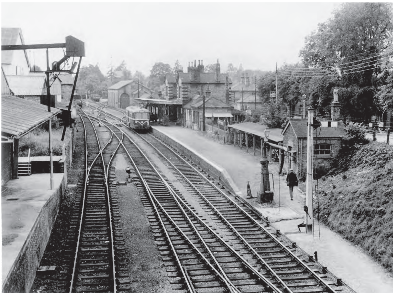
Saffron Walden station looking west towards Audley End. Steam age equipment is still obvious and the semaphore signal has a wooden post, whilst the smoke besmirched goods shed is beyond the station.
