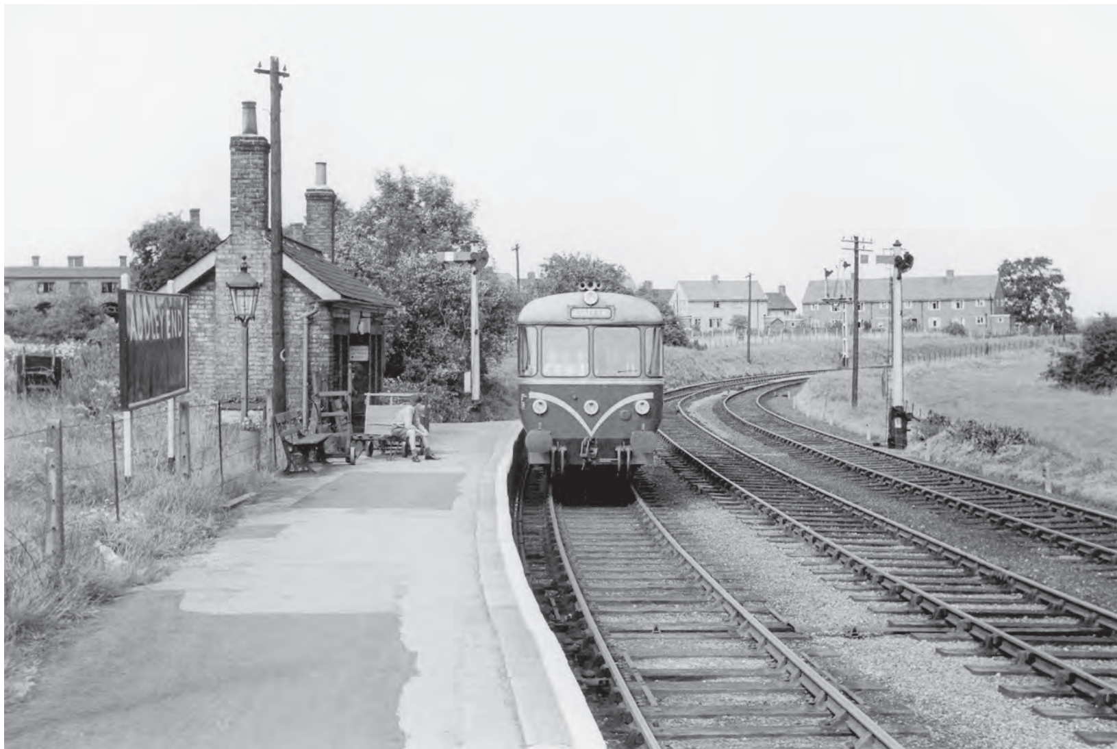
This is the branch platform at Audley End with the railbus arriving from Saffron Walden. Two lower quadrant semaphore signals complete the scene.
