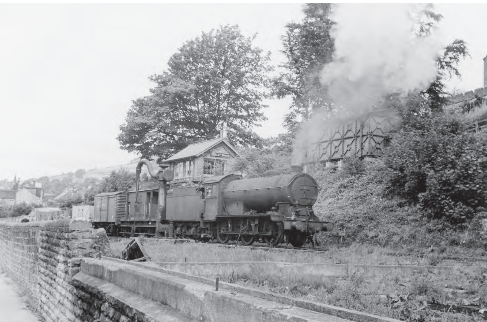
Starbeck allocated 'J39' 0-6-0 64861 is backing wagons into the yard at Pateley Bridge. Note the signal box is out of use with its windows smashed, although the name board is still present. The water column has an elegant swan neck, the water being supplied from the large tank seen above 64861.
