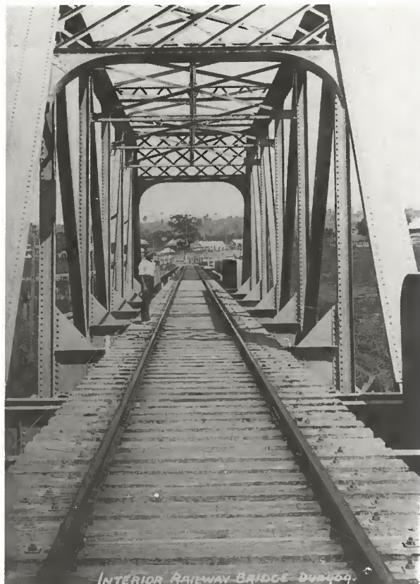
Truss bridges such as this abound on the North Coast Railway, between Maitland and South Brisbane. The Williams River bridge, a few hundred yards north of Dungog station, is shown, the photograph taken c.1913 from the northern end, with part of the old, historic town in the distance. G. Kelly
