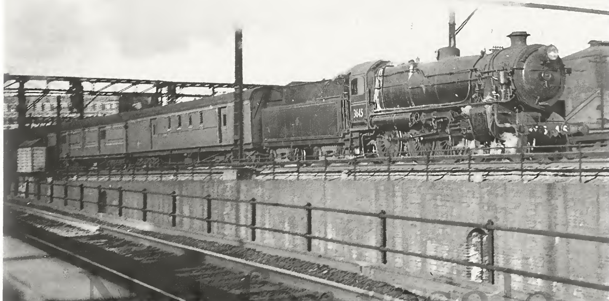
The first of the procession of mail trains ex Sydney was No.7 North-West Mail, seen here behind Belpaire-boilered 3645 as it steams past Eveleigh on 1 August 1955 with the KP mail van prominent behind the locomotive.
