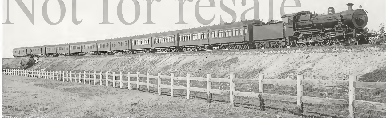
NN1028, later 3502, was very new when photographed at the head of a posed 'express' train in 1914. A KP mail sorting van, itself new, is the second last vehicle, behind five attractive 72'6" twelve-wheel cars, these being two TFX second class and one TBC first class sitting cars, a TAM sleeper and a CAM composite sleeper, with an EHO van as the last vehicle. SRA Archives
