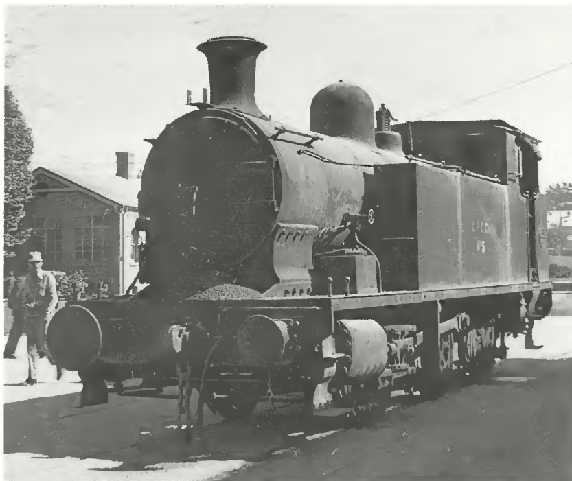
On Anzac Day 1960, a Steam Tram and Railway Preservation Society tour, returning from a weekend in the west, paid a visit to the Portland cement works. The works' locomotives were placed around the yard for inspection. This interesting view of No.5 shows a number of features that were changed after the locomotive had its rebuild in the late 1960s. The large buffers were replaced with smaller ones, the link coupling was removed and an automatic knuckle coupler installed in its place. Headlights were fitted after the overhaul and the wording 'CPC Co. No.5,' stencilled on the locomotive's water tank, disappeared.
