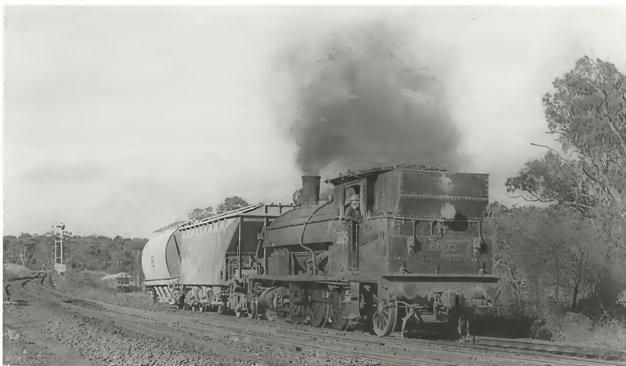
2605 shunts wagons in the down sidings at Portland station prior to returning to the works on 25 August 1973. Various wagon types were usually kept on hand in these sidings and transferred to the cement works for loading as orders warranted. The main line can be seen to the left, climbing towards Pipers Flat on a rising 1 in 50 grade. It was this grade that necessitated special operating conditions when trains were shunting Portland station to help avert any possible run-aways.
