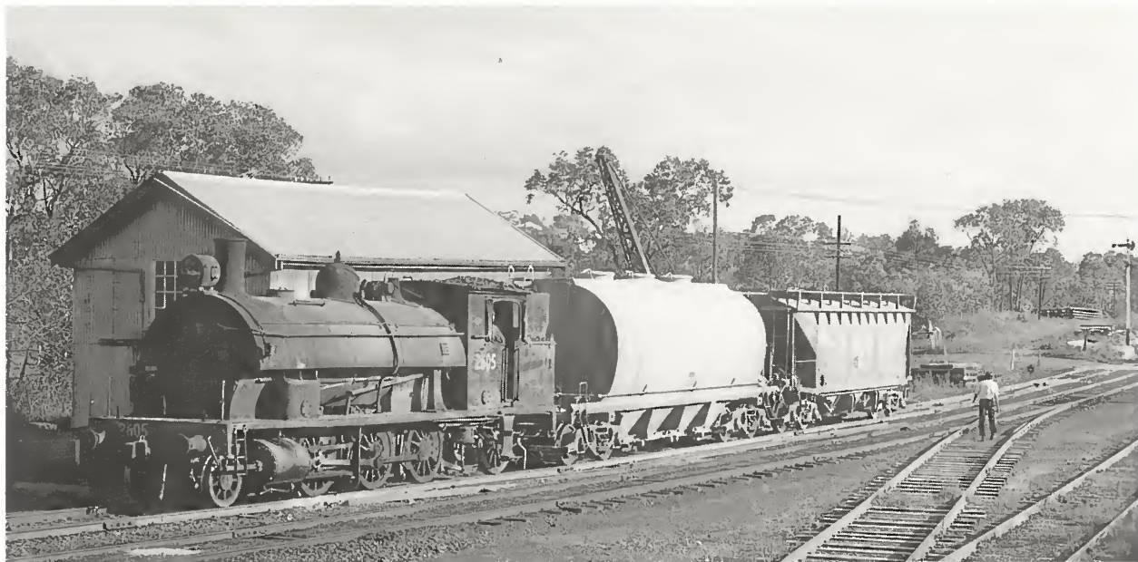
2605 eases to a halt in the goods siding at Portland station while the station assistant walks back to close the Williewa Street gates. The locomotive will then propel its load, consisting of ARX and FRH wagons, into the storage siding to await collection by the afternoon government train on 25 August 1973. Even at that time, the goods shed and adjacent crane were seeing very little activity.
