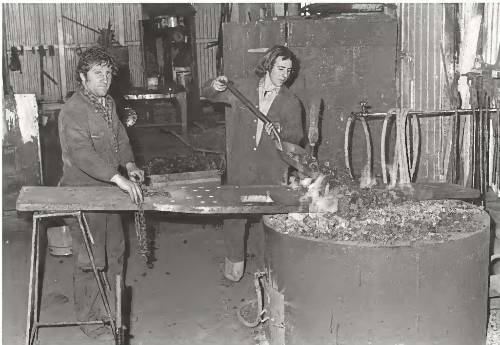
Peter Broadhead (at left) and Michael Marmont indulge in a little blacksmithing the old way, when straightening 3642's accident-damaged buffer beam.
