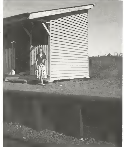
Left: The station office at Tamrookum was of simple fibro-cement construction and contained a desk for the signalman on duty as well as a bed for the use of officers sent there on relief. Signalman Wal Jenkins stands near the office with the staff exchanging platform and oil lamp to the right.
