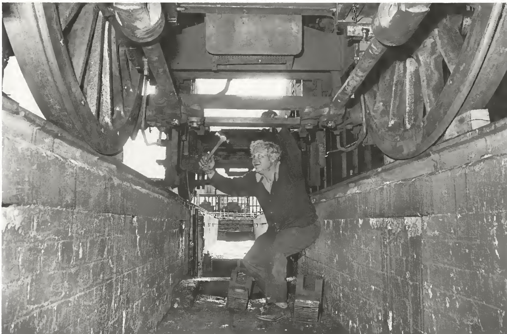
Senior fitter, the late Les Peterson, drives home a pin in the old express locomotive's brake rigging during re-assembly of the locomotive. The new boiler was yet to be restored to the frame.
