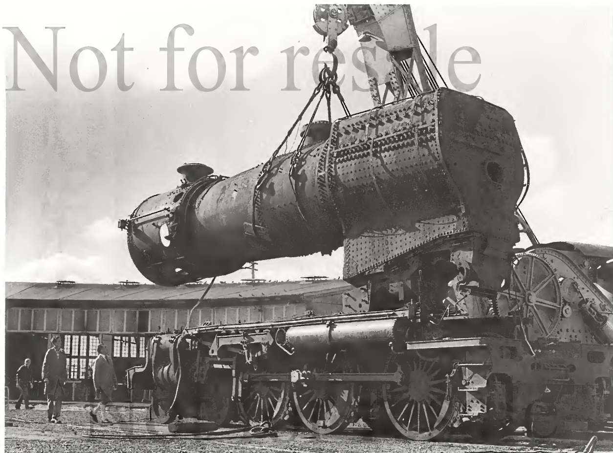
3642's old boiler, No. 3642B, swings from the jib of steam crane 1048, marking the start of the engine's complete restoration. The date: 19 March 1979.
