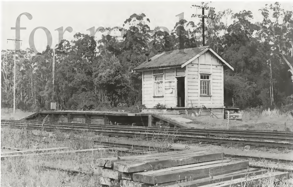
In 1971 decay of many station buildings was well advanced. The timber buildings on Johns River had been demolished, with the lone, concrete-block signal cabin and shortened timber-faced platform remaining.
