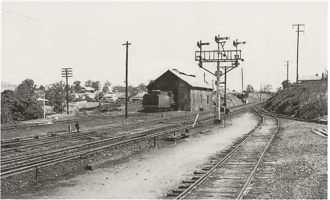
The southern end of Dungog yard. The locomotive shed is in the centre of the photograph, with Standard Goods engine 5350 having a well earned rest. The turntable road is out of view to the left. The track beside the shed is the stock siding, serving the stock race in the middle distance. The triple doll signal (Down Second Home) stands beside the main line, with the tracks in the foreground leading to the goods sidings. I.K. Winney
