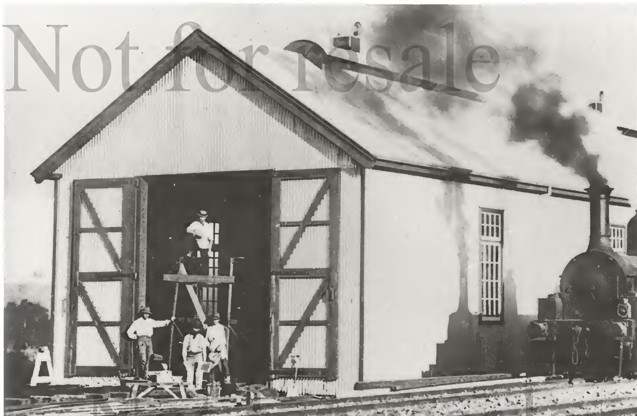
An enlarged view of the front of the Dungog engine shed, with workmen and scaffolding in the doorway of the new building. The heavy swing doors are in position, with roofing and gutters completed, although the smoke chutes are partly finished. SRA Archives
