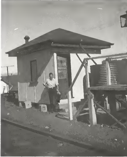
Left: The station office at Tamrookum was of simple fibro-cement construction and contained a desk for the signalman on duty as well as a bed for the use of officers sent there on relief. Signalman Wal Jenkins stands near the office with the staff exchanging platform and oil lamp to the right.
