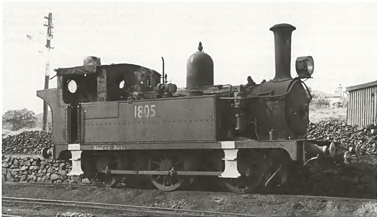
All six of the 18 class 0-6-0 tanks were used at Port Kembla at some time or other but the whole six were not necessarily there simultaneously. 1805 shows the final form of the class having automatic couplers, electric headlight and a steam driven turbo-generator. The photograph was taken beside the coal stack at Reids Hill.
