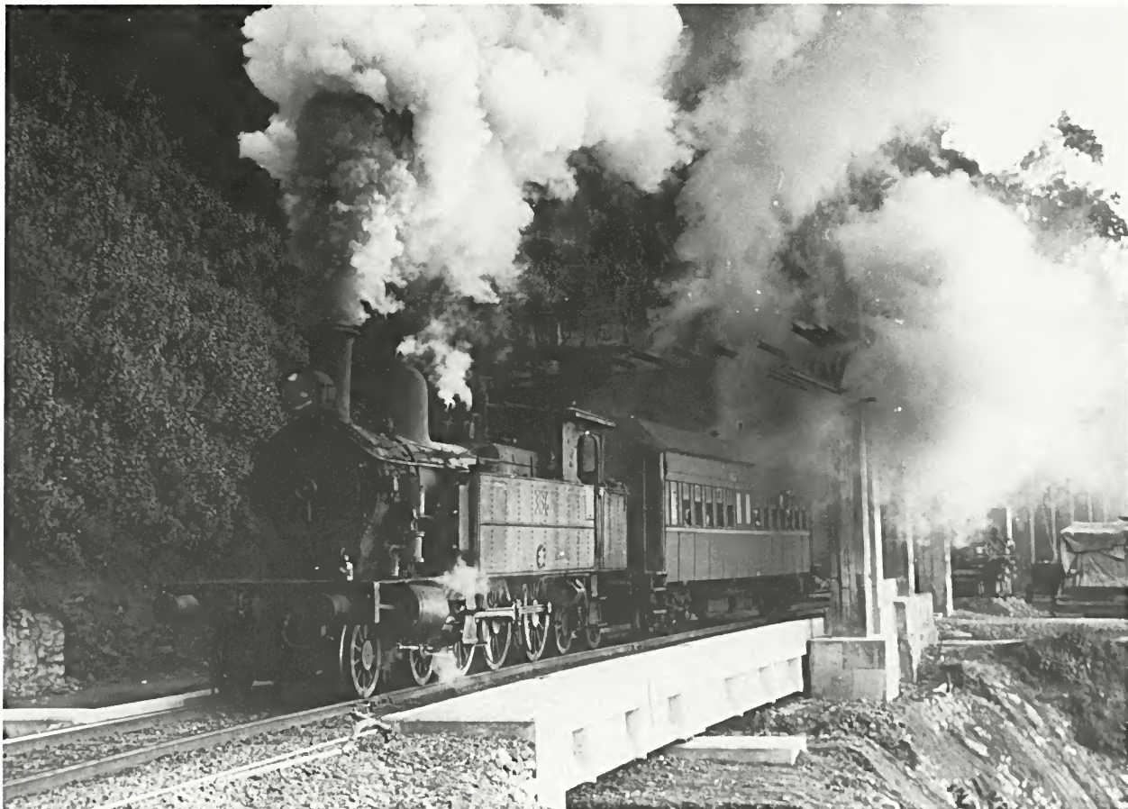
Rock falls and adequate drainage are two problems associated with the Unanderra-Moss Vale line and these can still cause problems during periods of cyclonic rain, when nearby Robertson can have the state's highest rainfall total. Two rock-fall shelters, which have been erroneously called snowsheds, were built to prevent landslips' cascading onto the line. 3136 emerges from one of these shelters as it climbs upgrade from Dombarton.
