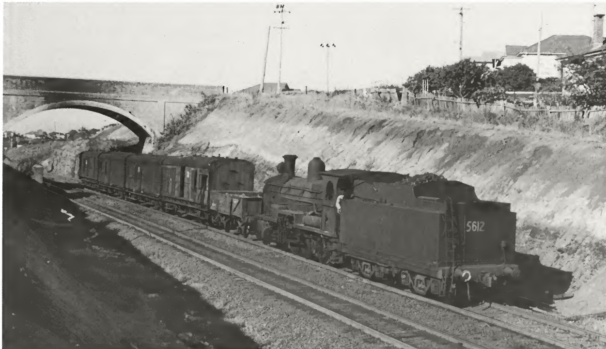
5612 hauls an unusual load consisting of a solitary S truck plus four brakevans (PHG, MHG, MHG, LHG) near Thirroul. This train was a local trip working from Port Kembla. A number of the overbridges, built when the line was duplicated in the 1915-1923 period, had a reinforced concrete arch with brick abutments and walls.
