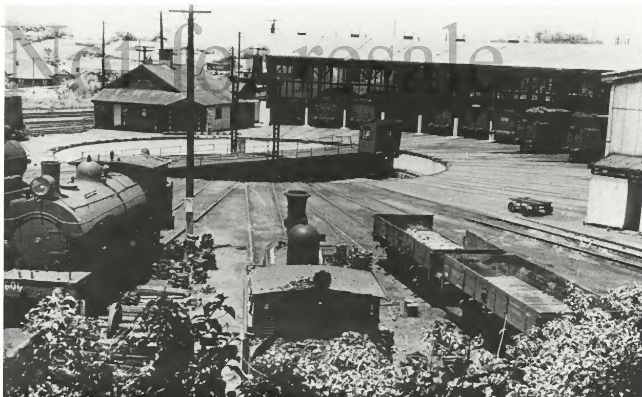
The open tracks radiating from the turntable at Thirroul were put in subsequent to the opening of the depot in 1917, mostly during the 1940s and 1950s. In 1949, the Public Works Department's engines shunting the Port Kembla industrial network came under the wing of the District Locomotive Engineer at Thirroul, where some repairs were now made. Two such engines are shown in the foreground - 2601 and a 20 class. Note the two wooden D wagons used for loco ash and the hand trolley used to transfer stores between the traffic yard and the machine shop.
