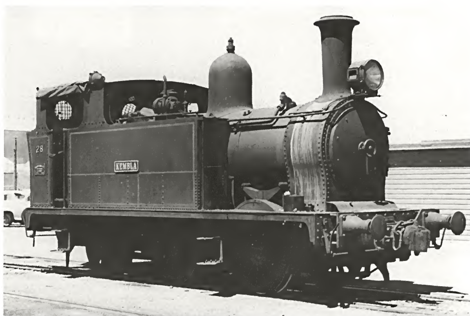
Above: 2604 was the second last of its class to survive in NSW Railways' service and spent some time as a shunter at Port Kembla. It was fitted with automatic couplers and an electric headlight for these duties. The 26s were the only class of engine to retain two single-tone whistles, a relic of pre-1925 practice. The Reids Hill breakdown train is behind the engine. 2604 finished its days at Bathurst, a long-time haunt of the class.
