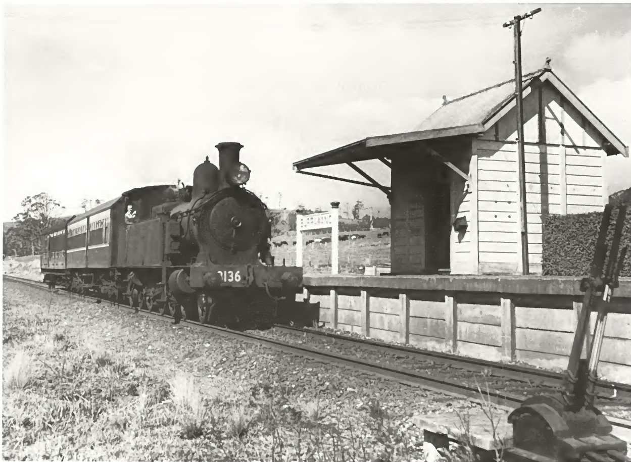
The stations at Burrawang and Calwalla were constructed of pre-cast concrete slabs which require virtually no maintenance except for an occasional coat of paint. 3136 has no passengers to pick up as it passes Burrawang on Saturday, 13 February 1965.
