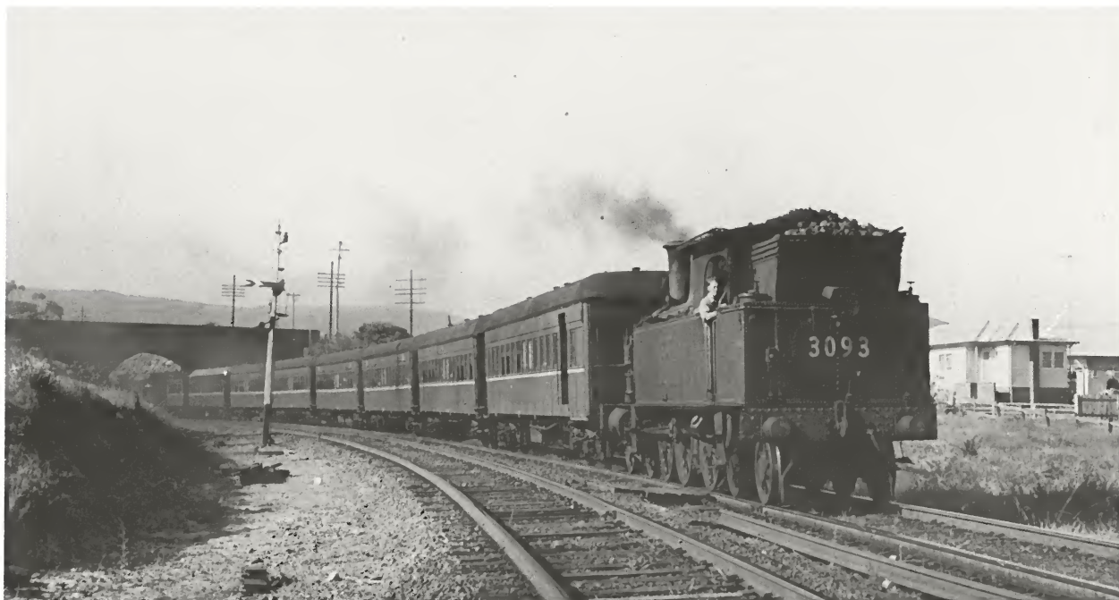
3093 had just shut off steam on a southbound all-stations run approaching Woonona on 5 January 1965. The coal bunker of 3093 has been extended using a railing to increase its capacity. The signal, Bulli's up distant, and the arch bridge beyond were both casualties of the electrification of the line in the mid-1980s.
