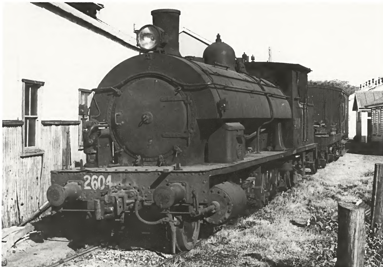
Above: 2604 was the second last of its class to survive in NSW Railways' service and spent some time as a shunter at Port Kembla. It was fitted with automatic couplers and an electric headlight for these duties. The 26s were the only class of engine to retain two single-tone whistles, a relic of pre-1925 practice. The Reids Hill breakdown train is behind the engine. 2604 finished its days at Bathurst, a long-time haunt of the class.
