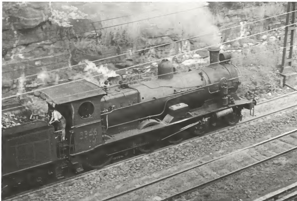
3346 is running light engine to Hornsby through the sandstone cutting just to the west of Cheltenham station. The fireman must be relieved that 3346 does not have a near-full load behind the drawhook as it runs easily up the 1 in 40 grade. Saturday, 2 May 1959.
