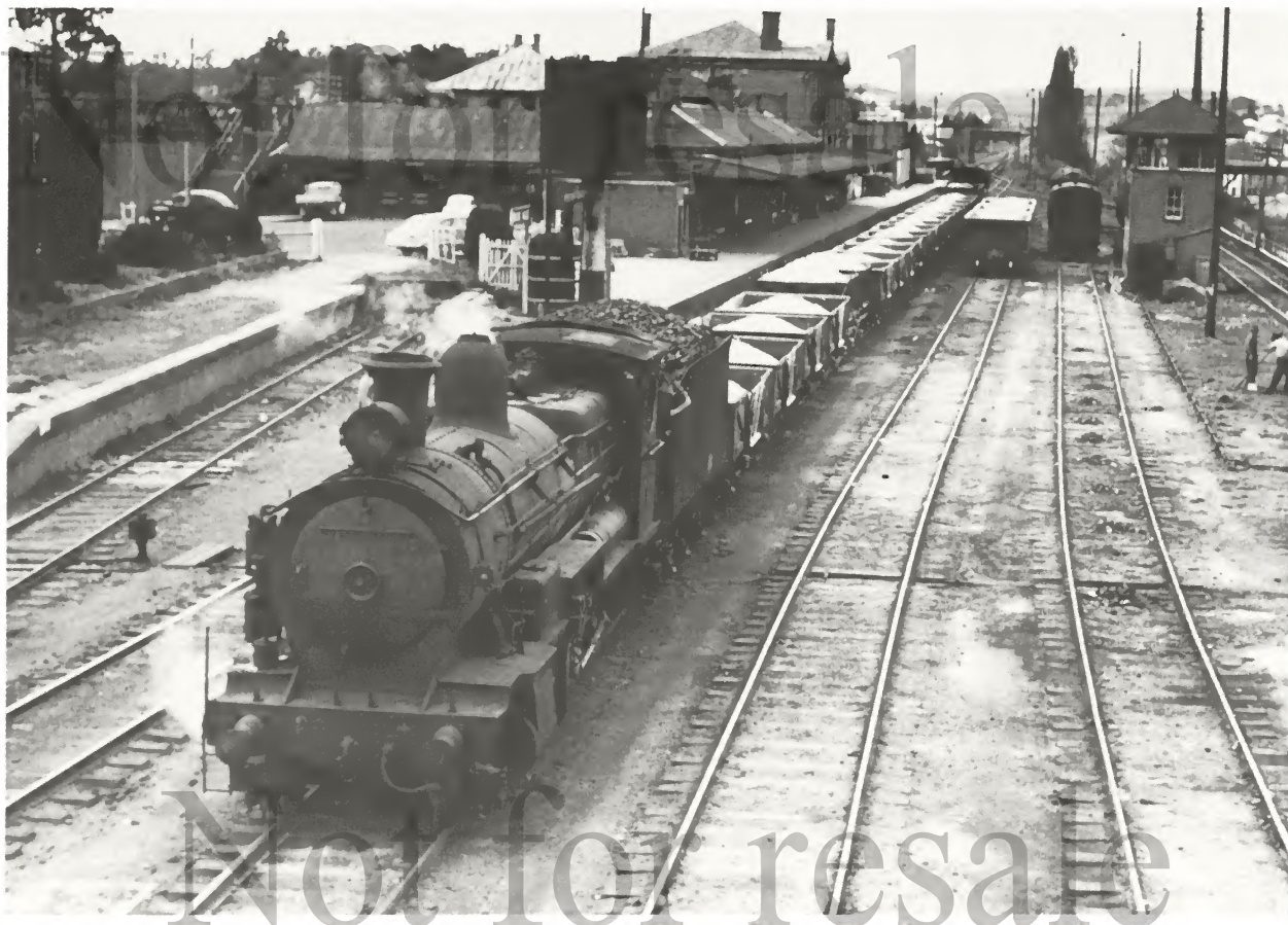
One of the purposes of constructing the Unanderra-Moss Vale line was to bring limestone from the quarry at Marulan South to the steelworks at Port Kembla. In steam days, four-wheeled vehicles such as S wagons and LCH hoppers were used to carry the mineral. 5601 waits at Moss Vale with a limestone train on 17 May 1958.
