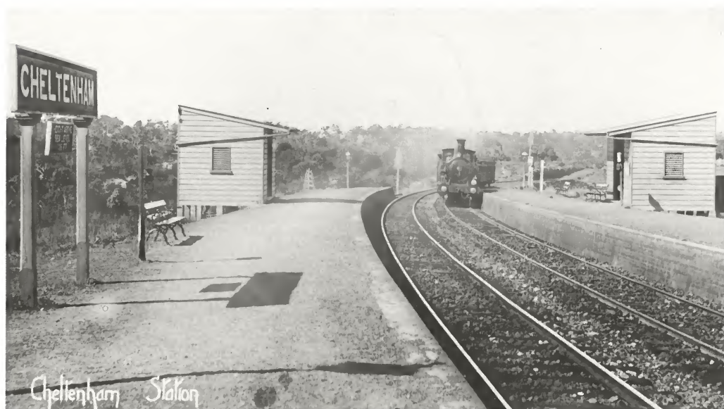
This old post card shows an S class 4-6-4 side tank locomotive at the head of a six car American suburban set, arriving at Cheltenham station with a down suburban passenger train. It is likely the photograph was taken around 1910.
