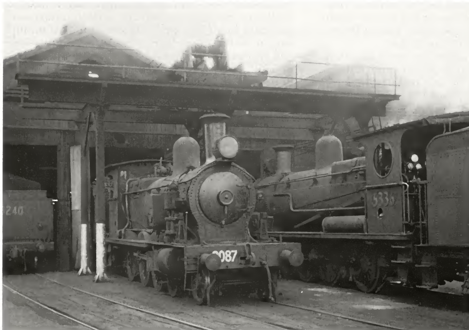
Mudgee engine, saturated 3087 is undergoing repairs at Bathurst loco as it stands outside the eastern end of the large running sheds in company with 5240 and 5336, the latter being one of the few remaining 53s fitted with both specially balanced driving wheels and Wampu tender. Tuesday, 26 December 1961.
