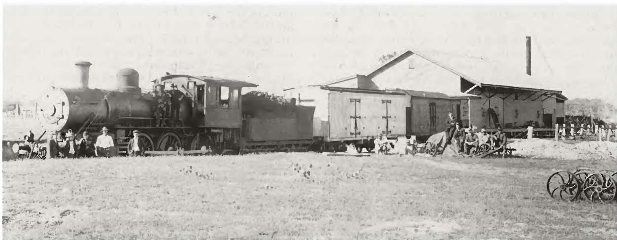
An O class (later 23 class) 4-6-0 passenger locomotive, with cowcatcher and marker lamps, stands at the head of two bogie refrigerator cars on the rabbit freezing siding at Coonabarabran. It is likely the photograph was taken around 1920, the period when the two different refrigerator cars were given the BRC code. In the right foreground are wheels off old horse-drawn wagons used on a light railway during the construction of the line.
