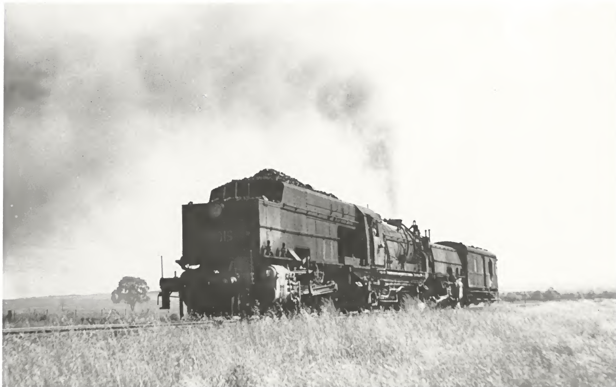
At 9.30am on Thursday, 5 January, 6015 and MHG van charge up the 1 in 60 grade of Bourke Hill, west of Dubbo, and head for the silos at Tomingley West and Wyanga. This train (running as F2) returned later that day with a full load of wheat, being given the train number K9 by Control. Engine 6015 was a light-type Garratt and was permitted to operate on the light lines beyond Dubbo. It was not fitted with dual controls and is actually running 'bunker-first'.
