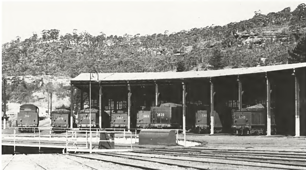
A typical western line-up of engine power in Lithgow loco, October 1962. From left, 3661, 3378, 5135 (saturated), 3087, 5468, 3822, 5400 and 3240 represent the types of locomotives used in the Lithgow-Bathurst-Mudgee area during the period. The roll-call of engines would have been complete, had a 26 class and a 60 class Garratt also been present.
