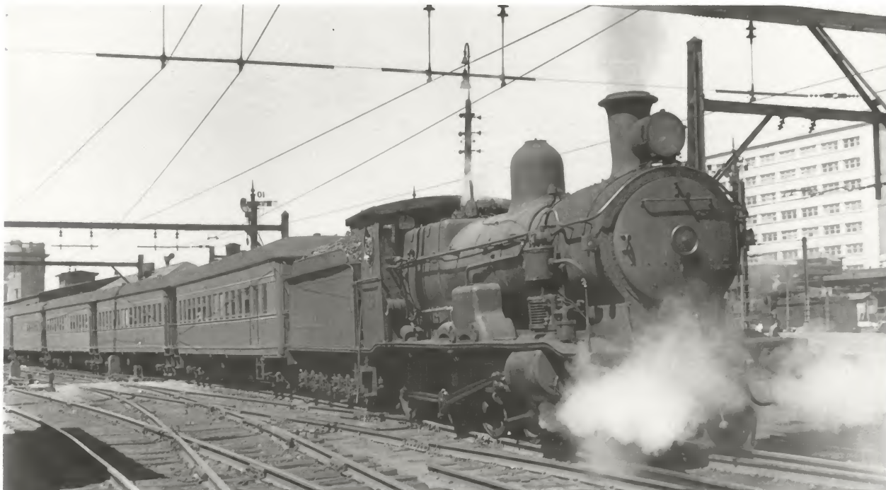
The last in the class, 3391 departs from Sydney station's No.10 platform on Saturday, 26 January 1957 at the head of the 2.30pm passenger to the Illawarra line. The first P class engine to be fitted with superheating, 3391 retained the low frame with curved footplate based on the original P class design. 3391 was unique in many ways. Another 32 class engine, off a recently arrived train, can be seen to the right of 3391.
