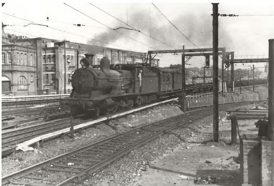
Opposite Page: On Wednesday 24 January 1968, crane locomotives 1034 and 1044 are engaged in lifting sleepers and lengths of rail in Sydney yard. A good deal of co-operation between the drivers of the two locomotives was necessary to ensure a safe and successful lift.
