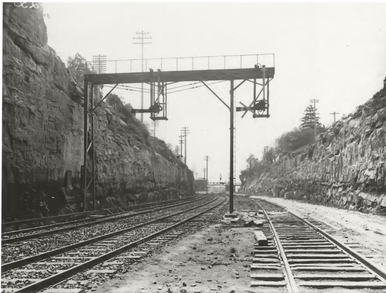
This 1921 photograph shows the completed civil engineering works in the Arncliffe cutting. The two original tracks have been shifted westward and were to form the Illawarra local lines two years later. Sighting and space limitations required that two of the upper quadrant signals be suspended from a gantry. The original signal arms were flat with a pressed-in strengthening rib at their top and bottom edge. There was a supporting bar behind the arm as well.
