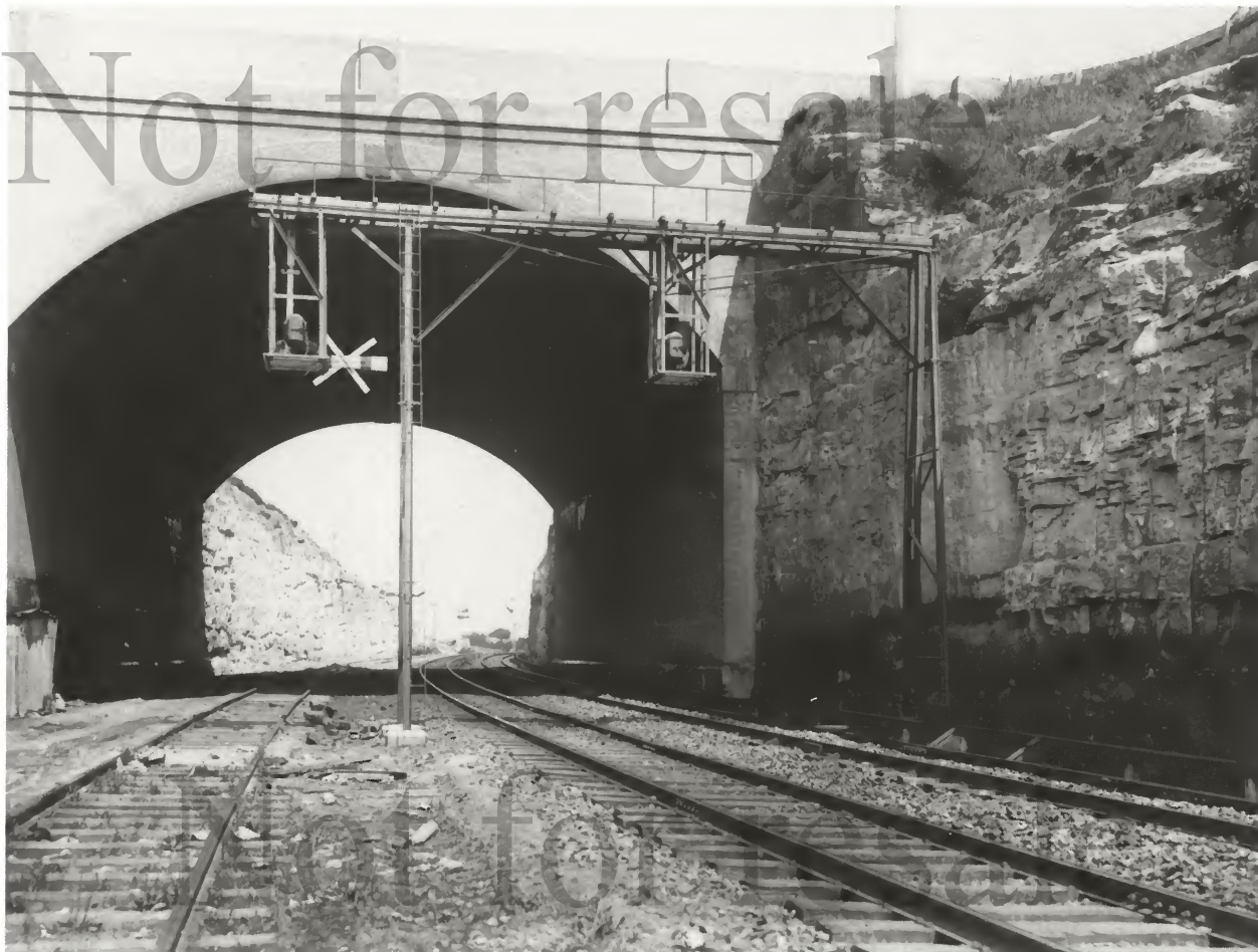
This view is looking at the northern end of the Arncliffe cutting. The cross on the signal arms indicates that it is not in use. The signal applying to the up Illawarra (later the up Illawarra Local line) has been positioned to the right of its expected location to improve its sighting by the train driver.
