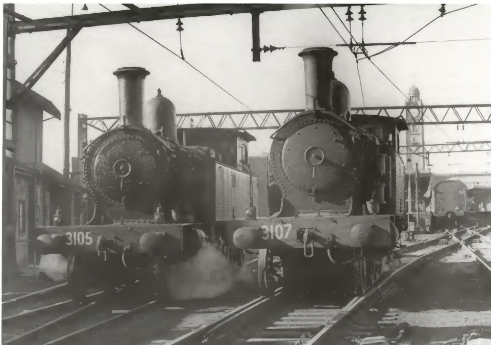
The mainstay of Sydney yard shunting for many years, the 30 class 4-6-4 side tank locomotives are represented here by 3105 and 3107, photographed outside the western car sheds near No.1 platform. The cars formerly used on 'The Fish', SOB set 102, can be seen at right, standing in No.1 platform in the late afternoon. After electrification of the west, SOB102 was reduced to seven cars and ran on Nos 19 and 20 South, the 'Southern Highlands Express'.
