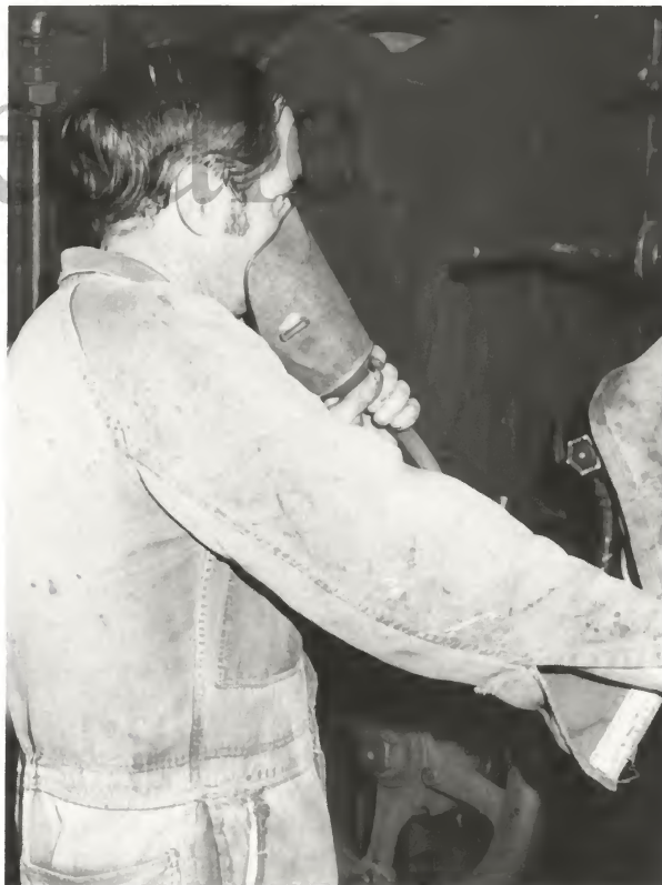
In 1927, respirator equipment was brought into use in Ardglen tunnel, to assist crews working in the smoky atmosphere. Masks, hoods and gloves were available. Here, the driver makes use of the mask connected to the engine air supply. R.D. Love
