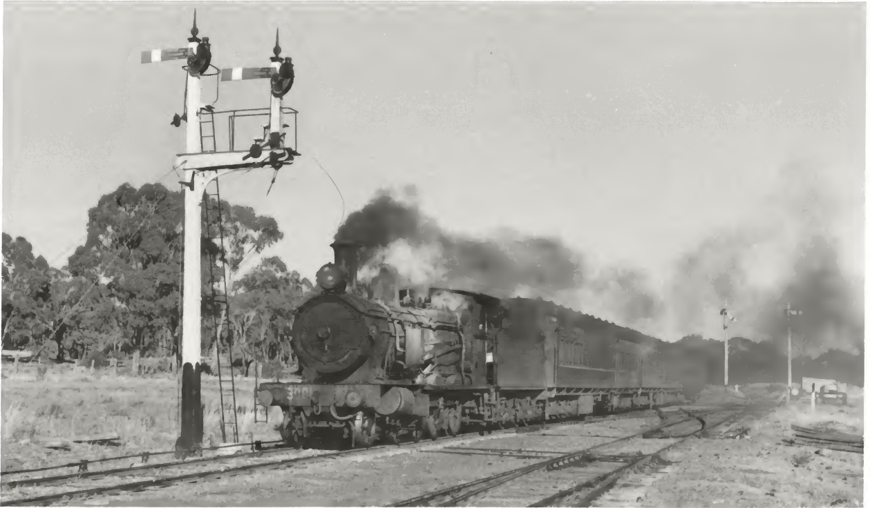
On 3 June 1967, 3001 leads No.63 down Mudgee Mail into Merrygoen yard, two twelve-wheelers and a van making up the load on this day. The scissors crossover and the up starting signals (mounted on a wooden post) were later replaced by less interesting installations.
