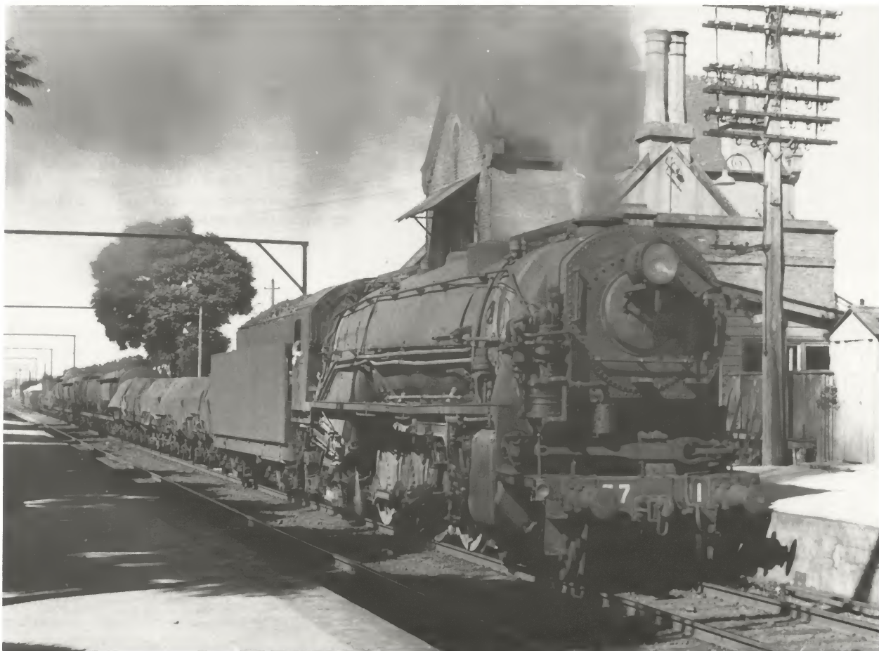
On Tuesday, 30 August 1955, a westbound goods train with 5711 in the lead charges through Emu Plains station at the foot of the climb up the Blue Mountains. Further up the mountains, at Valley Heights, 5711 will probably receive assistance from a Standard Goods locomotive over the almost continuous 20 mile long stretch of 1 in 33 grade to Katoomba, taking water at Lawson.
