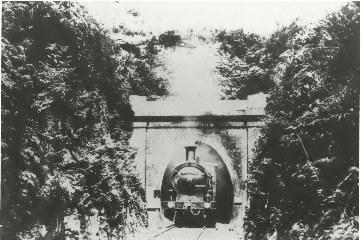
A tight fit. One of the old, single line tunnels on the original route of the Illawarra line, between Waterfall and Stanwell Park, c.1900. These tunnels were notorious for problems with heat, smoke and fumes affecting both crews and passengers alike. A T (later 50) class engine emerges from the portal, showing the lack of free space when a train occupies these single line bores.
