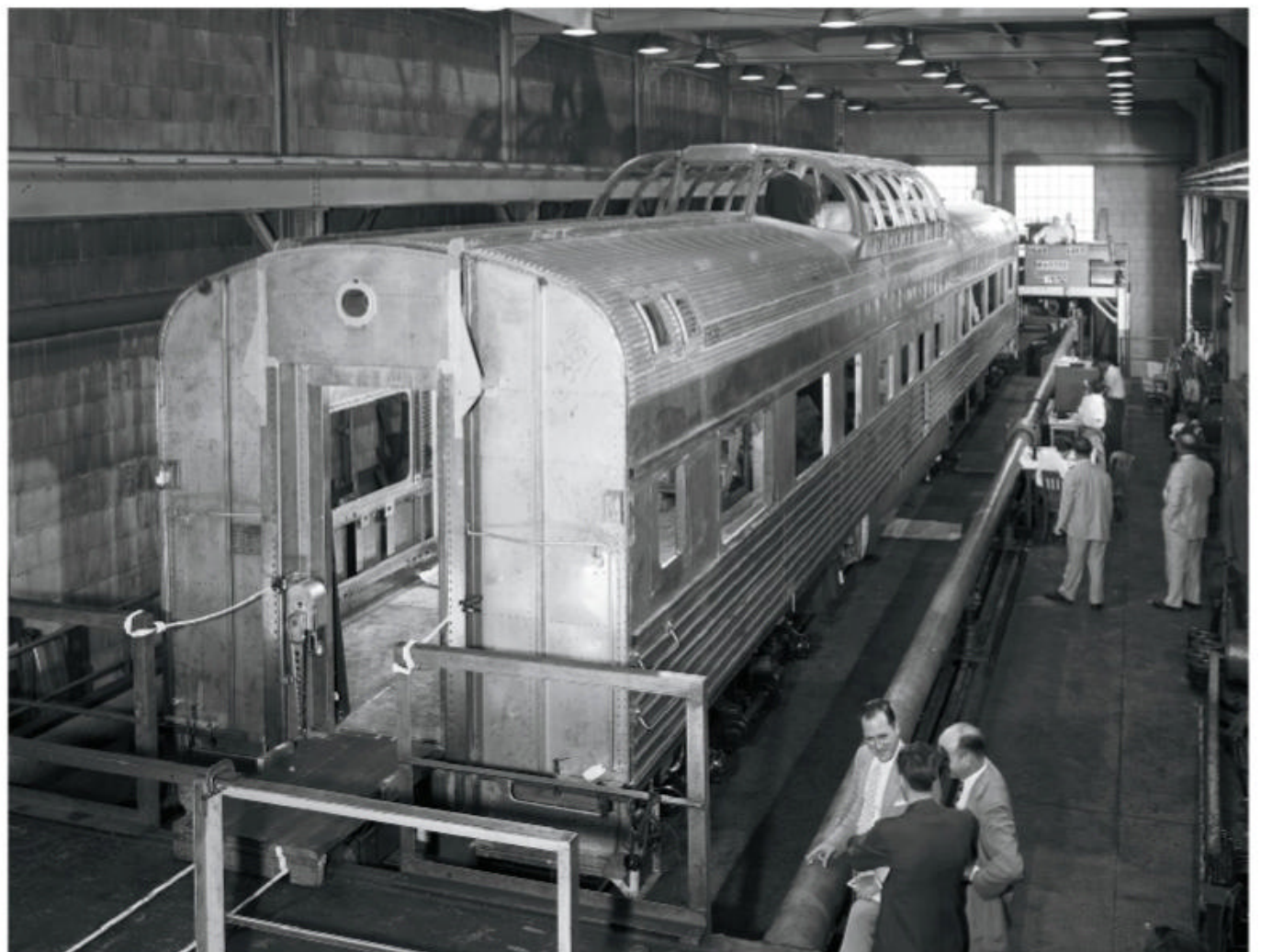
Budd and CP personnel inspect a partially completed Skyline dome car for the Canadian in mid-1954. The car is on Red Lion's compression test plant. Railroad Museum of Pennsylvania
