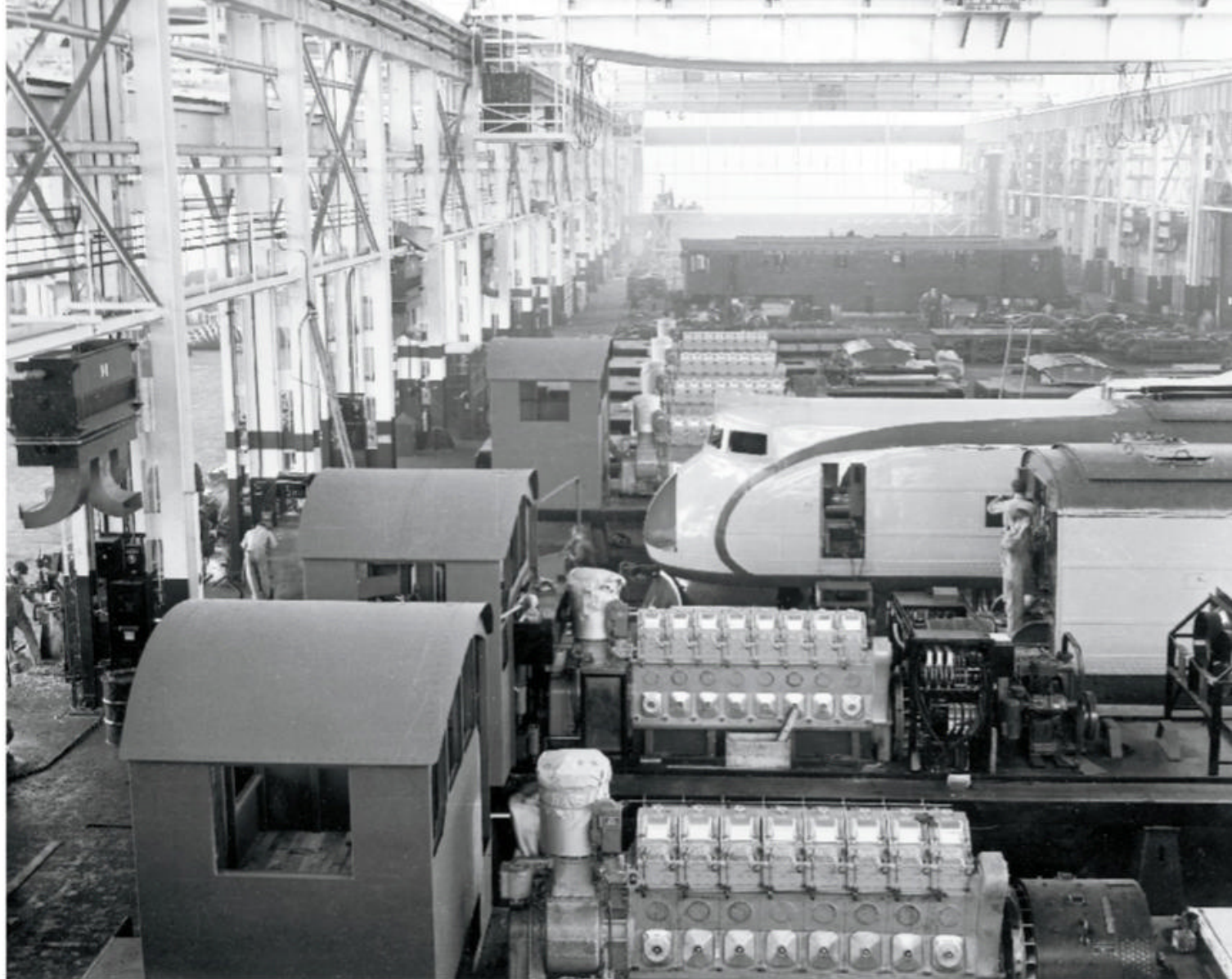
Several switchers, the power units for Union Pacific's M-10002 streamliner, and B&O box-cab passenger unit No. 50 occupy the shop floor of EMC's new plant at La Grange, Ill., in 1936. Electro-Motive
