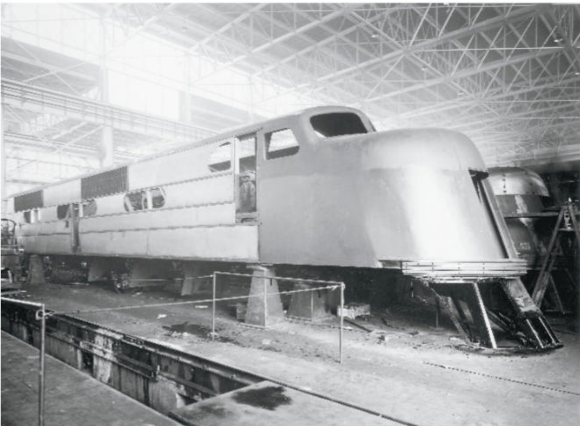
EMC followed up the homely box-cabs with the mechanically similar E series, styled by GM's Leland Knickerbocker. At left, the first example, B&O EA No. 51, takes shape at La Grange. At right, sister 55 leads a train through Philadelphia in the mid-1940s. Left, Electro-Motive; right, Frank and Todd Novak collection
