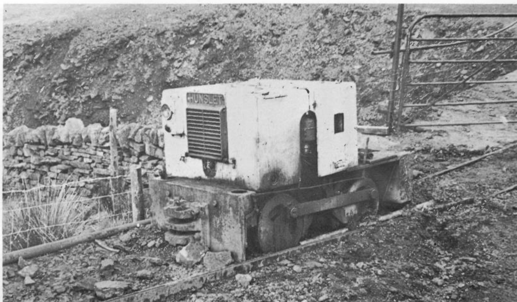
INDUSTRIAL DIESELS — (1) AYLE COLLIERY CO LTD. AYLE EAST DRIFT. ALSTON, CUMBERLAND. Hunslet 'Tiny Tim' 2 ton mining diesel with 15H.P. Enfield engine. One of the smallest industrial locos ever built. No. 4991 (1956) sits outside the adit, right on the county boundary between Cumberland and Northumberland. [2ft gauge] (Pete Nicholson)
