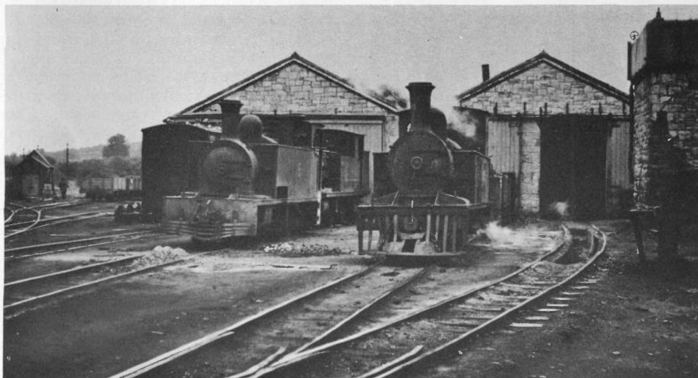
BALLINAMORE SHED (C.I.E.) IN 1954. LOCOS No.8, 4-4-0T (Stephenson 2619 of 1905), No.5, 2-6-2T (Hunslet 555 of 1892) ex T.&D. & another, 2-4-2T (Nielson Reid of 1899) ex C.B.&P. (Courtesy Photomatic Ltd.)
