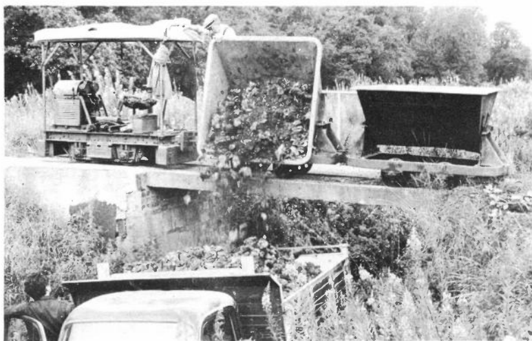
NEWSTEAD WORKS 9/8/71 Rare 4wheel Petrol engined Lister 26288 of 1944 discharging skip contents into road vehicle at the tip. (Sydney Leleux)
