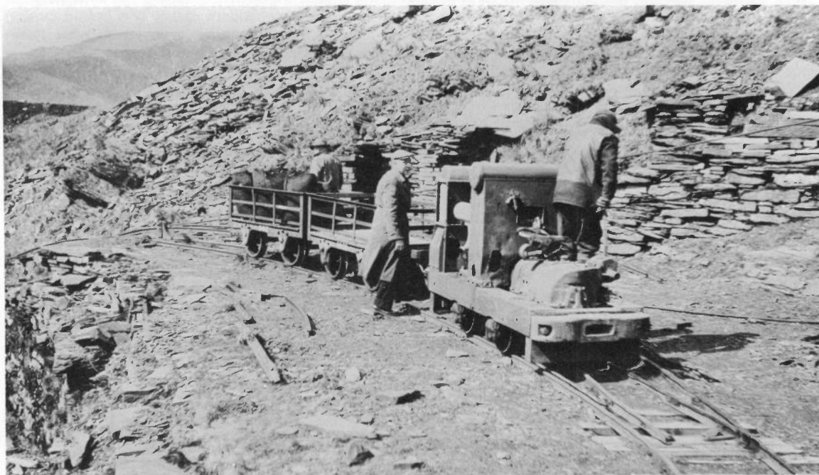
Maenofferen, April 1970. Unidentified Ruston (probably 18/21h.p. RH174542) cautiously shunts two wagons up to the incline head, an operation requiring some care since on one occasion, about 1965, RH175138 ran away down the incline and was damaged so badly that it had to be scrapped. (Chris Down)
