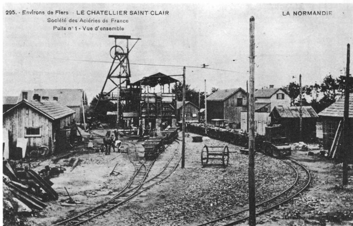
A general view of the Halouze mine showing the 630mm gauge layout. One of the Thomson-Houston locos stands on the right with a train of tip wagons. (collection P. Pontremoli)
