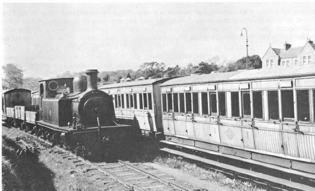
At the same location in May 1950, Hudswell Clarke 4-6-2T 15 is arriving with a goods train. Carriage B12 on the right, a bogie 1st/3rd built for the Letterkenny & Burtonport Extension Railway in 1904, had by then lost its acetylene lighting and this, together with a reduction of the weeds on the track, are the only significant changes in thirteen years. (R.C. Riley)
