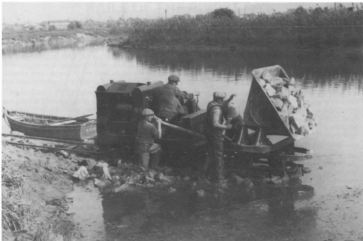
Tipping one of the first loads of stone at Lower Parting, Gloucester, clearly showing the two men with poles holding down the wagon frame. 10th May 1939.
