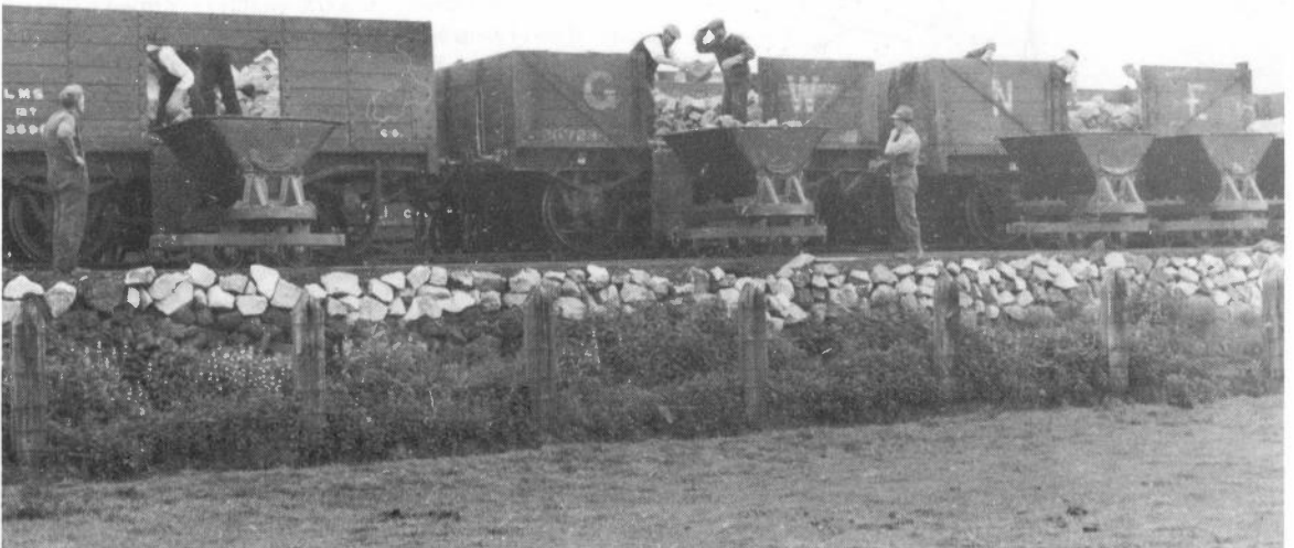
Transferring stone by hand at the G.W.R. Docks Branch sidings. Note the variety of main line wagons, and the number of men (nine) employed. 10th May 1939.
