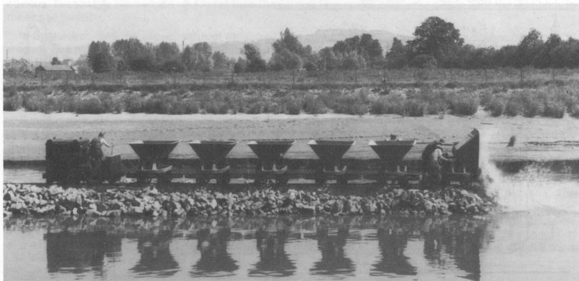
The training wall at Lower Parting nearing completion on 5th June 1939.
