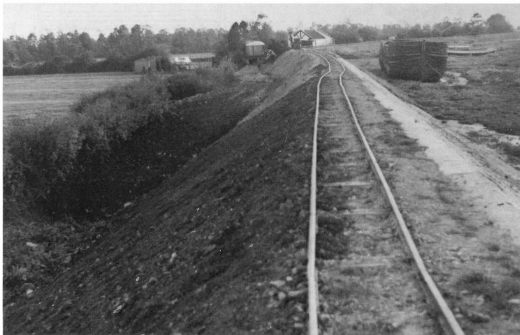
Shepperdine Sea Wall Improvement Scheme on 25th October, 1956, showing quarry overburden being tipped to reinforce the rear of the sea wall. Note how the track was slewed as tipping progressed, and the dragline loading skips in the background.
