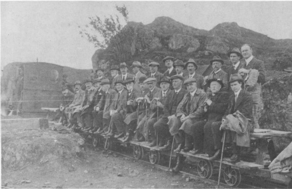
A train standing on the "main line" behind the winding house at the incline head, ready to leave for Llyn Cowlyd. One rail of the line to the incline can be seen in the left hand corner. The five vehicles are steel tip wagon frames fitted with temporary seats.
