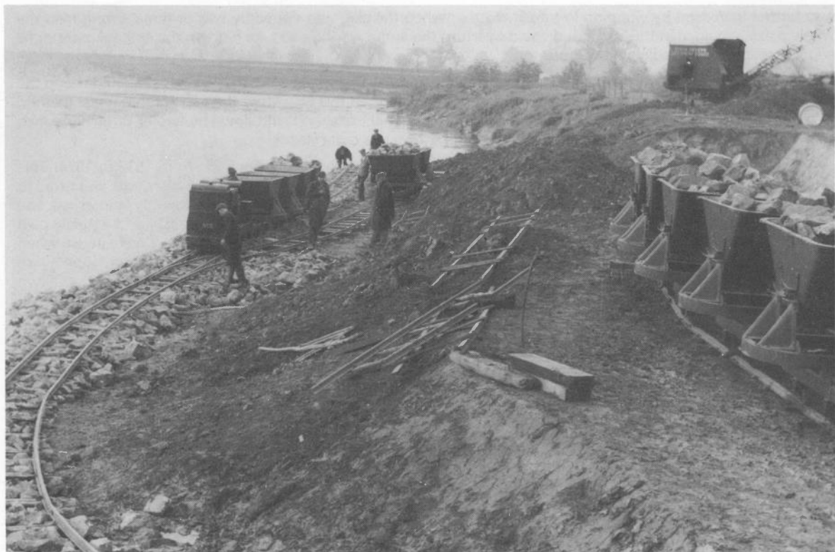
Works progressing at Lower Parting, with a second siding installed. Note that eight men are employed here, and the almost new skips on the right. 17th May 1939.
