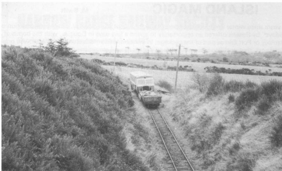
Culvert repairs near the old Castletown road bridge occupied railcar 20 and a bogie flat loaded with building materials. (A.D. Swift)
