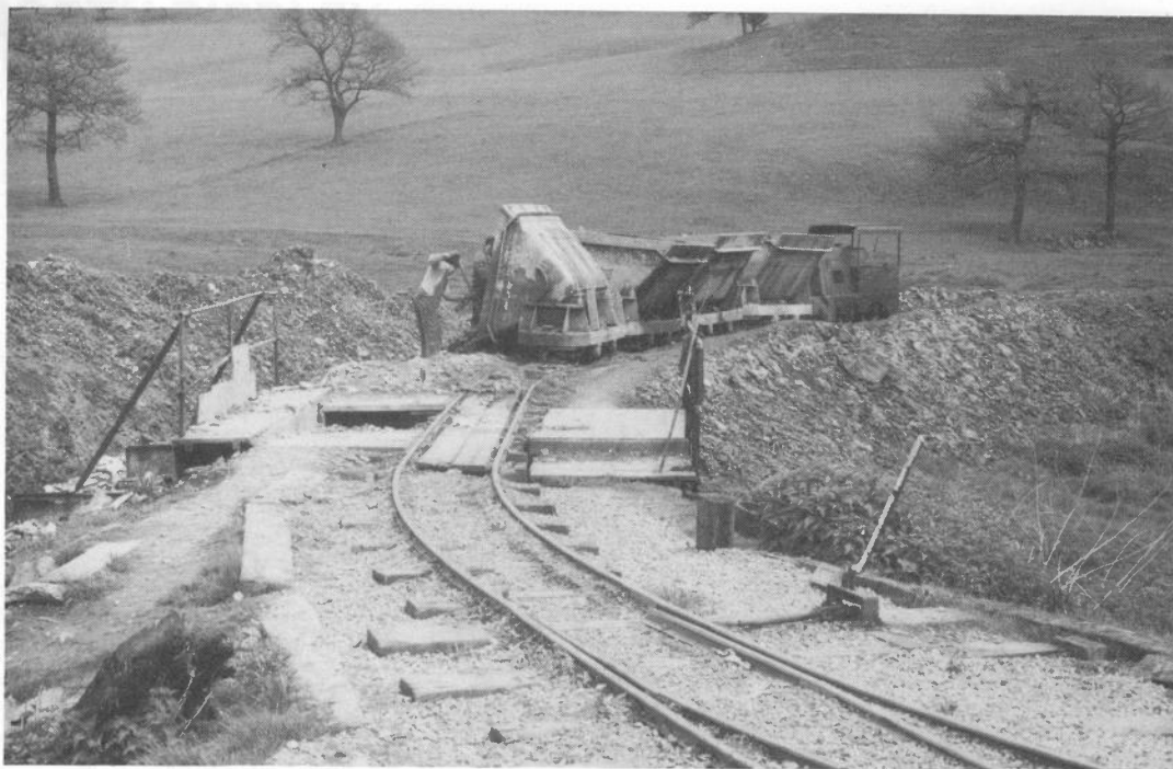
Unloading filter cake from the Firth Bros. skips onto the tip. April 1979.
