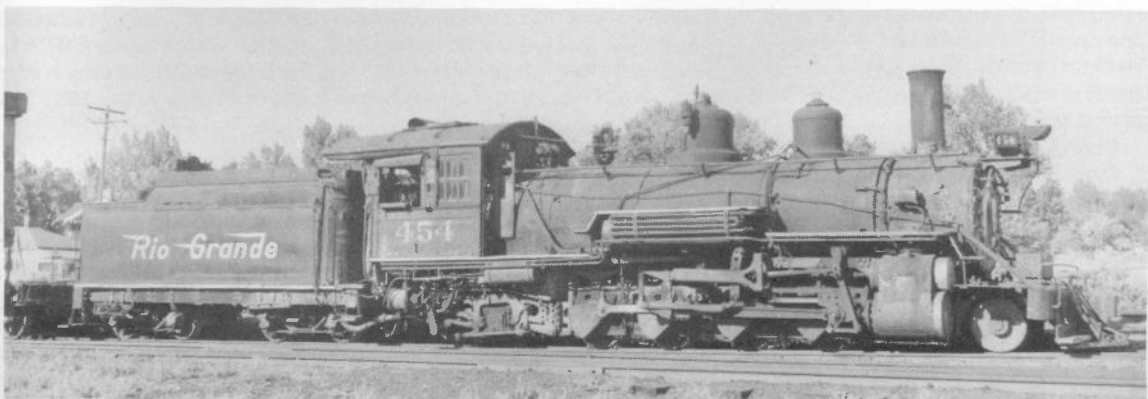
D. & R.G.W. R.R. 2-8-2 Class K.27 No. 454 in final superheated form with piston valves and Walschaerts valve gear. Seen at Montrose 16.8.53. In this form Nos. 453, 463 and 464 ended their days at Durango switchers, but this loco was scrapped at Montrose in 11. 1953.
