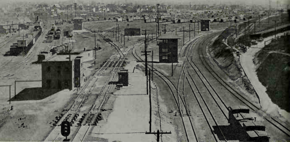
The great eastbound N.&W. classification yard at Roanoke, Va., showing: (lower left) hump signal, retarders, master scales and scalehouse, retarder control towers, floodlight towers; (far left) ice dock; (outside right) eastward running track, thence cab tracks. Courtesy Norfolk & Western Railroad.
