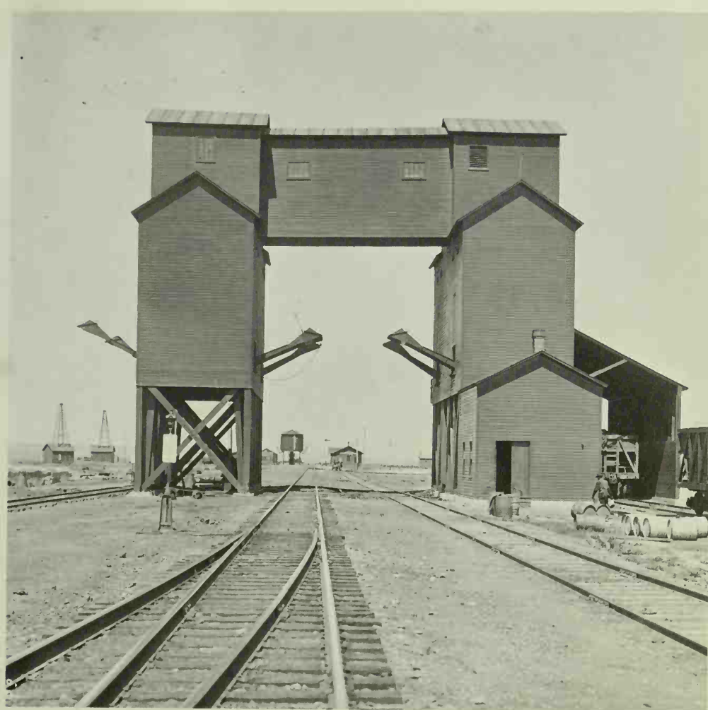
The coal tipple at Wamsutta, Wyoming, and the water plug at Sidney, Nebraska, with its lantern to show its position at night were the familiar facilities for fueling the iron horse at the turn of the century. (Two Photos: Wyoming State Historical Department.)
