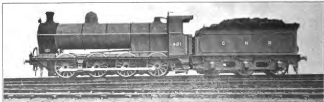
Fig. 5035. Eight-Coupled Goods Locomotive. Great Northern Railway. Cylinders 19 1/2 in. x 26 in.; Working Steam Pressure 175 lbs. per sq. in.; Total Heating Surface 1,138.84 sq. ft.; Diameter of Drivers 56 in.; Weight on Drivers 122,340 lbs.; Total Weight 122,340 lbs.
