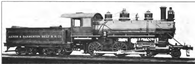
Fig. 34. Mogul (2-6-0) Locomotive. Built by the Baldwin Locomotive Works for the Akron & Barberton Belt Railroad. Cylinders 20 in. x 24 in., Working Steam Pressure 180 lbs. per sq. in., Heating Surface 1,829.3 sq. ft., Diameter of Drivers 56 in., Weight on Drivers 115,000 lbs., Total Weight 132,000 lbs.
