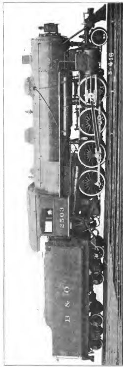
Fig. 43. Consolidation (2-8-0) Locomotive. Built by the American Locomotive Co. for the Baltimore & Ohio. Cylinders 22 in. x 30 in., Working Steam Pressure 205 lbs. per sq. in., Heating Surface 2,792.2 sq. ft., Diameter of Drivers 60 in., Weight on Drivers 185,000 lbs., Total Weight 206,500 lbs.
