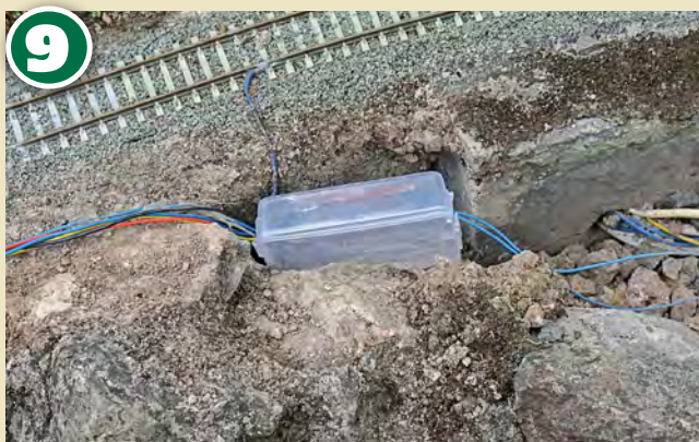
At the top of the viaduct the lighting circuit has been broken into, a junction box inserted and the cable for the harbour lighting run along the viaduct. The space around the junction box will be filled with gravel and capped over with a weak peat:mortar mix.
