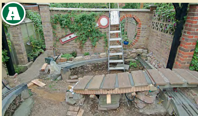
2005 and construction of the final trackbed, bottom pond and bridge to the garden extension is under way. For years this area had been a temporary section on timber.
