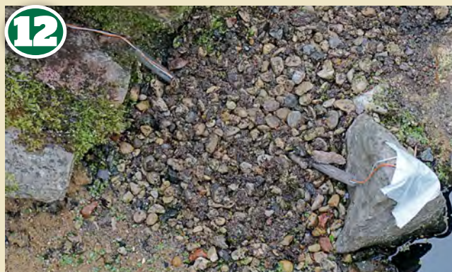
The cable for the harbour light runs through a protective tube where it will be below water level. The ends will be covered with mortar.
