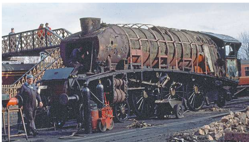
Union of South Africa in the process of being dismantled for overhaul at Bridgnorth on the Severn Valley Railway on March 5, 1989.
