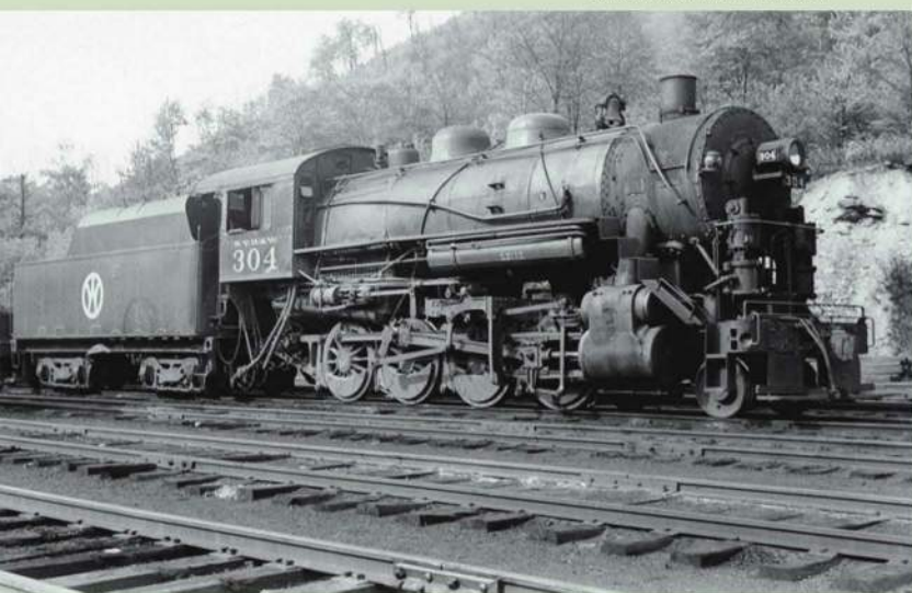
This New York, Ontario & Western steam locomotive was a Consolidation-type with a 2-8-0 wheel arrangement. The railroad was the first major railroad to suffer complete abandonment in the post-World War II era, with its last train operating in 1957.
