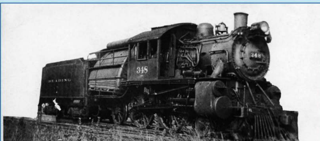
READING COMPANY NO. 348 4-4-2 PASS. LOCO.-ATLANTIC TYPE
