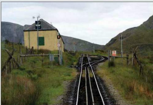
Below: The latest installation at Hebron seen from the train on 11 June 2009. There are two wind turbines and solar panels, and the signals use LEDs. On the uphill journey the top points are changed by the guard using a remote control, the driver having that responsibility on the way down.
