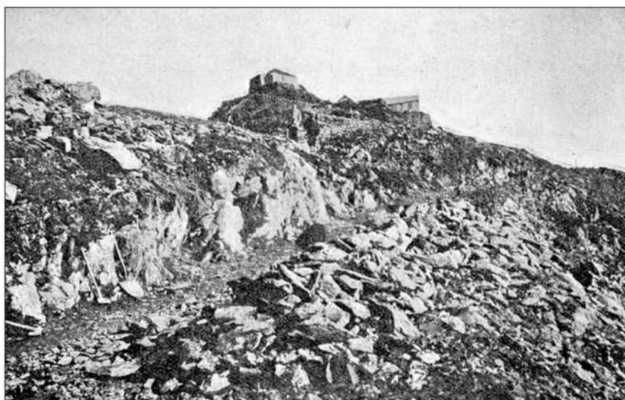
Top: The cutting below Halfway, ready for track laying. At about 20ft, it is the deepest on the line. Clinton Holme/Author's collection
