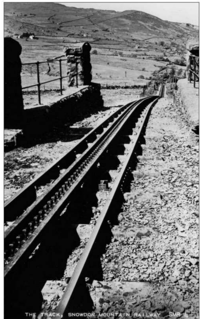
Below The track looking downhill near Hebron. One of the iron stays set in concrete to stop the track creeping down the mountain can be seen between the rack and the right-hand bearing rail. Commercial postcard/Author's collection
