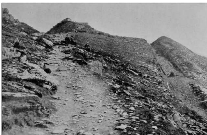
Top: The cutting below Halfway, ready for track laying. At about 20ft, it is the deepest on the line. Clinton Holme/Author's collection
