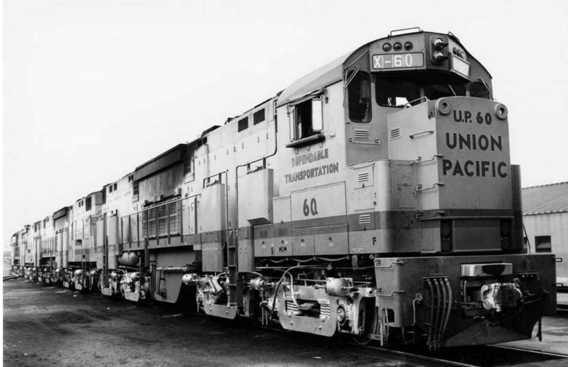
All three locomotive manufacturers built massive double-diesels for Union Pacific in the 1960s. Alco's effort was this A-B-A set of C-855s, each unit riding on four pairs of B trucks and powered by dual 16-251 engines. They were 86 feet long, weighed 528,000 pounds, and were slightly taller than typical Century models. Jay Williams collection
