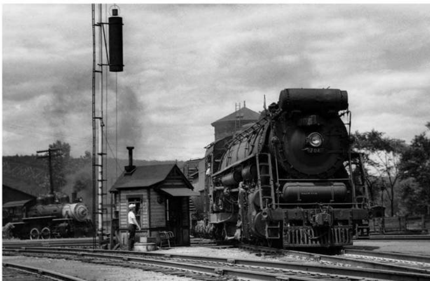
In 1928, Alco Schenectady delivered 10 2-10-4 Texas types to the Central Vermont Railway. The CV had recently entered the Canadian National fold and had been completely rebuilt north of Brattleboro following Vermont's great flood of November 1927. The CV's 2-10-4s shared qualities with big CN designs. They were the largest locomotives in New England and were not allowed south of Brattleboro. On June 21, 1952, 2-10-4 No. 708 leads a southward freight across the Rutland Railroad diamonds at Bellows Falls. Jim Shaughnessy
