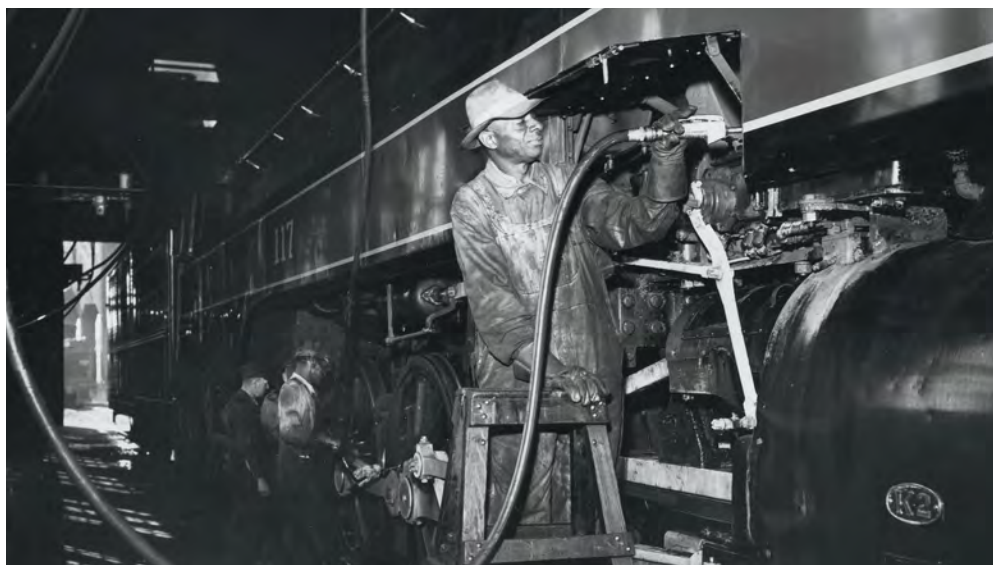
2:50 Inside the lubritorium, lubricators are filled; rods and valve gear greased; and stoker, headlight, feedwater heater, injectors, and air pumps checked.
