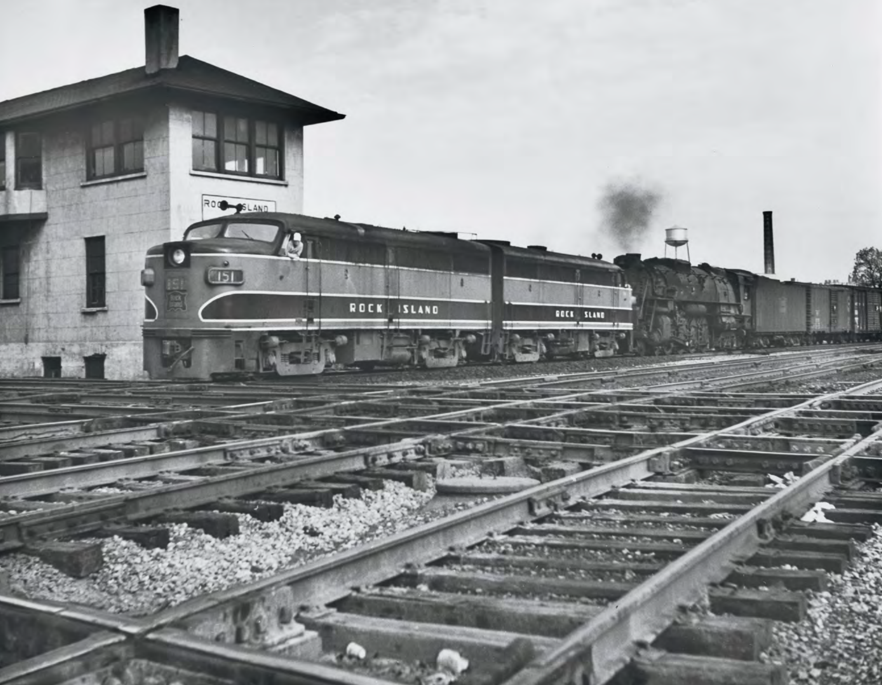
The fireman on FA 151 leading "Rocket Freight" No. 91 leans out as the Alco hits the GM&O diamonds. Behind sister FA 145 is 4-8-4 No. 5119. EMD re-powered RI's 8 Alco A-B-A trios with 567s in 1954-57, and they were renumbered 128-143.
