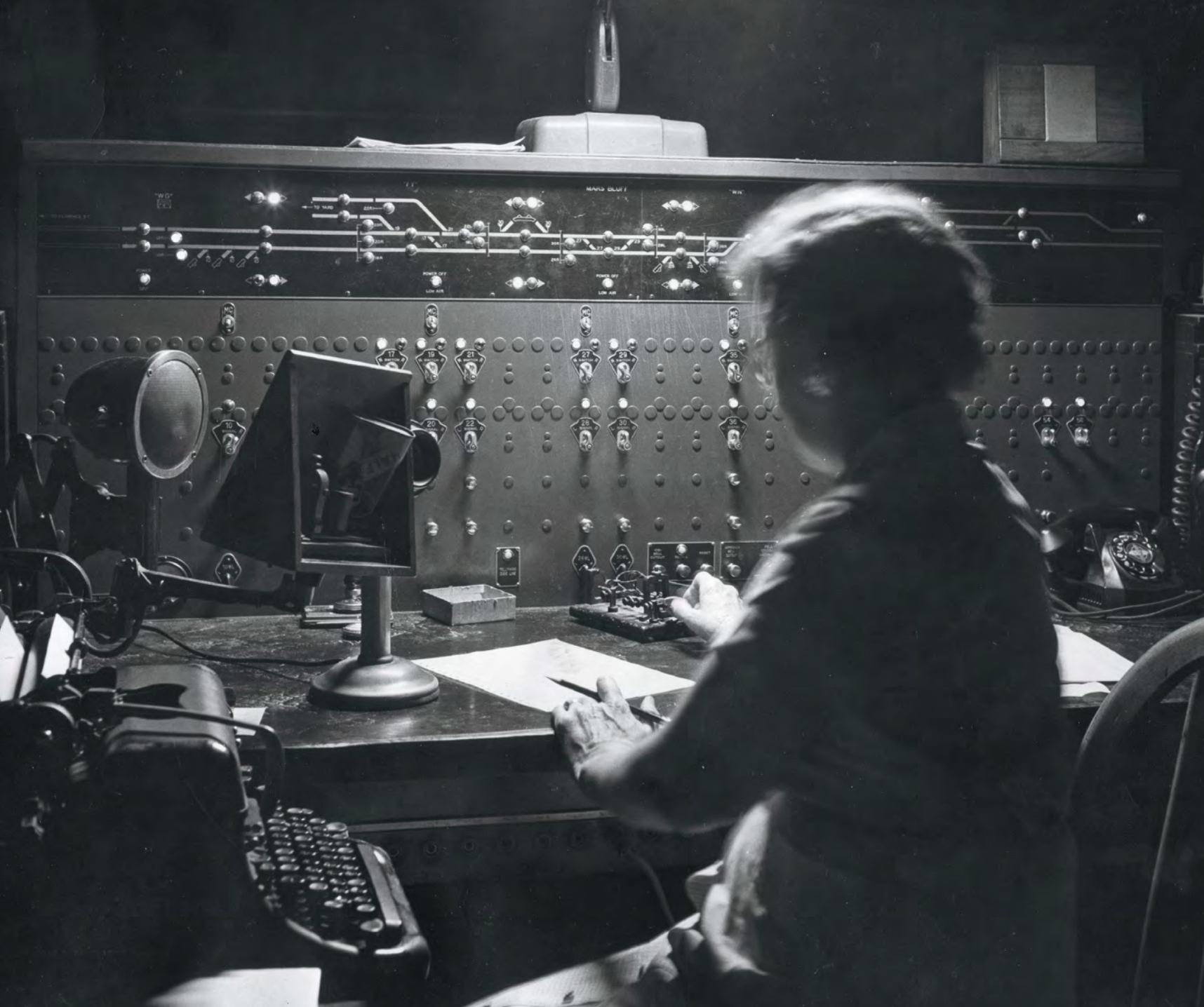
Operator Mrs. L. H. McBratney keeps the Coast Line streamliners on the move during the night trick at WG Tower in Florence. The C.T.C. console here controls the 12.6 miles of main line from Florence north to Pee Dee, S.C.
