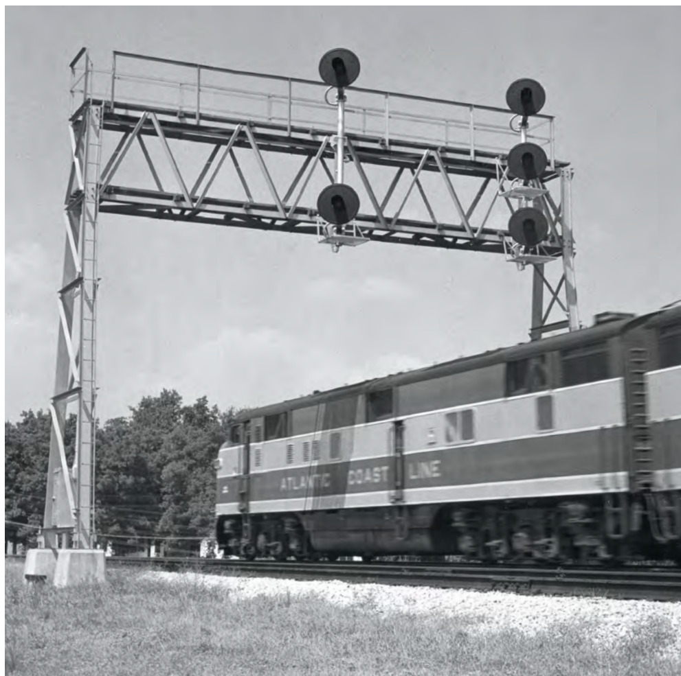
C.T.C. signals, angled for better visibility on a left-hand curve, preside over train 76, the northbound Havana Special , as it slows for its Charleston, S.C., station stop.
