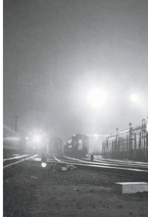
A blue lantern by the pilot of E7 No. 539, heading up the East Coast Champion at Florence, indicates the train is not to be moved during its 5-minute servicing stop.
