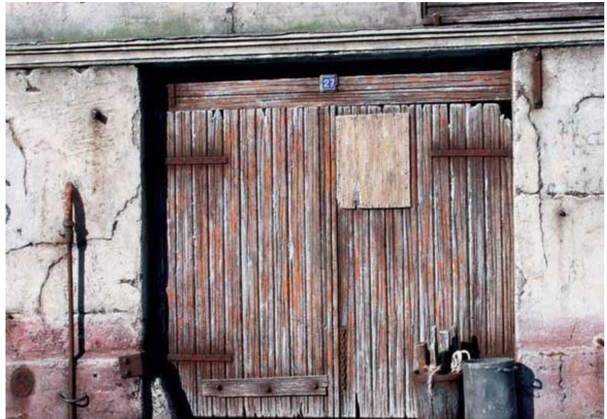
Planked wooden double doors made by the author in one of his buildings. The typically French blue and white enamelled house number plate adds the finishing touch.
