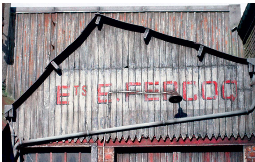
Other results of faded and weathered paintwork on wood with variations in the planks, different shades of colour, rotten planks and so on...
