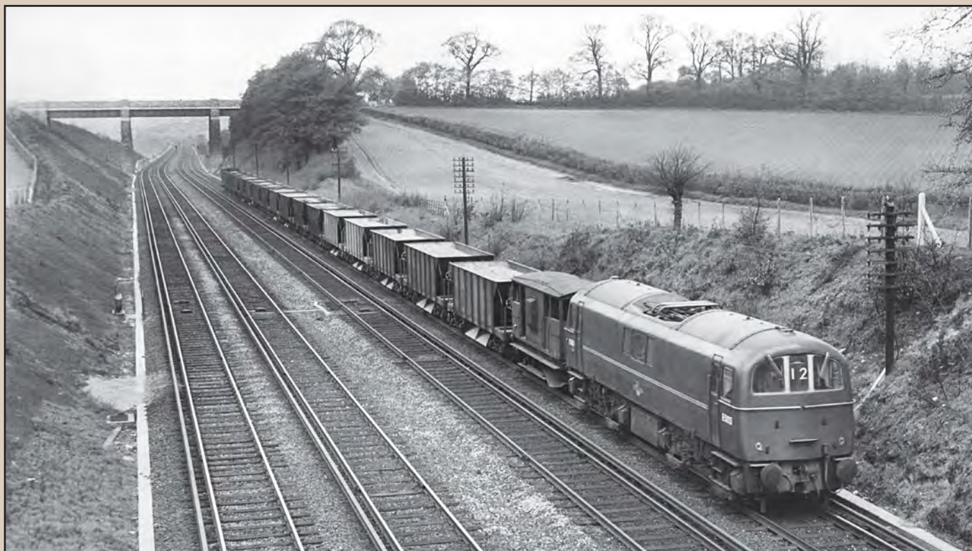
Below: On 27 April 1960, No. E5013 powered an 'express freight' test hauling 16 loaded wagons carrying 1,010 tons of ballast from Dover to London, to gauge performance of the fleet. The train is seen near Swanley. Derek Cross
