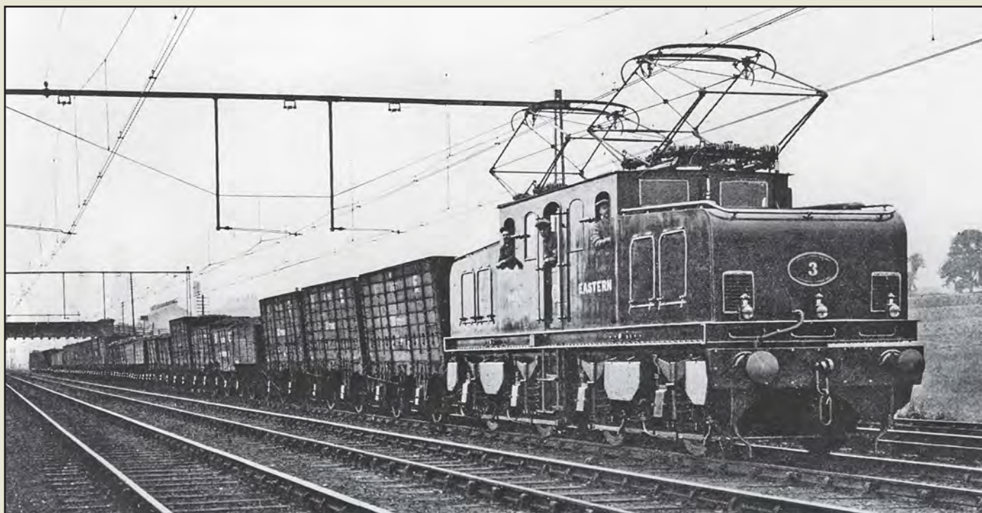
Below: The pioneer of the ten strong Bo-Bo freight fleet No. NER3 is seen soon after introduction in 1916 carrying out performance and riding tests with a long rake of wooden bodied coal and mineral wagons. Information on the reverse of the original photograph, indicates the train was bound for Newport with driver Jefferson at the controls. It also quotes that each train operated with a footplate crew of three.
