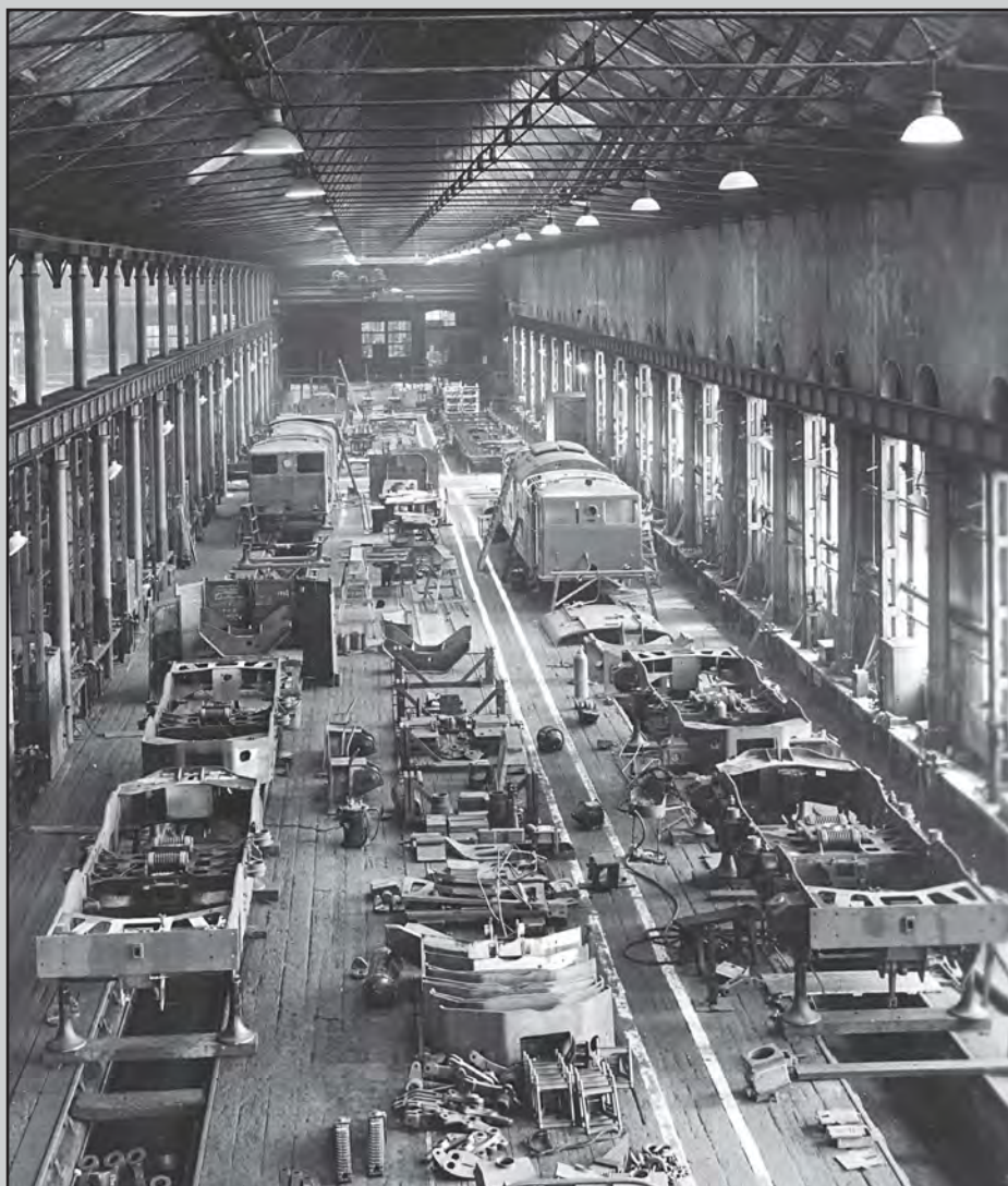
Left: Fleet production of the LNER Bo-Bo 1,500V dc locos commenced at Gorton Works in the new year of 1950, with some seven locos seen in various stages of assembly in mid-March. Several of the early built locos were transferred by rail to Dukinfield Works in a near complete condition for the installation of electrical equipment and some static testing, before returning to Gorton for completion and painting. This view shows five locos under various stages of construction with two pairs of bogies under assembly in the foreground. CJM-Collection
