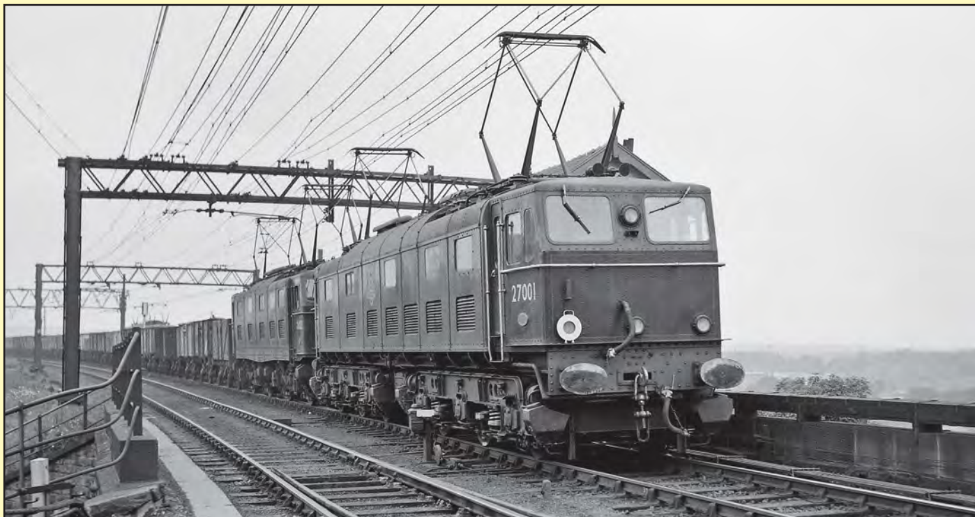
Above: Images of Class EM2 and EM1 locos operating together are very rare, the two classes could not operate in multiple and thus had to work in tandem, with a crew on each loco, unless the second loco was being hauled 'dead in train'. With both locos having their pantographs raised, obviously both locos were staffed in this image of No. 27001 and 26023 powering a freight train in March 1954 as a running in turn for the then new EM2.
