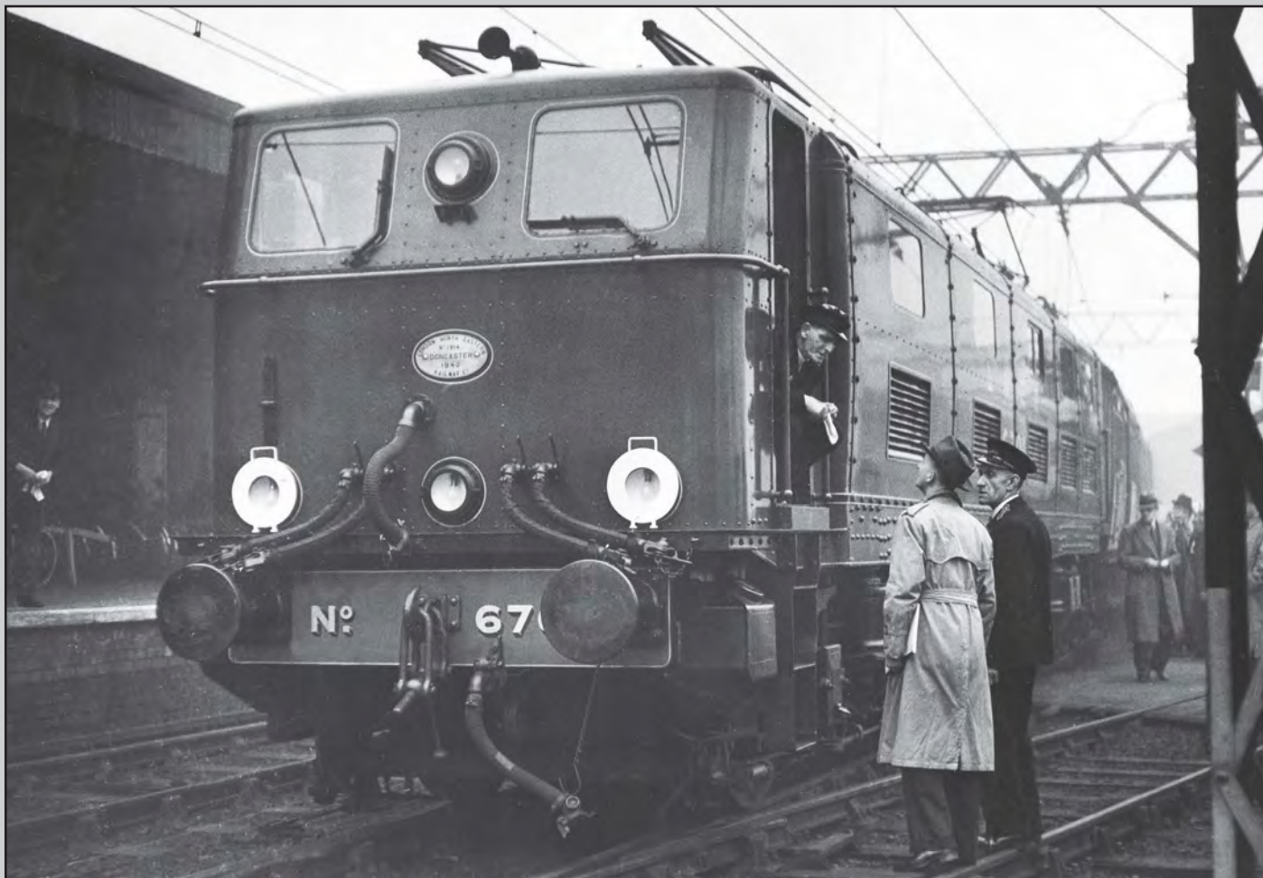
Above: To enable testing of LNER 6701 the loco was hauled over the Pennines to Manchester and operated limited test runs over the electrified Manchester-Altrincham line in mid 1941, this rare illustration shows the loco at Altrincham. CJM-Collection
