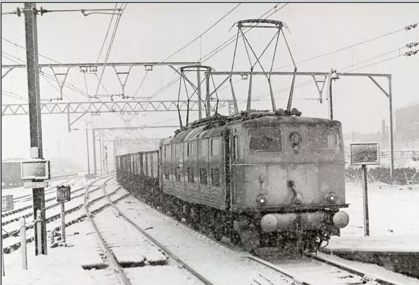
Below: With a short vacuum fitted coal train behind, No. 76003 approaches Penistone station from the Sheffield direction in a heavy snow storm during the morning of 31 January 1980. This loco was built as No. 26036 and was renumbered as 76036 in January 1974. It was further renumbered to 76003 on 22 October 1976 when like brake fitted locos were numerically grouped together. CJM
