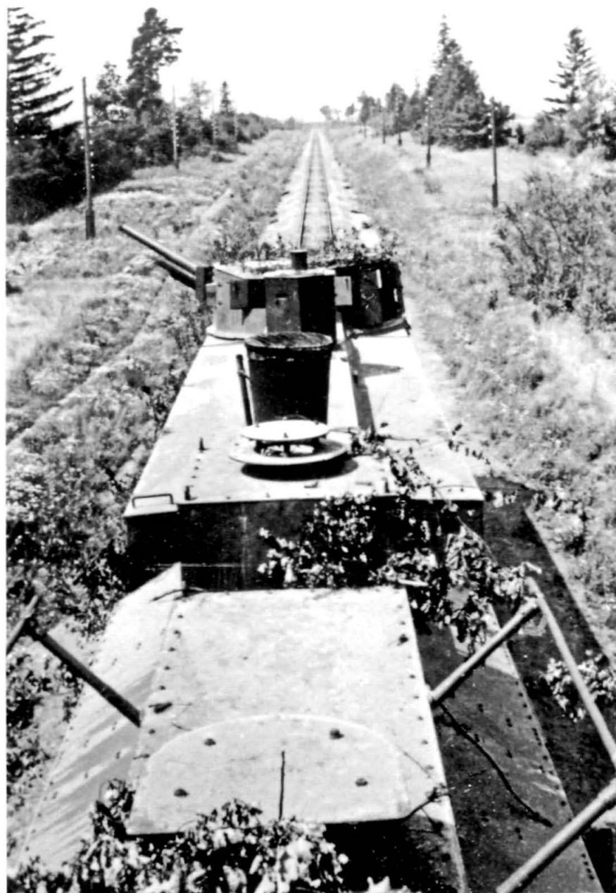
Many Soviet armored trains were lost in the 1941 summer battles. This is a heavy armored train with the photo taken from the command car, the radio aerials evident in the foreground. The heavy artillery car in front is a Military Depot 60 type built in 1931–32 with the characteristic single turret. (NARA)
