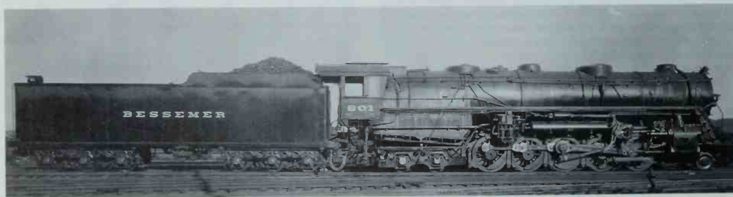
B&LE's 47 2-10-4s were copies of Burlington's 2-10-4s and were put to the same use — hauling heavy trains of minerals. B&LE photo.
