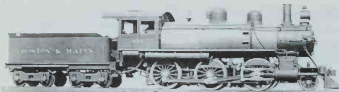
Boston & Maine Moguls 662 (later 1389) and 1366 were built by Alco's Manchester Works in 1903. Number 662 illustrates the appearance as built; No. 1366 was photographed in 1945 and shows the difference four decades can make: cross-compound air pump, steel cab, centered headlight, piston-valve conversion steam chests, and cast tender trucks. The large turbogenerator is for train lighting; the cluster of cables at the top of the smokebox is for lighting the train when the engine is running in reverse. Photo of 1366 by Homer Newlon.
