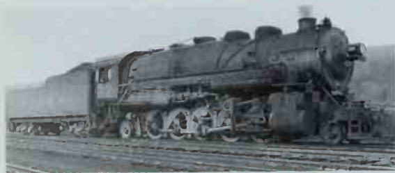
New York, Ontario & Western 356, built by Alco in 1915, followed the design of the first 2-10-2s in having its firebox over the rear two pairs of 57" drivers. Canadian Government Railways, Boston & Maine, and New Haven rostered similar Santa Fe types. Photo by A. V. Neusser.
