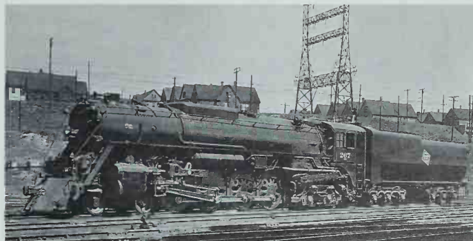
Because of wartime restrictions on new designs, the S3s combined elements of 4-8-4s Alco had recently built for Rock Island and Delaware & Hudson — and the result was a good looking engine. Milwaukee Road photo.
