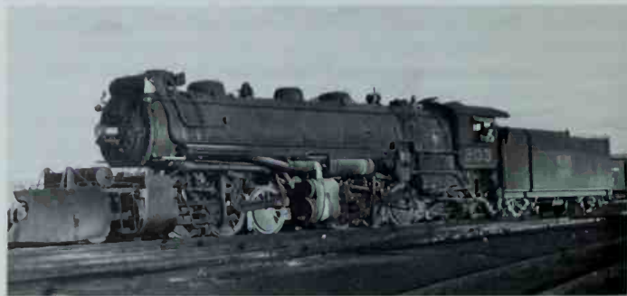
WP's 2-6-6-2s were somewhat lighter than the USRA 2-6-6-2 but had larger cylinders and could exert the same tractive effort. After 1931 they were assigned to the Keddie-Bieber line, where the snowplow pilot was a necessity in the winter. Photo by Philip C. Johnson.
