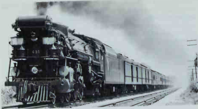
C&O had the first Mountain type and the heaviest Hudson, but the F-19 Pacific epitomizes Chesapeake & Ohio passenger power. Number 491 displays the C&O "flying pumps" face, with (top to bottom) Elesco feedwater heater, bell, paired cross-compound air pumps, low-mounted headlight, and slatted pilot. Photo by Lucius Beebe.
