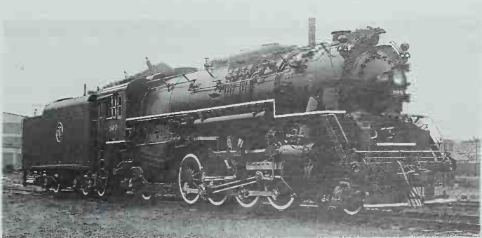
DT&I's Mikados are one of the few examples of a road reverting to a smaller locomotive after purchasing large ones. The 800s looked like the Berkshires, but most had short 8-wheel tenders. Lima photo, collection of P. E. Percy.
