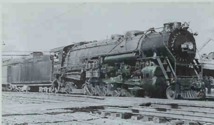
The USRA heavy Mountain was the basis for FEC's last group of 4-8-2s, 801-823, built in 1926. Number 803 carries two cross-compound air pumps on her right side, balancing a feedwater heater pump out of sight on the left side. Photo by James G. LaVake.
