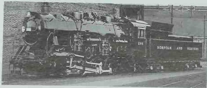
After years of using outmoded road engines for switching, N&W went for the 0-8-0 whole hog with 30 purchased from Chesapeake & Ohio in 1950 and 45 of its own manufacture between 1951 and 1953. Engine 244 was the last reciprocating steam engine built for service on an American common carrier railroad. N&W photo.
