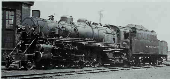
K-6B Pacific 2094 is a 1924 product of Alco's Brooks Works. The inward-sloping cab sides are a Lehigh Valley characteristic. The built-up coal bunker let the engine run from Jersey City to Buffalo with a single stop for coal at Towanda, Pennsylvania. Photo by Donald W. Furler.
