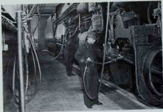
N&W's Lubritorium featured drop hoses like those in an automobile service station that made lubricating locomotives faster and easier. N&W photo.
