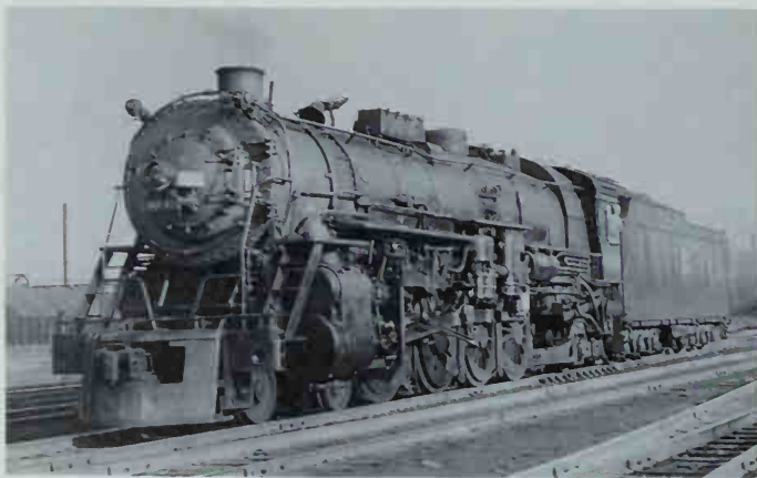
Mountain type 4045, a 1923 Brooks product, was rebuilt about 1940 with lightweight rods, roller bearings on all axles, and large tender, and was converted to a coal burner. Photo by John W. Malven.
