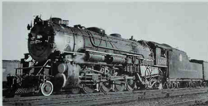
The relatively low drivers (63") and main rod connected to the third drivers indicate that Rio Grande 1509 was designed primarily as a freight locomotive. Photo by Wesley Krambeck.
