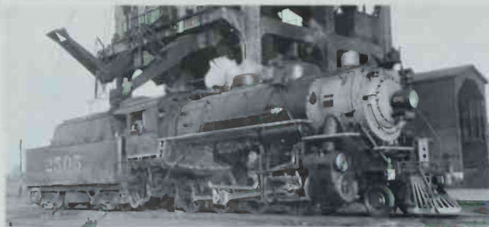
Southern's heaviest 2-8-0s were the ten members of the Ks-3 class, built by Alco's Richmond Works in 1926 for service in the coal-mining area north of Knoxville, Tennessee. Photo by Walter H. Thrall, Jr.
