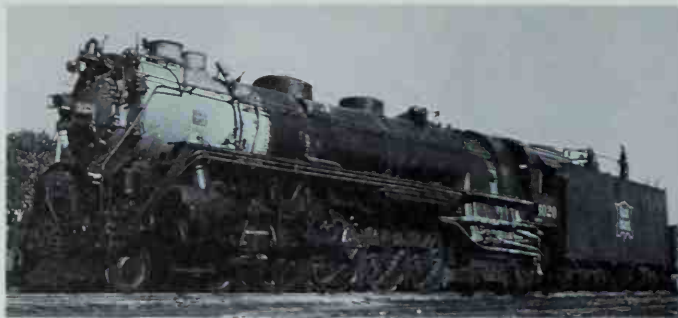
No railroad in the U. S. had more 4-8-4s on its roster than Rock Island. Number 5020, shown taking on fuel oil at Enid, Oklahoma, in 1948, was built by Alco in 1929. Rebuilding in the late 1930s included 74" drivers, disk main drivers, and increased tender capacity. Photo by Sid Davies, collection of Charles E. Winters.
