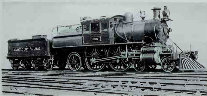
Atlantic City Railroad 1027 is a Vauclain compound built by Baldwin in 1896. The high-pressure and low-pressure cylinder on each side drive on a common crosshead. The piston valve for both cylinders is just inboard of the high-pressure cylinders. Baldwin photo; Collection of H. L. Broadbelt.
