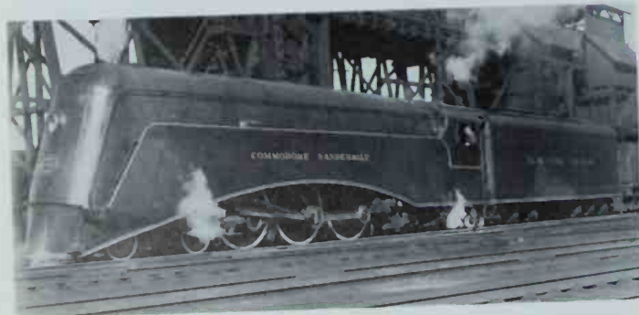
New York Central Hudson No. 5344 was streamlined in 1934 and given the name Commodore Vanderbilt . In 1939 it was reshrouded to match the 10 J-3a Hudsons delivered the previous year. Photo by Glenn Grabill Jr.
