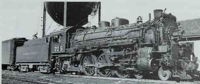
Pacific 715 illustrates trademarks of T&P power after the 1920s: shielded air pumps on the pilot and Elesco feedwater heater with a diamond-shaped T&P herald on its front. Photo by Charles M. Mizell, Jr.; collection of Harold K. Vollrath.
