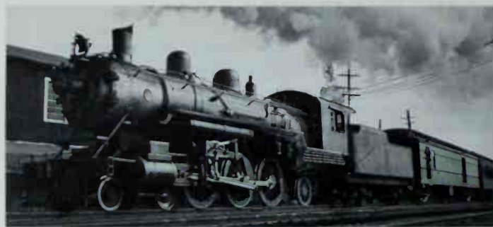
Southern's 4-6-2s weren't all Ps-4s. P-1 No. 1292, built by Baldwin in 1906, was built with 63" drivers for service in the mountains. Its slide valves are driven by Southern valve gear. Collection of Bruce R. Meyer
