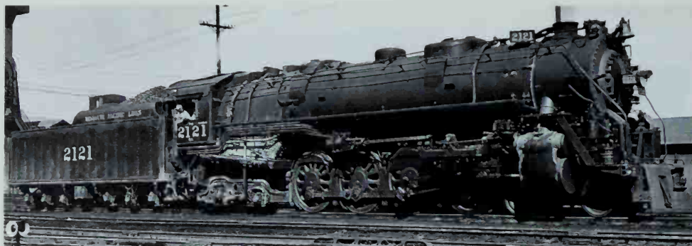
MoPac's shops at Sedalia, Missouri, took in the 2-8-4s and rebuilt them into 4-8-4s. They had twin sand domes like the 2-8-4s. Photo by Gordon B. Mott.
