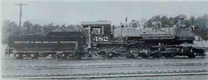
This side view of K-36 No. 482 clearly shows the details of the outside frame. The drivers are between the frames, but the counterweights and crankpins are outside. D&RGW photo.
