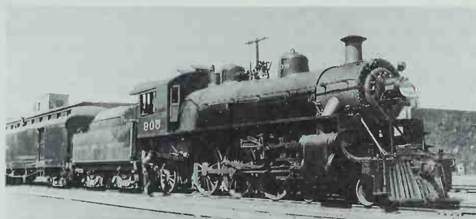
Light Pacific 905 has a slightly British look, with its capped stack, curved running board step, and lack of external plumbing. It was built by Brooks in 1903 as a 2-6-2, rebuilt to a Pacific in 1911, and given its British styling in 1924. Photo by C. W. Jernstrom.
