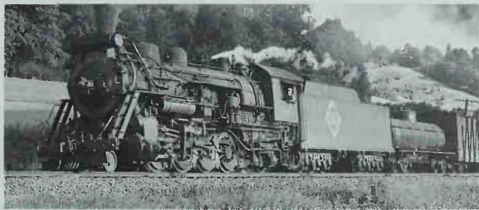
Mikado 3005, built by Baldwin in 1911, leads a way freight west near Alfred, N. Y., in 1950. Modifications to the 2-8-2 since construction include Elesco feedwater heater, disk main drivers, and a large 12-wheel tender. Photo by R. G. Nugent.
