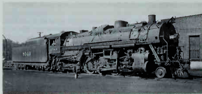
Rebuilding altered the appearance of IC's 2-8-4s; removing the Elesco feed-water heater made most of the difference. IC 8049 appears in its original form on page 284 as Lima 1.
