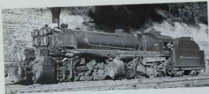
Z-3 Mallet 4025, pictured at Wallace, Idaho, in June 1952, was one of the middle group of 2-8-8-2s. The 40"-diameter cylinders of the low-pressure engine signify great tractive effort and little speed. The small tender implies frequent water stops. Photo by Don Roberts, collection of H. M. Griffiths.
