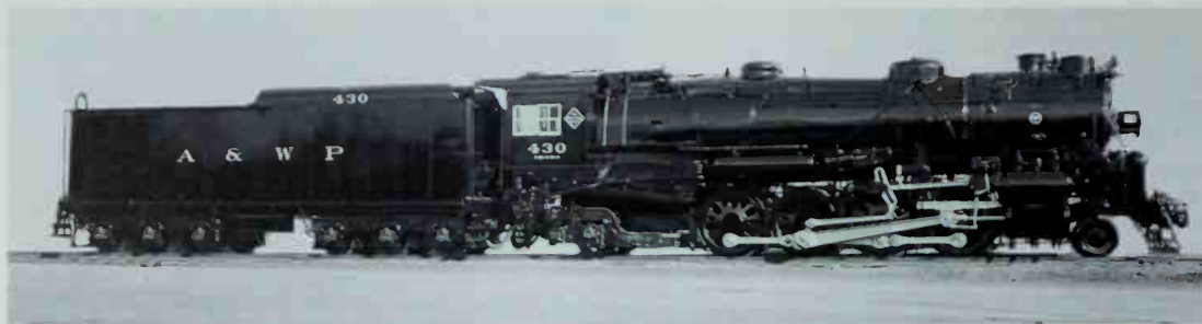
A&WP 430 and identical twin Western Railway of Alabama 380, built by Baldwin in 1944, were thoroughly modern copies of the USRA heavy Mikado of 1918. Among the improvements are dual air pumps mounted on the pilot, Elesco coil-type feedwater heater, Boxpok drivers, cast trailing truck, and a large 12-wheel tender. BLW photo.
