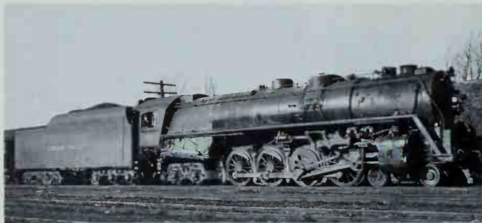
Wyoming type 5103 was built by Baldwin in 1932. The odd rear tender truck originally carried a booster. Photo by Ray Ollis Jr.
