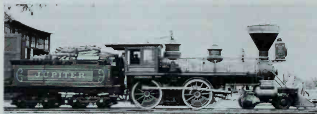
Virginia & Truckee 12, painted and lettered to represent Central Pacific Jupiter at the Chicago Railroad Fair of 1949, is a typical 1870-era 4-4-0, except for the air pump ahead of the cab. Collection of Frederick E. Braun.
