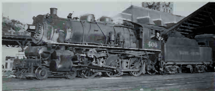
Maine Central's O-3 Ten-Wheelers were chunky locomotives, easily identified by the air reservoir on the pilot. Number 406 is ready to leave Portland on train 59 to Rockland in July 1945. Photo by Peter Ascher.
