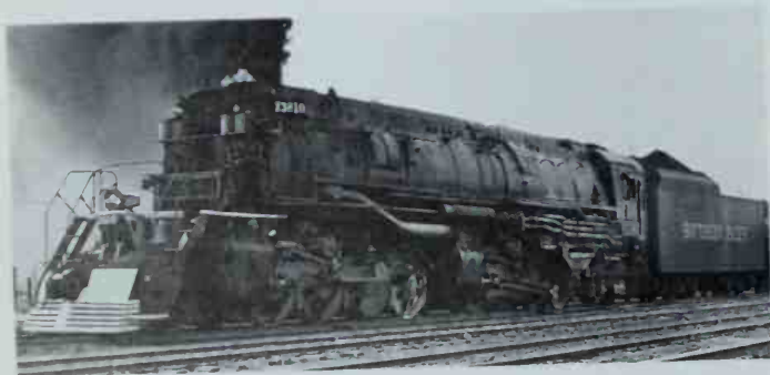
The Lima-built AC-9s were SP's only coal-burning articulateds of conventional layout. The skyline casing over the domes wasn't quite enough to qualify them as streamlined. Photo by R. H. Kindig.
