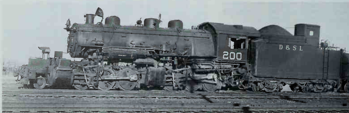
In the 39 years between 1908, when it was built, and 1947, when it was photographed, Mallet 200 acquired a lead truck, disk main drivers, built-up coal bunker sides, and a brakeman's cab on the tender. Photo by Richard H. Kindig.
