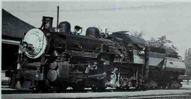
Southern Pacific 3000 was rebuilt in 1927 by the road's Sacramento shops from an earlier A-3 class Atlantic. Improvements included a Worthington BL feedwater heater and a booster-equipped cast trailing truck. In 1946 No. 3000 was dolled up with red and orange paint on its cab and tender to pull the Sacramento Daylight , a Sacramento-Lathrop, California, connection to the San Joaquin Daylight . Photo by Fred Matthews.
