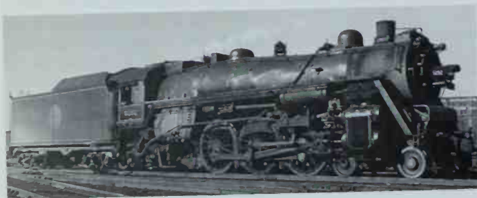
Alton 5292 (formerly Chicago & Alton 652) has lost its extended smokebox and gained a shielded air pump above the pilot, a smaller cab, and a larger tender, but the taper of the boiler remains. Photo by Bruce Meyer.
