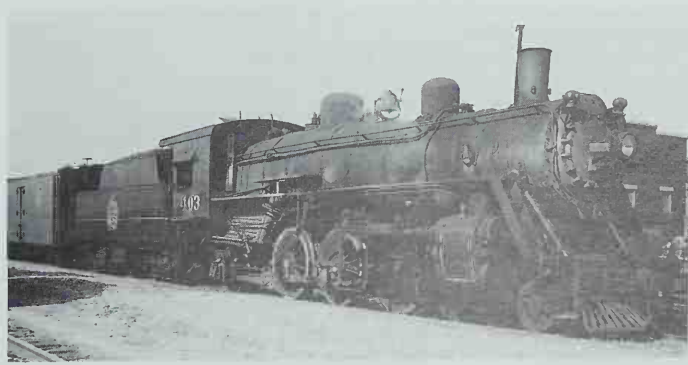
Pacific 403 is a P-2, built in 1913 with 64" drivers for freight service. The odd-shaped cab is typical of ACL's early Pacifics. Photo by George W. Pettengill.
