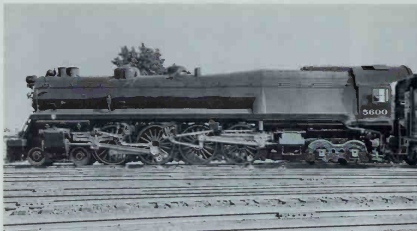
George H. Emerson's final watertube-firebox experiment was No. 5600, a duplex-drive 4-4-4-4. The location of the rear cylinders made them vulnerable to dirt and cinders. Add them to the humped firebox, an air reservoir tucked in above the forward cylinders, a double stack, and backward valve gear and you have an engine that is not quite Picasso-esque but seems to have too many parts in the wrong places. B&O photo.
