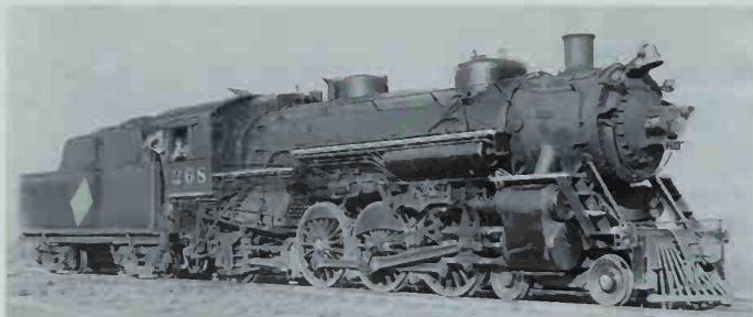
In the 1920's Mobile & Ohio bought ten 4-6-2s that were copies of the USRA light Pacific. The principal point of difference between the USRA locomotive and M&O's Pacifics was the cab roof: the USRA cab roof had a deeper curve. Photo by John B. Allen.
