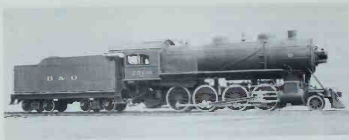
Baltimore & Ohio 2500 was the first of the E-27 class, which ultimately numbered 414 locomotives. Note that the firebox is over the rear pair of drivers. Collection of C. W. Witbeck.
