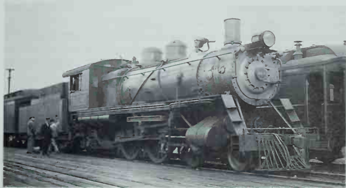
SP&S's Atlantics were duplicates of Great Northern's, balanced compounds with inside high-pressure cylinders driving the first axle and outside low-pressure cylinders driving the second axle. Their rebuilding to simple locomotives and the addition of booster-equipped cast trailing trucks duplicated GN's modifications. SP&S removed the boosters in 1931, a year before this photo was taken. Photo by R. V. Nixon.
