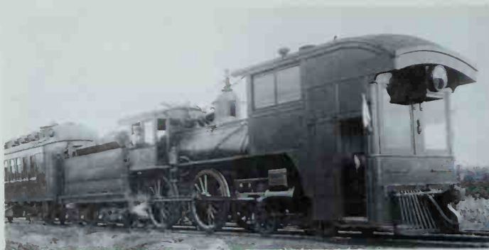
In the Teens the Burlington rebuilt and modernized many old 4-4-0s for light duties, creating the A-2 class. A few A-2s became inspection engines, like No. 360. Photo by C. H. Osgood; collection of L. E. Griffith.
