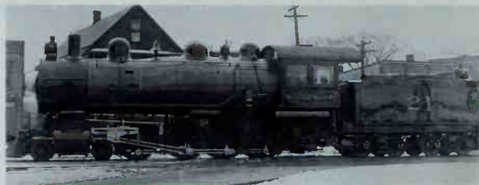
paint, plus white trim on the tires and running boards, and the glass removed from the cab windows. The second and third drivers are blind — and so close together that there is no room for a flange on either. Right side, C. W. Witbeck collection; left side, Alco History Center.
