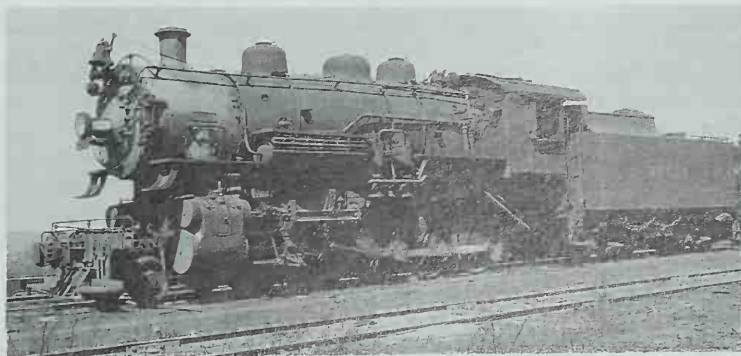
Twelve-Wheeler 205 was built by Brooks in 1899. Its inboard valves and narrow Belpaire firebox are typical of Brooks locomotives of the time. It was renumbered 225 in 1911 and rebuilt in 1926 with outboard piston valves, Walschaerts valve gear, a wide radial-stay firebox above the drivers, and an extended smokebox. 205, Alco Historic Photos; 225, collection of Harold K. Vollrath.
