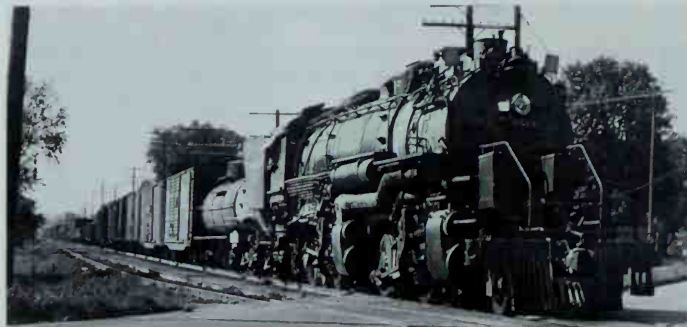
Cylinders the same size fore and aft are evidence that 2-8-8-0 No. 757, shown leading a freight north out of Neosho, Missouri, has been converted to a single-expansion engine. Photo by William K. Barham.
