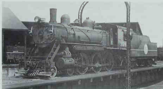
Ten-Wheeler 359, at Lakeland, Florida, in 1946, is representative of ACL's Copper Heads, even though the ornamental copper flange on the stack is long gone. When it was superheated it was equipped with Modern steam chests. Photo by George W. Pettengill.
