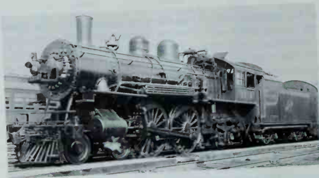
Chicago & North Western 1314 was a member of the first group of Atlantics built with a wide bituminous-burning firebox behind the drivers. Collection of John S. Kamacher.
