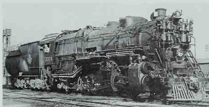
The 69" drivers of GN's O-8 class Mikados put them in the same league with the 2-8-4s of Erie and Nickel Plate. Photo by H. W. Pontin.
