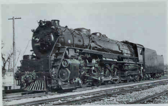
Northern 3008, photographed in 1929, illustrates the H class as delivered, with spoked drivers and banjo frame at the rear. Photo by A. W. Johnson.
