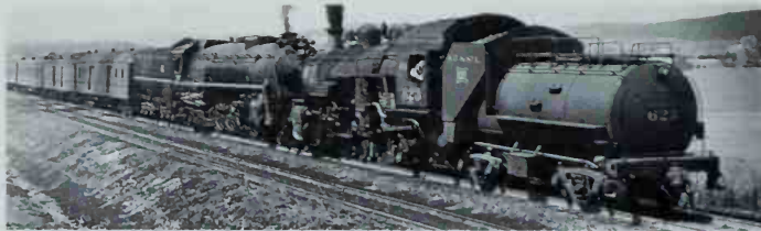
The Mikes put in time in Cumberland Mountain helper service. Passenger train helpers were coupled ahead of the road engine, in this case a J3 4-8-4, and were as likely to run backward as forward. Photo by Hugh M. Cromer.
