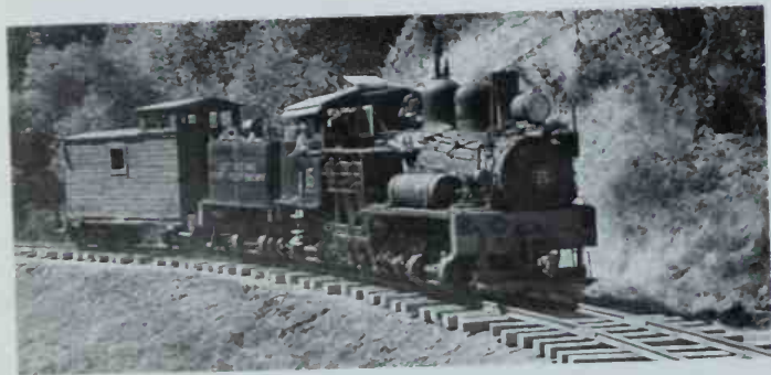
Shay No. 15 of the West Side & Cherry Valley, a tourist-carrying successor to the West Side Lumber Company, displays the basic elements of a Shay: three slide-valve cylinders, longitudinal driveshaft, bevel gears driving each axle, and boiler off-center to balance the cylinders. Photo by Robert L. Hogan.
