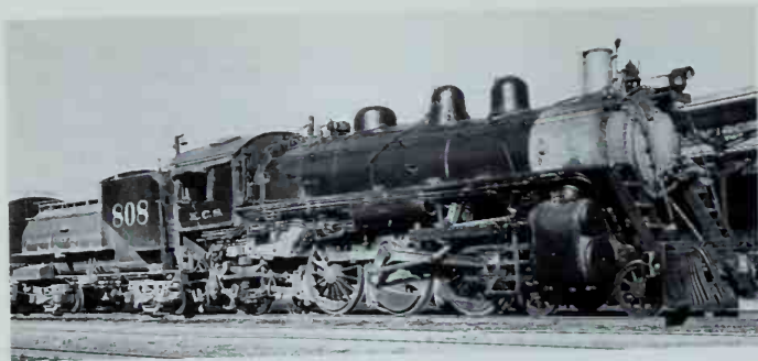
Pacifics like No. 808 (built by Schenectady in 1919) were KCS's most modern passenger power. The second sand dome is unusual on a passenger engine. Photo by Charles E. Winters.
