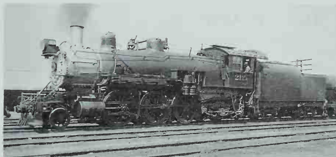
The CB&Q was a major user of the Prairie type, with 429 of them on its roster. Number 2121, shown at Congress Park, Illinois, in 1939, is an R-5, built in 1907. The inboard piston valves and squared counterweights were already out of date when the locomotive was built. The low tender with curved coal bunker sides and the "mantel-clock" headlight are Burlington trademarks. Photo by J. W. Saunders.
