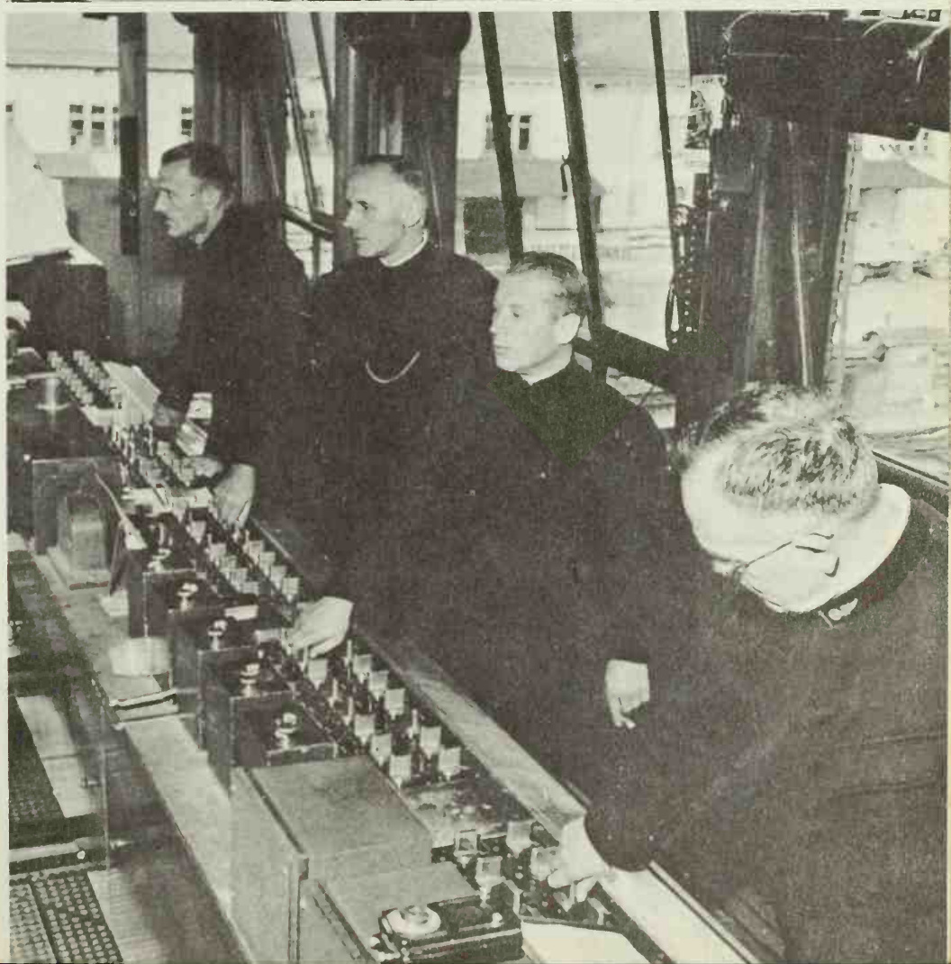
The all-electric interlocking panels of the Zurich signal box interlocking frame. Note the uniforms the signalmen wear. The author spent some time in this box.
