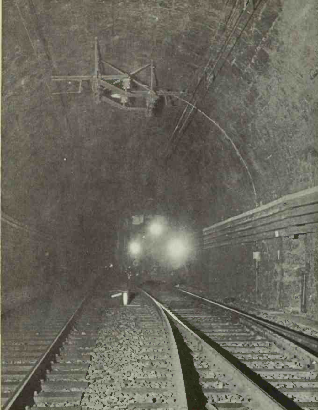
Passenger trains approaching Gotthard crossover in the middle of the Gotthard Tunnel, which is controlled from Göschenen. Note the fireman looking out on the "right side"—also the fine drainage, excellent ballast, and steel ties.
