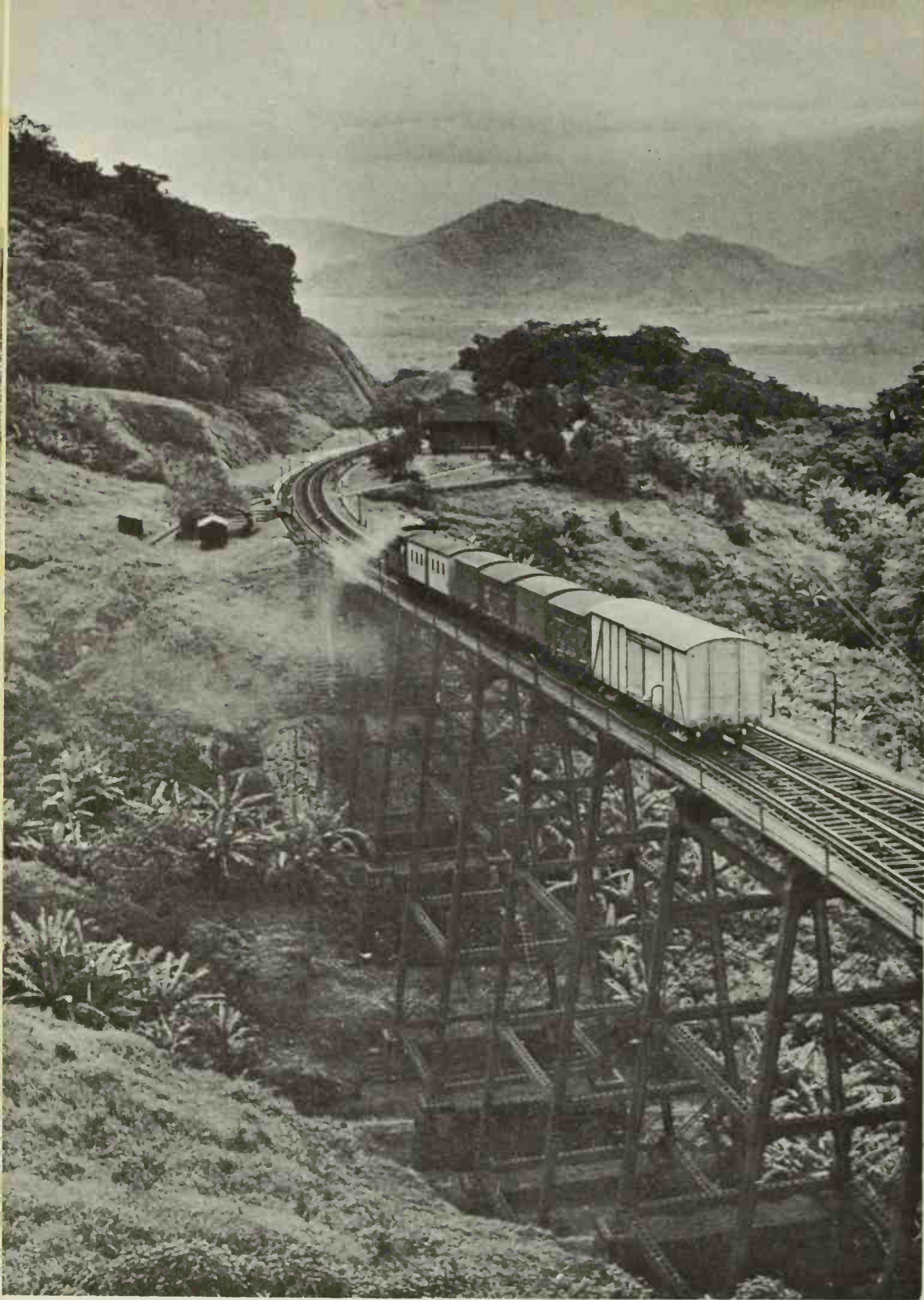
Freight train approaching siding near the bottom of the Serra incline. Santos Plain is in the background. The engine is practically nothing more than a brake and the tonnage is usually pushed up, with the engine on the head end descending, the cable, of course, doing the real work.
