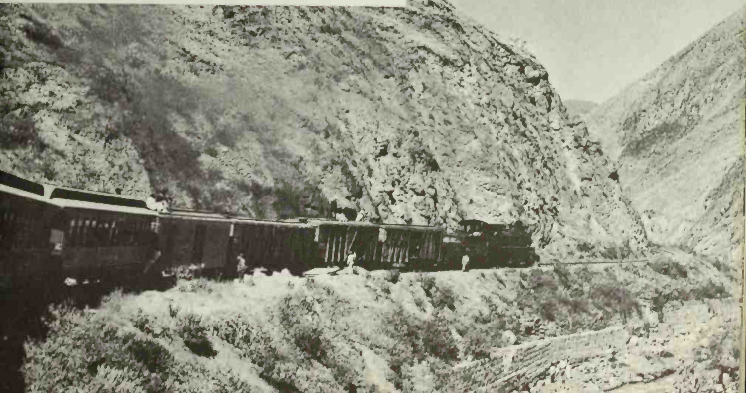
Typical mixed or second-class train on the Guayaquil and Quito Railway leaving the narrows of the Devil's Nose. Maximum curvature is 29 degrees. The standard rail is 55 to 70 pounds per yard.
